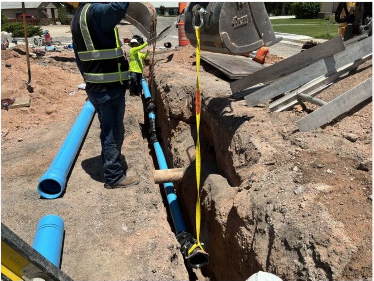
Placing DI 45 bends under existing water on Malachite Ave. sta. 42+00-42+13
