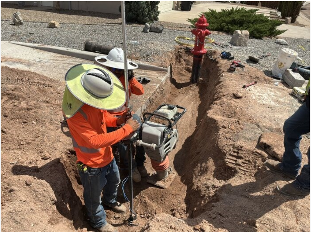
Survey as-built shot on GV for Hydrant #26
