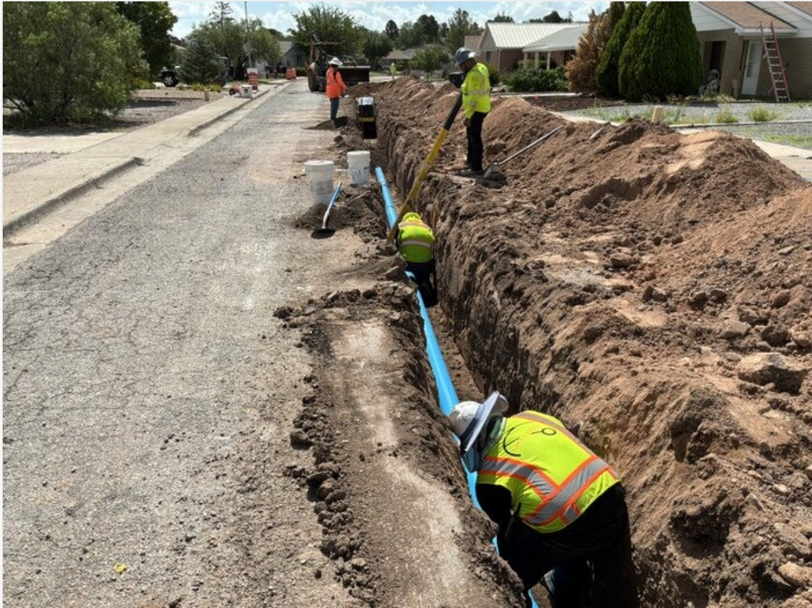
Placing 6" C-900 on Chalcopyrite Ave.
