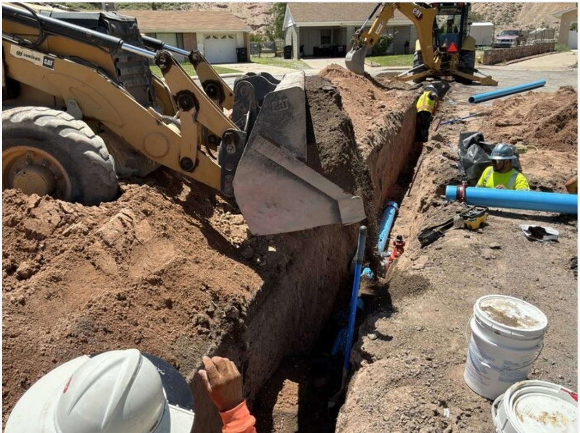
Placing processed bedding over 6"C-900
