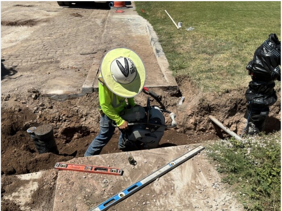
Compaction on backfill of fire hydrant on Copper Ave. and Chalcopyrite Ave.
