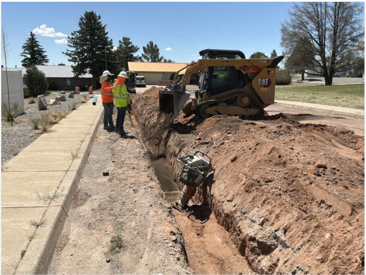
Placing backfill over 6" C-900 on Chalcopyrite Ave.
