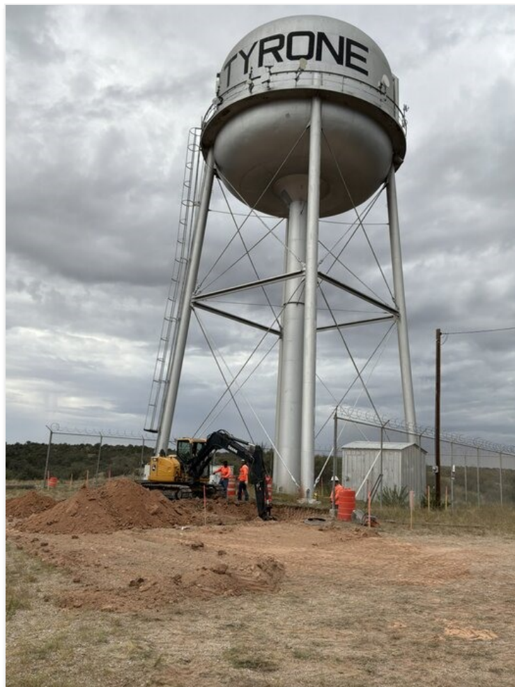
Excavation for the valve vault pit.
