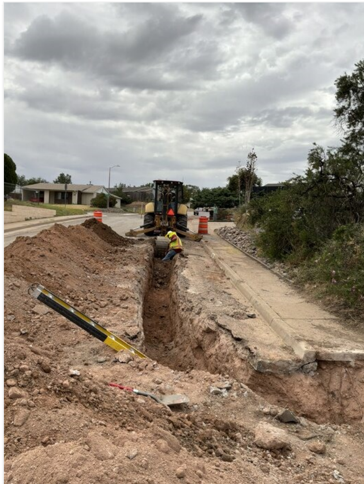
Excavating for 6" C-900 placement on Malachite Ave.
