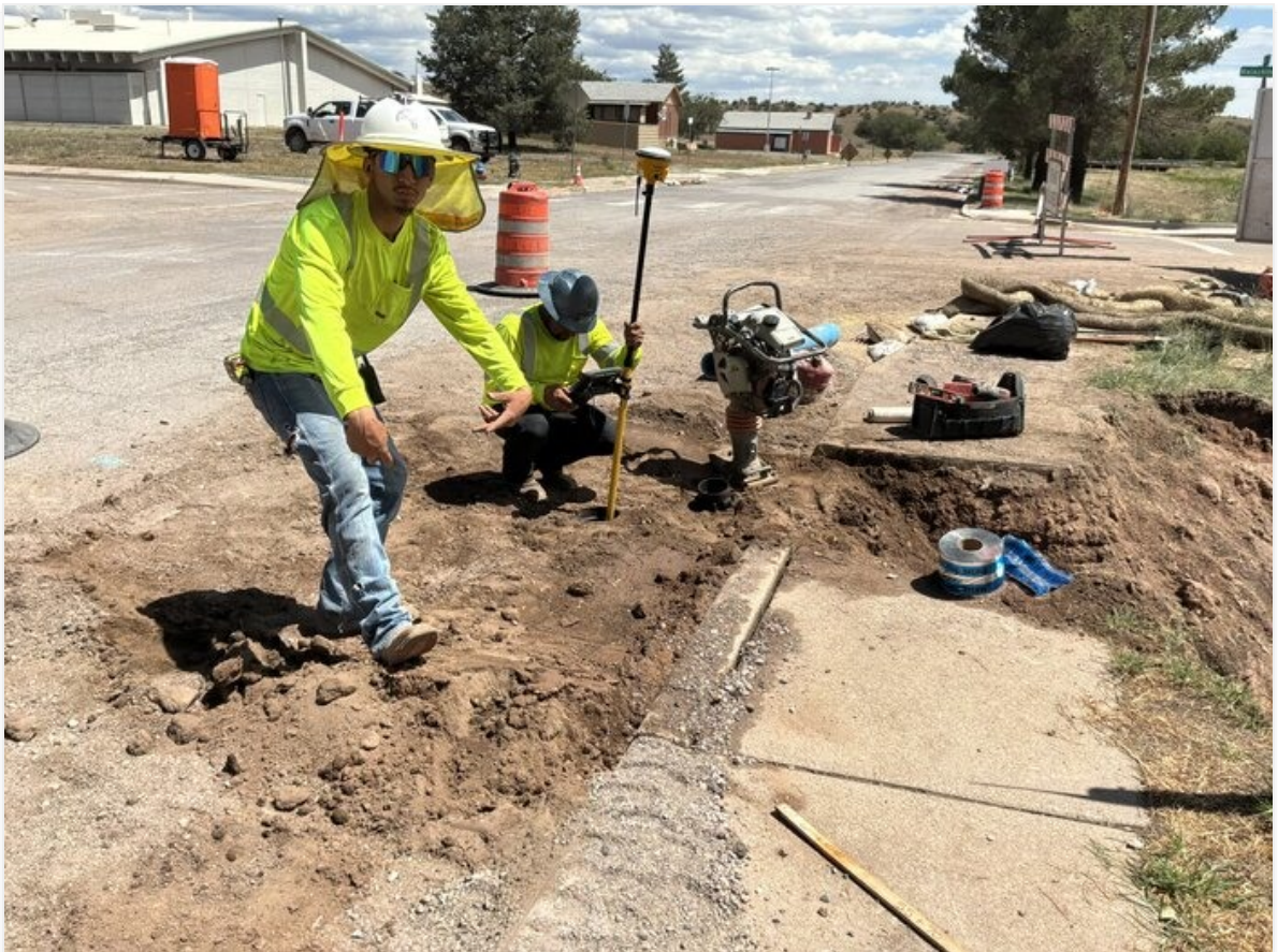
Survey as-built shot on DI fittings.
