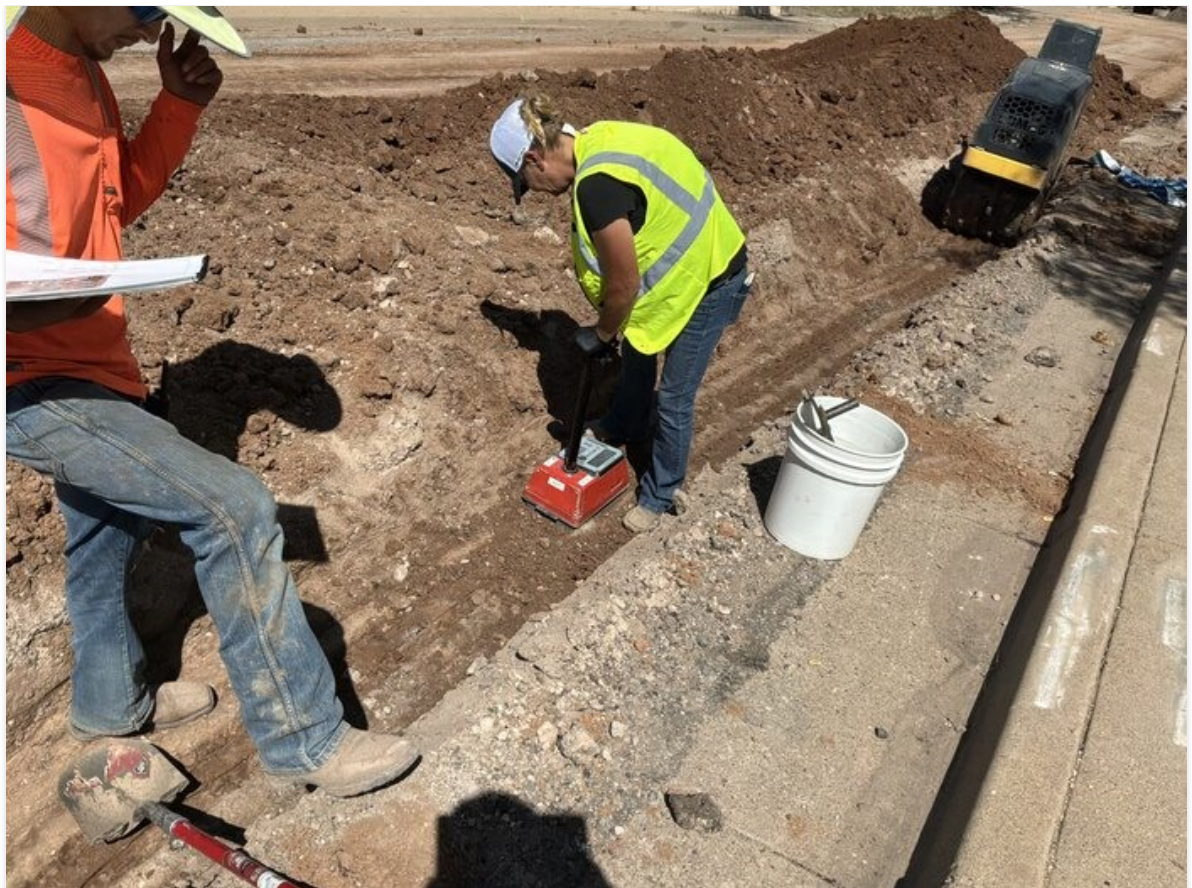
Summit Testing taking backfill densities.
