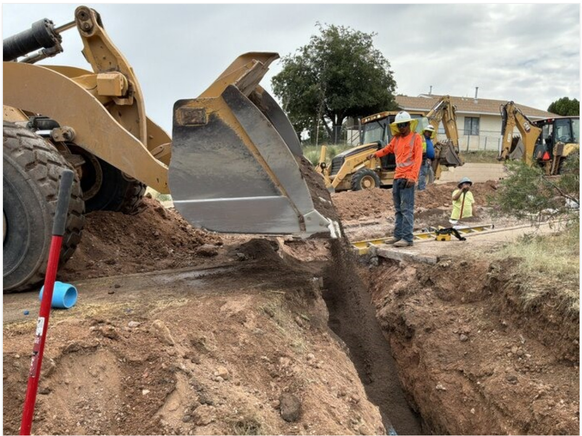
Pipe bedding being placed into trench.
