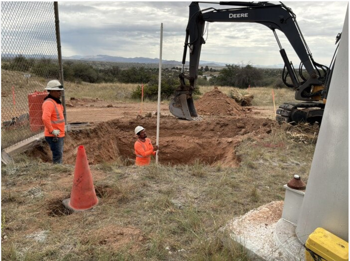
Checking depth for the valve vault pit at the tank site.
