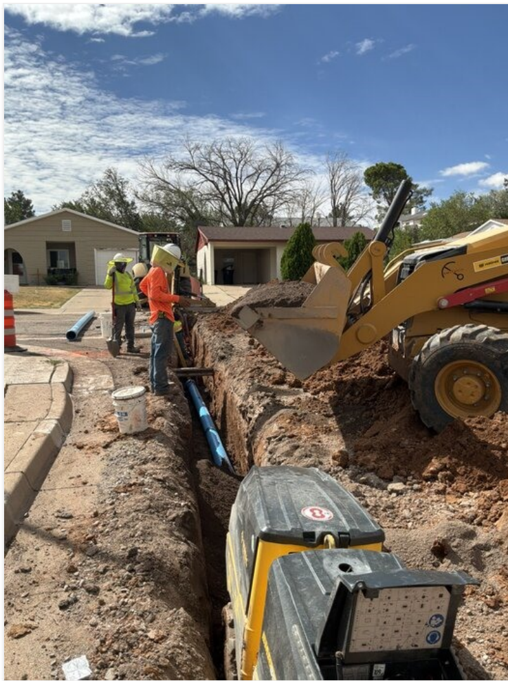
Placing backfill over 6" C-900 on Chrysocolla Ave.
