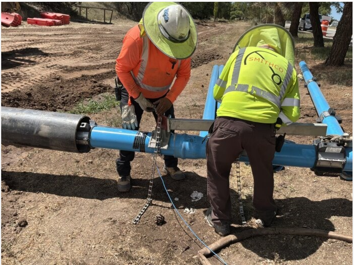
Pushing 6" C-900 together with tool.
