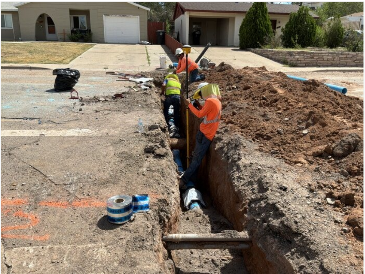
Survey as-build shot being taken on DI fittings on Chrysocola Ave.
