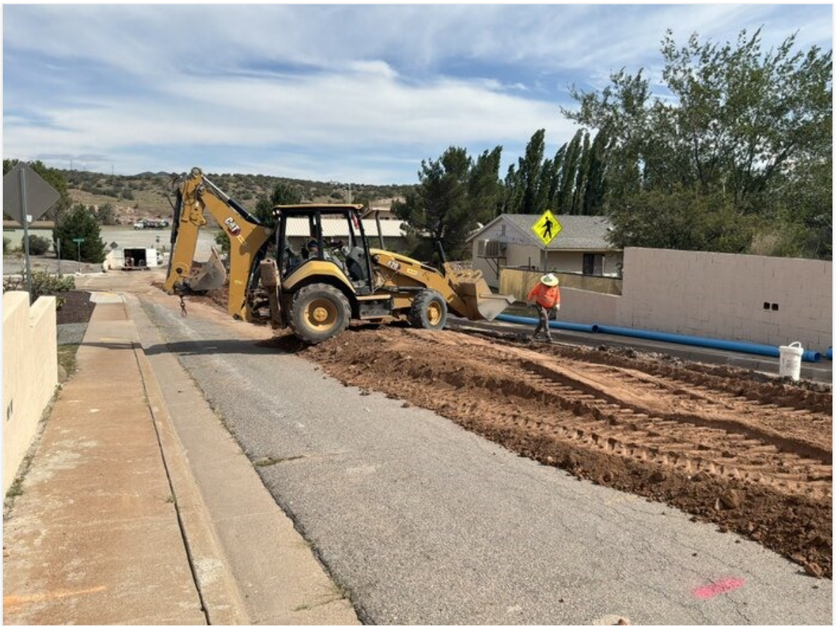
Backfill process on Chrysocolla Ave.
