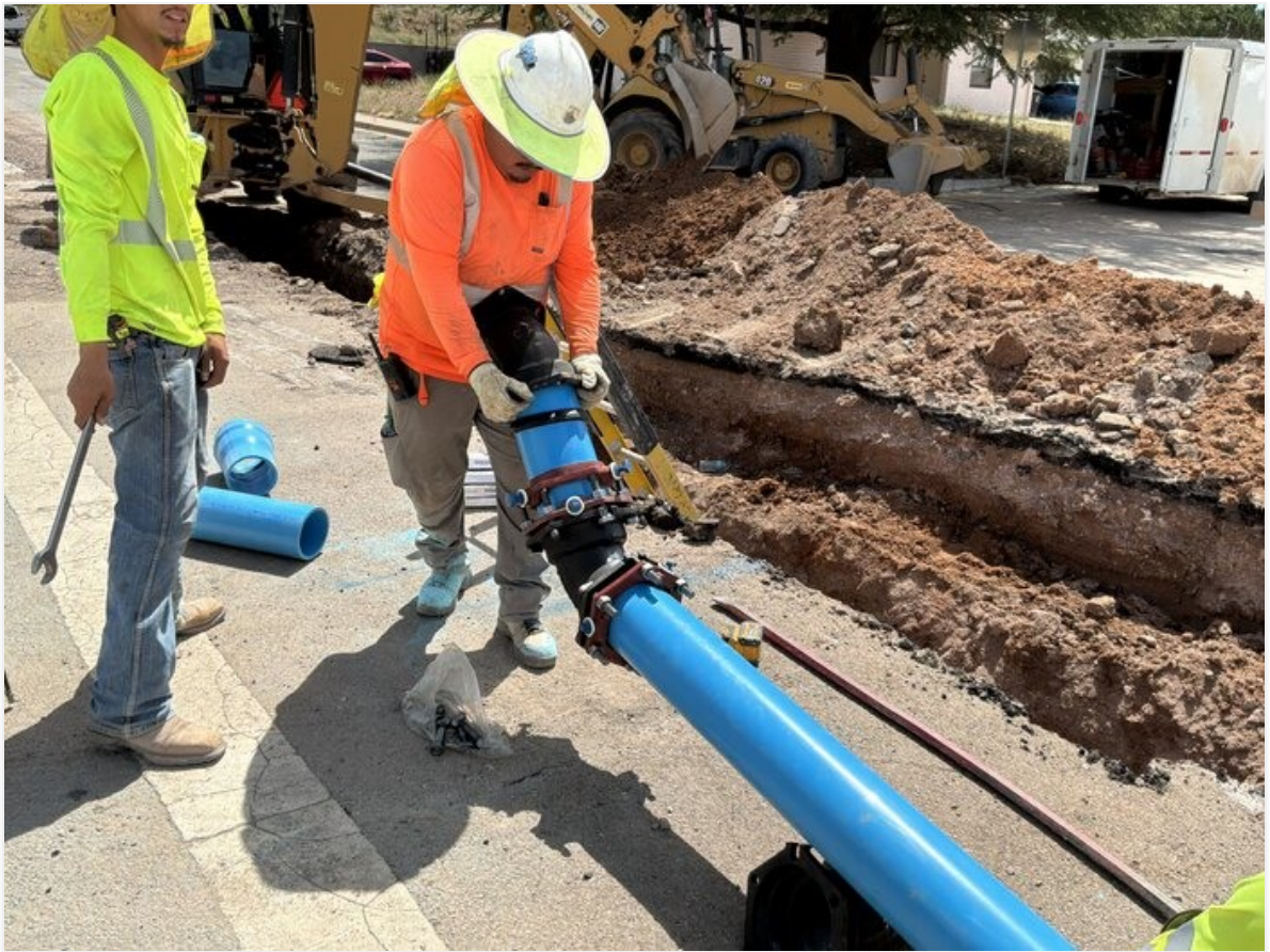
Connecting DI 45 outside of trench.
