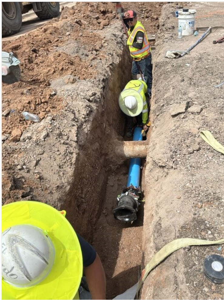
Going under existing water line Chrysocola Ave.
