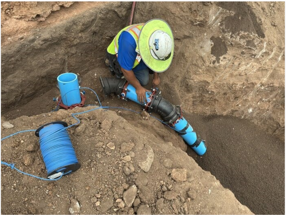
45 DI fittings coming out of the arroyo next to Malachite aAve.
