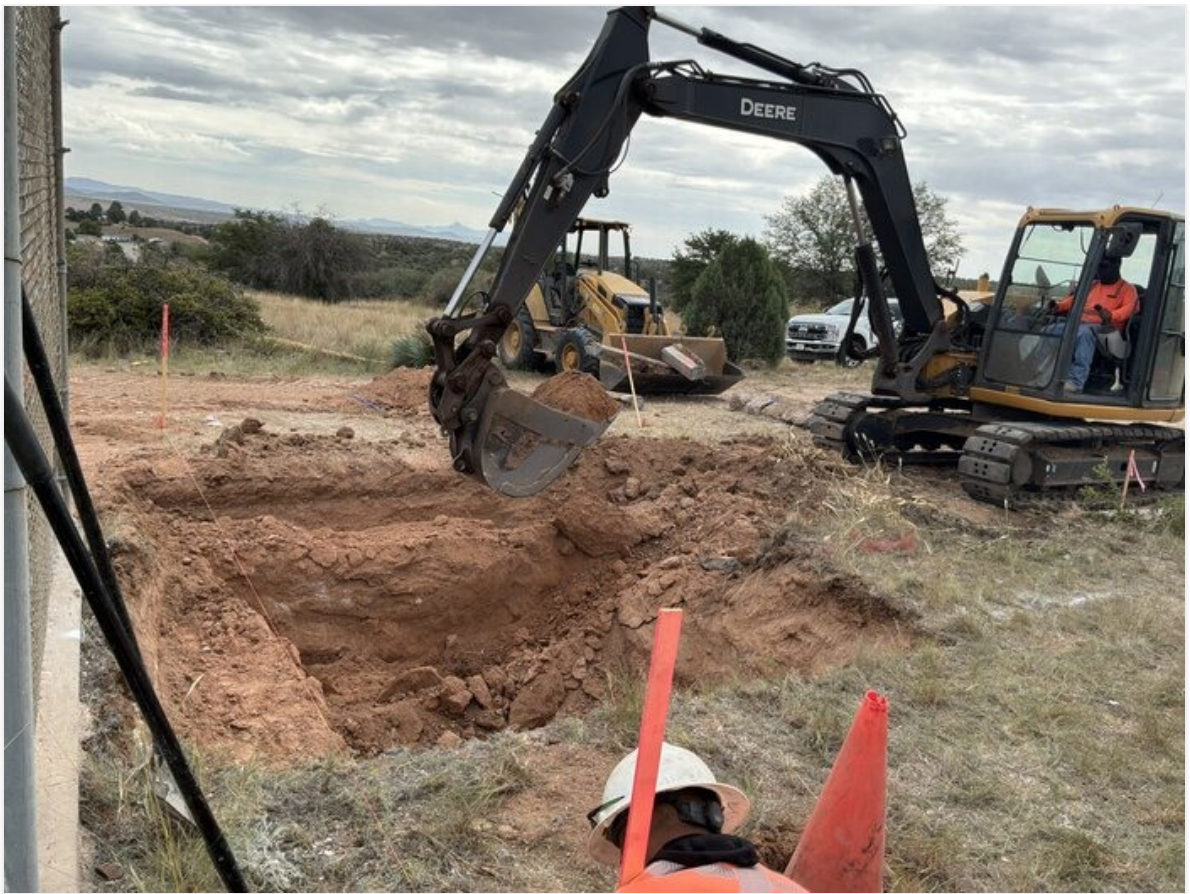
Excavation for the valve vault pit.
