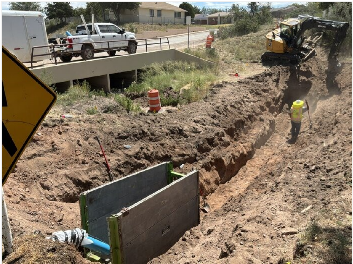
Excavation for 12" steel casing with trench box.
