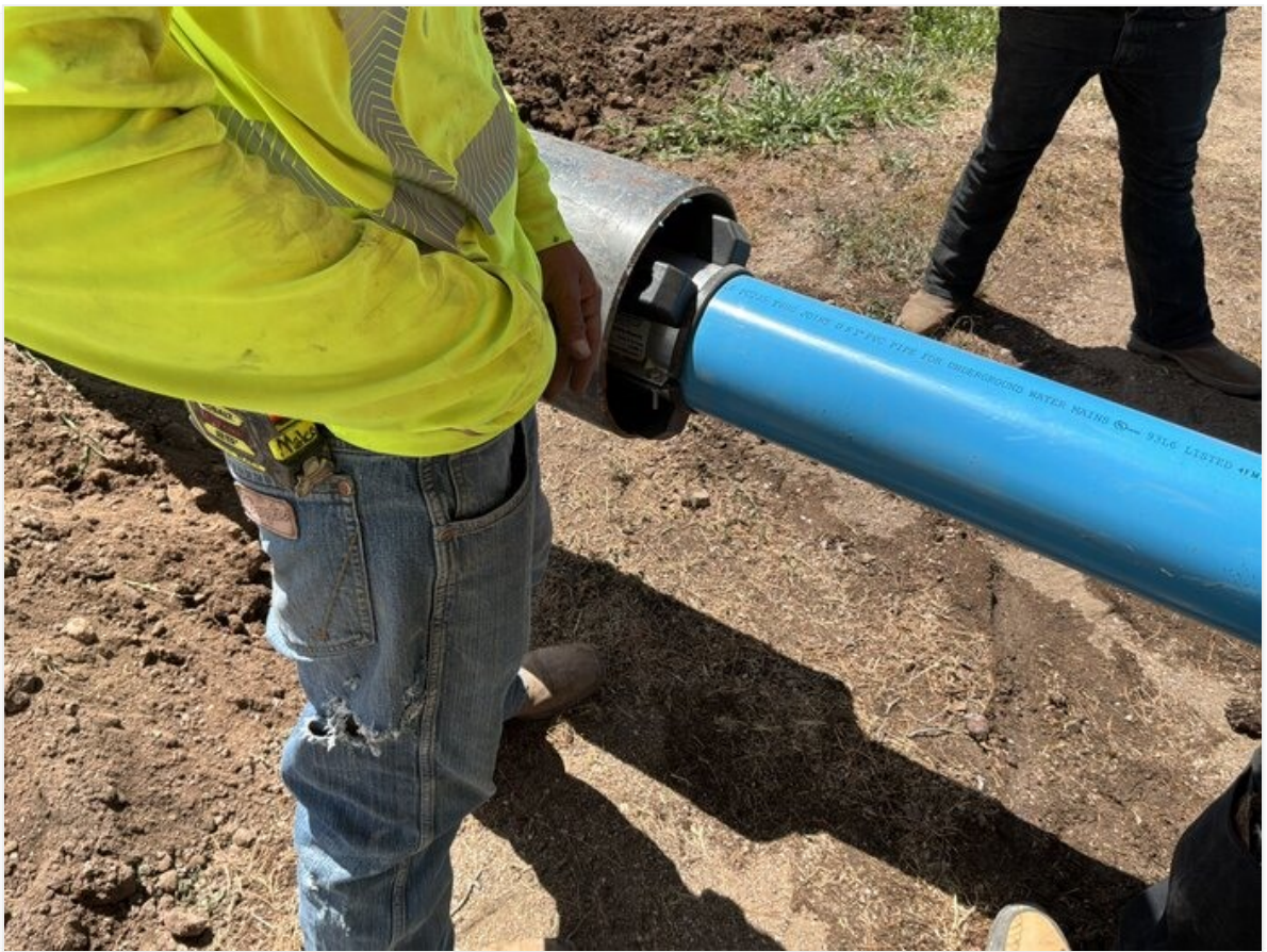
6" C-900 being pushed into 12" steel casing.
