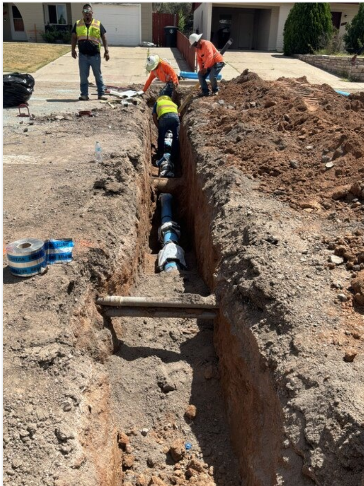
Di 45 fittings wrapped with anti corrosion plastic, under the existing water line on Chrysocola Ave.
