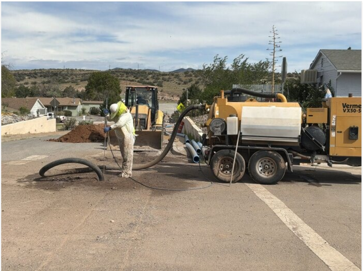
Potholing for existing utilities on Chrysocolla Ave.
