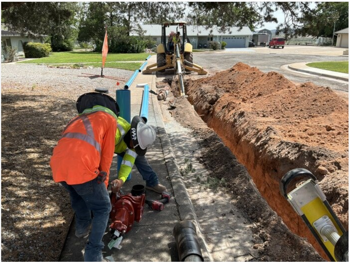
Placing megalugs on gate valve for Tenorite Ct.
