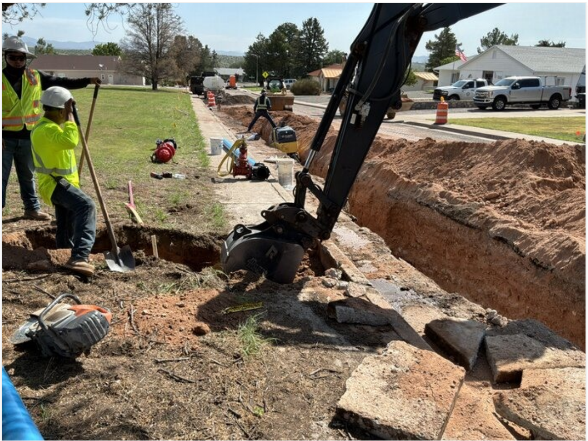
Removing curb and gutter for hydrant placement on Malachite Ave. sta. 39+34
