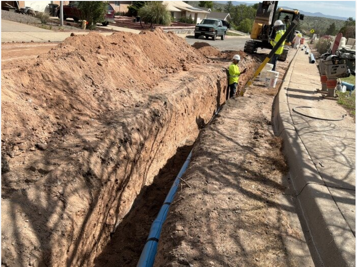
6" C-900 placement operations on Malachite Ave.
