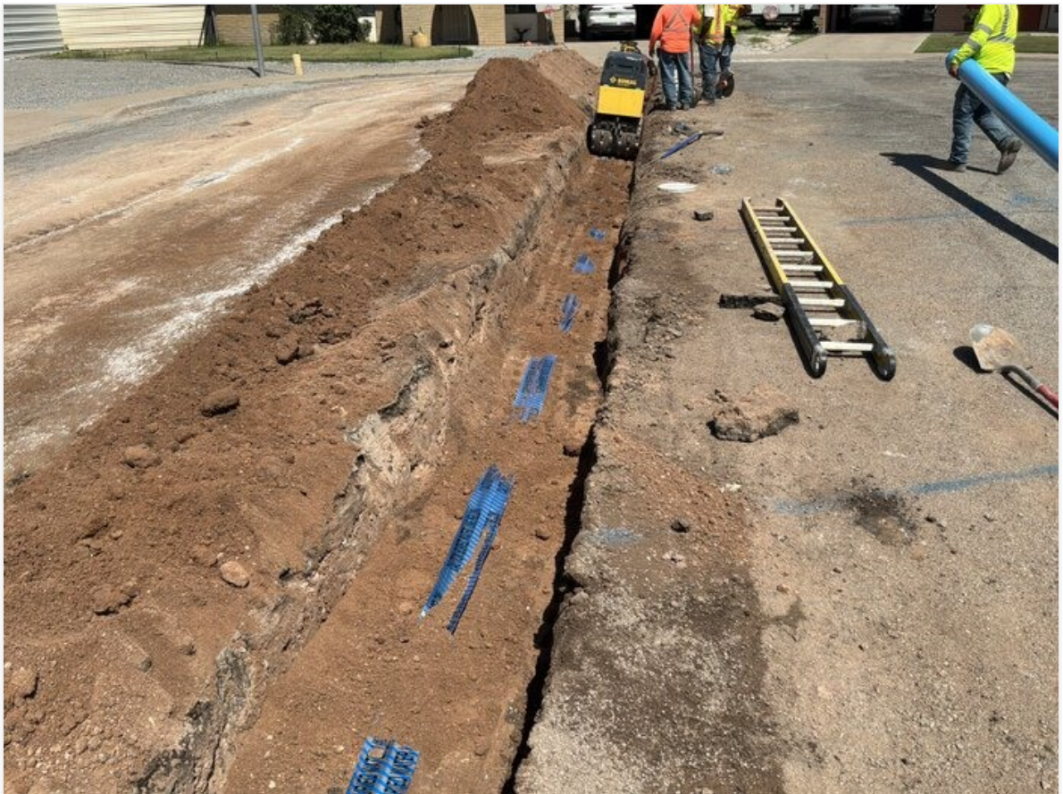
Caution tape in trench on Copper Ct north.
