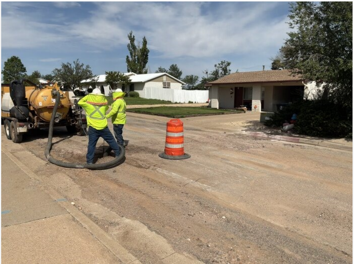
Potholing for gate valve on cuprite St.
