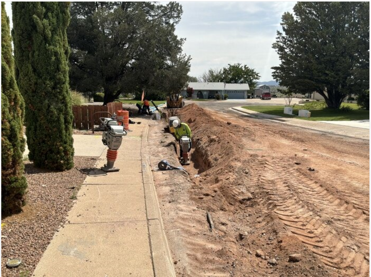
Compaction over 6" C-900 on Tenorite Ct.
