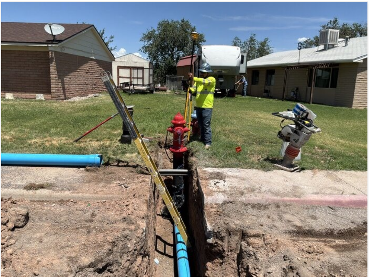
Survey as-build shot being taken on new hydrant on Cuprite St.
