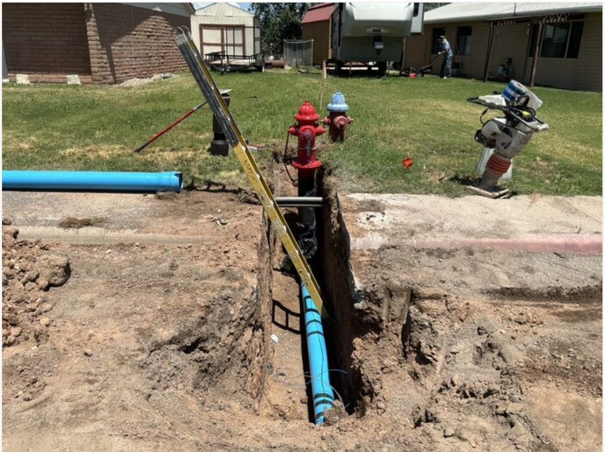
New hydrant placed on Cuprite St.
