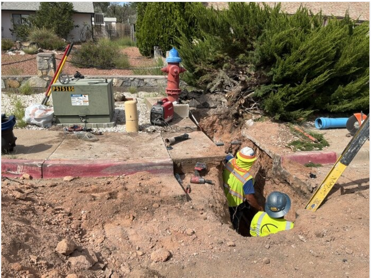
New hydrant placement on Cuprite St.
