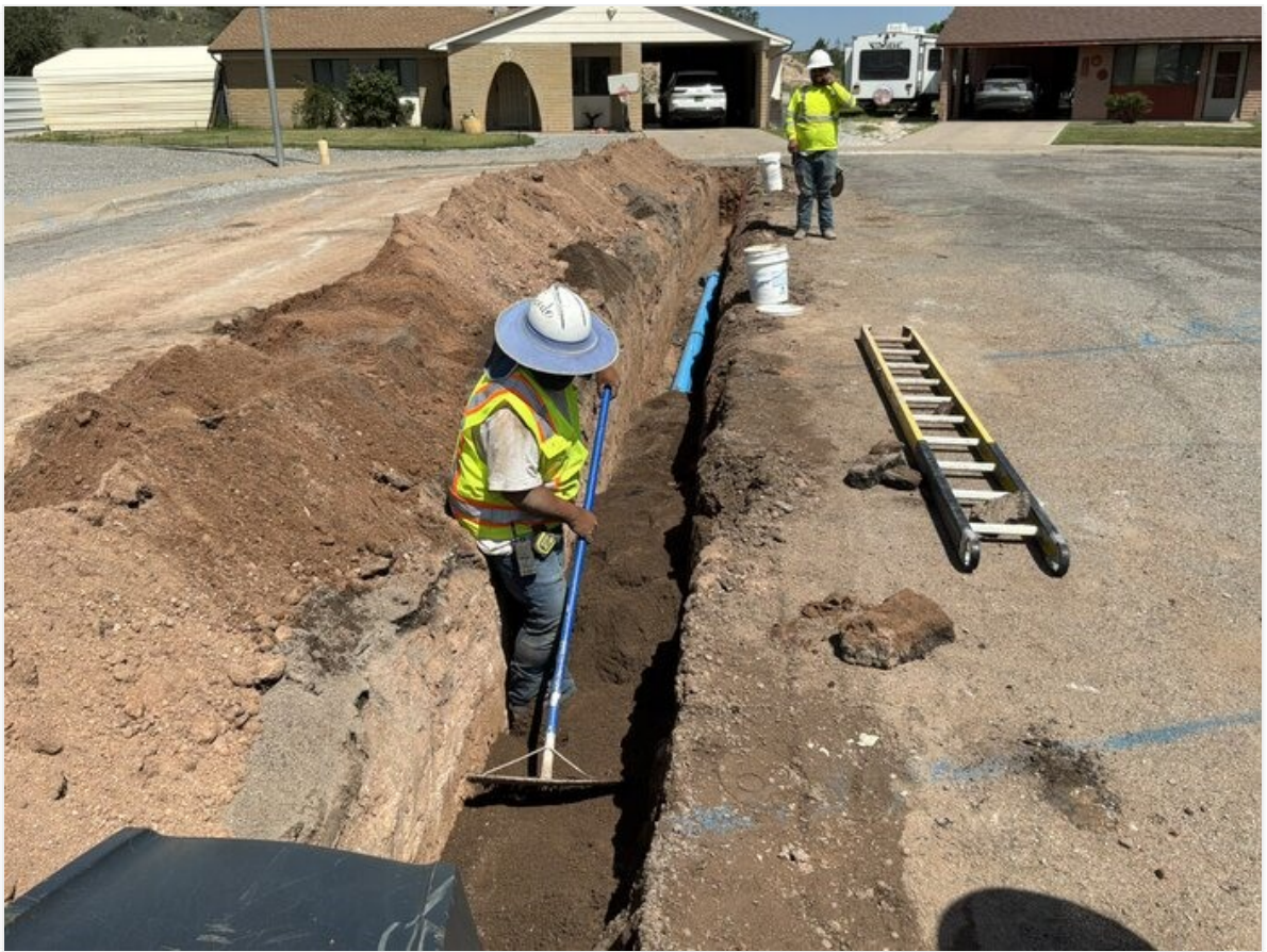
Pipe bedding on Copper Ct north.
