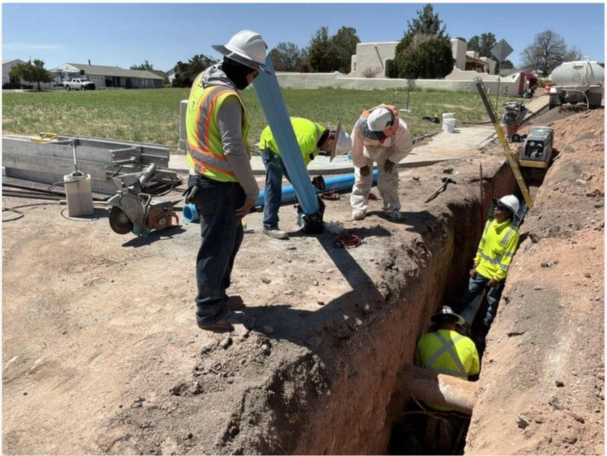
45 DI bends being assembled to go under existing water on Malachite Ave.
