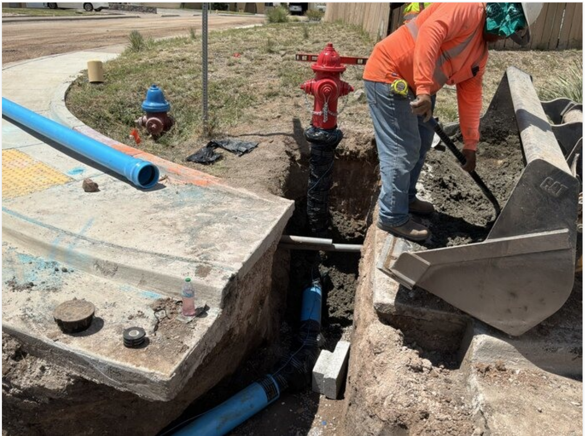
Concrete thrust block being placed for hydrant #13. (Sta 35+33)
