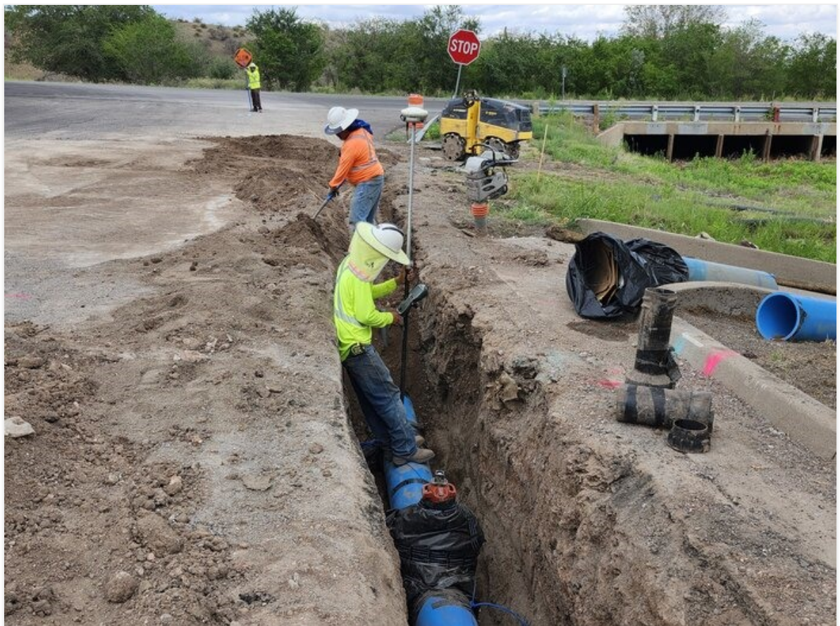
Survey as-built on replaced fittings for tie-in on Copper Dr. as per RFI #14
