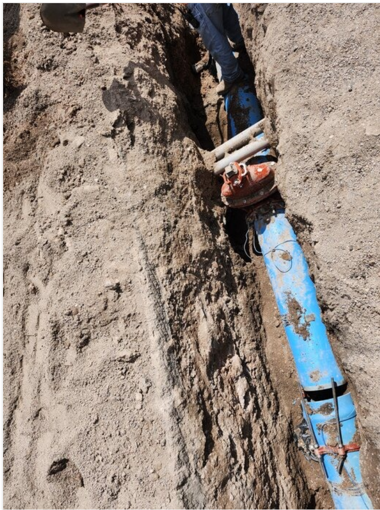
Removing installed GV, 2" saddle and cap as per RFI #14 on Copper Dr. tie-in.
