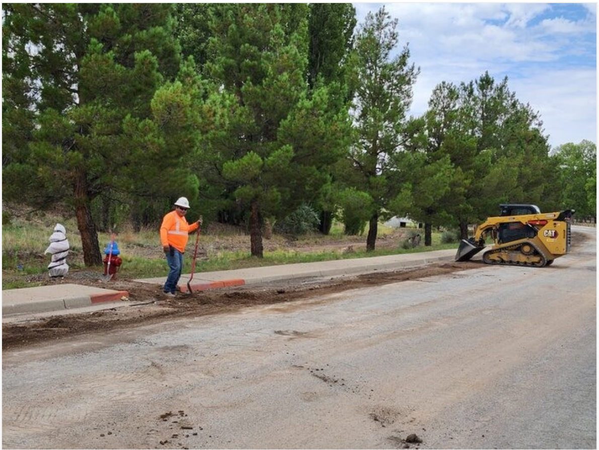
Contractor maintaining shoulder damage caused by rains.
