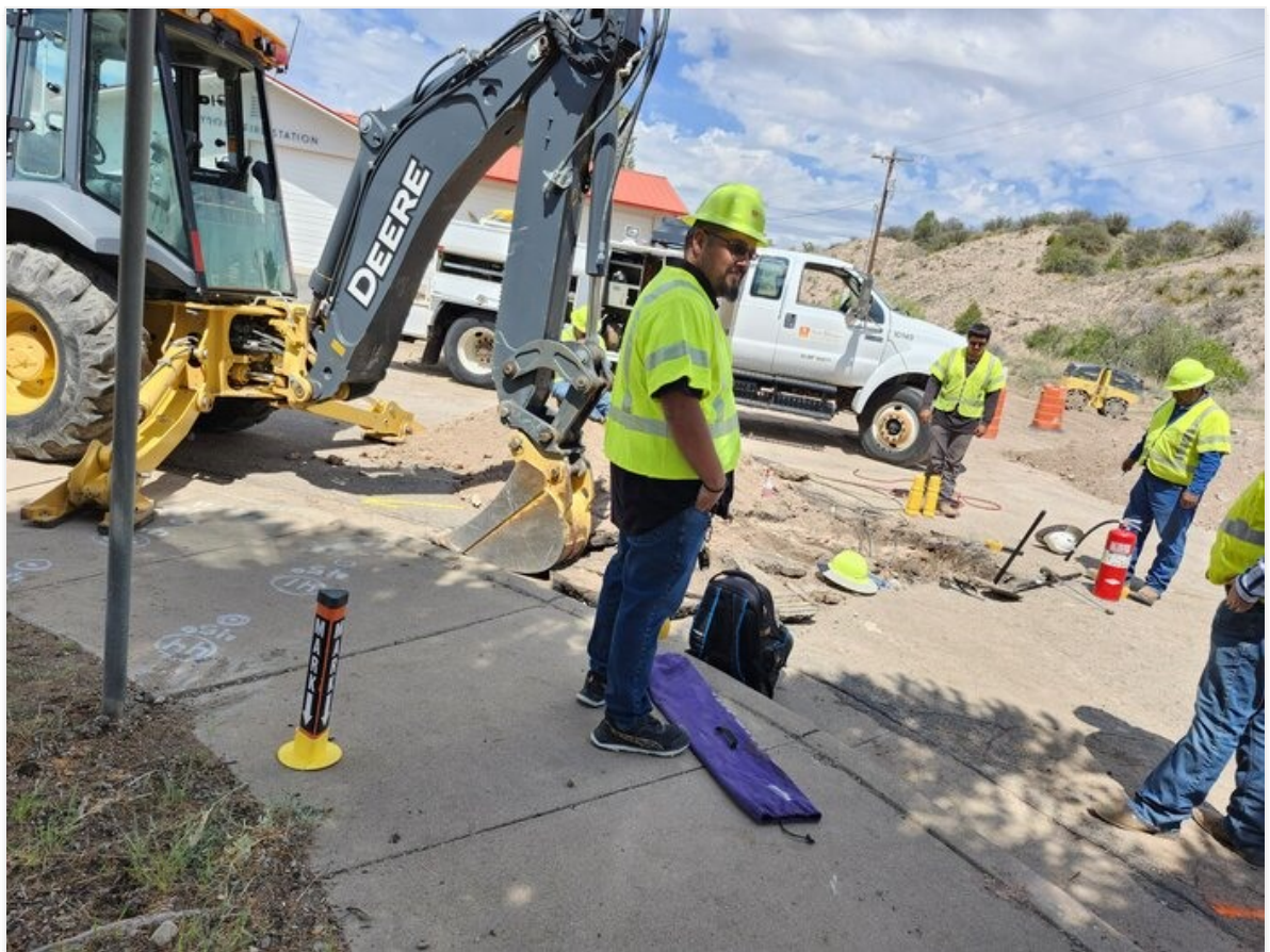
NM Gas making 2" gas repair on Malachite Ave.
