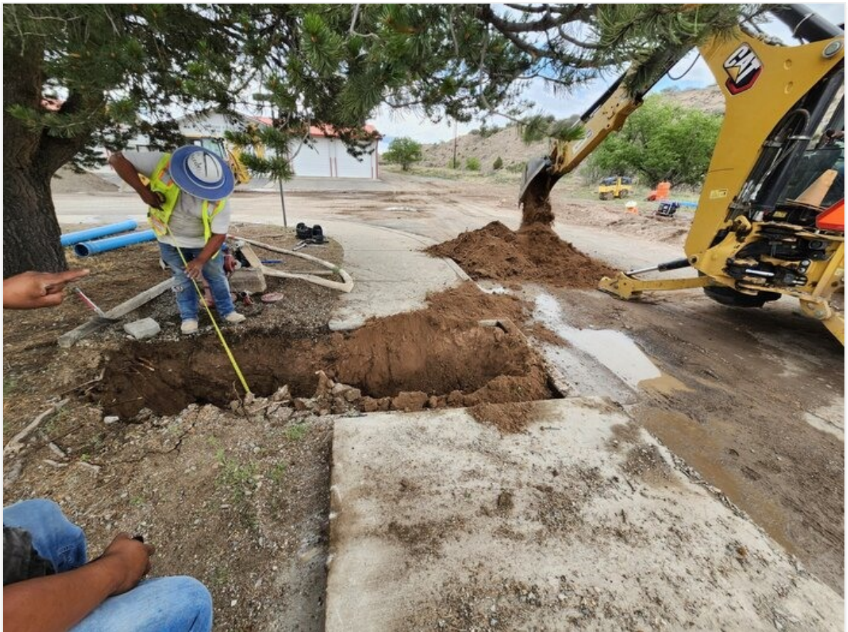
Hydrant #1 excavation on Turquoise Dr.
