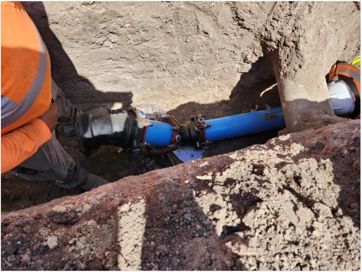
DI 45 bends under existing water line on Malachite Ave.
