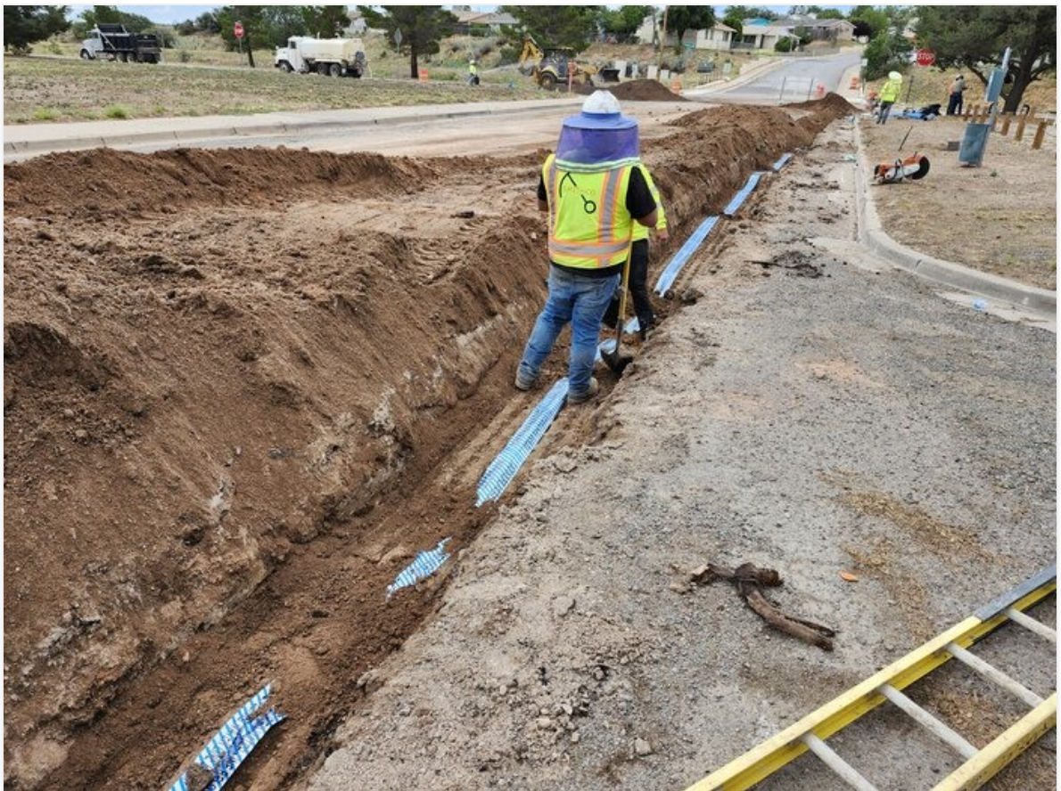
Caution tape being placed over 6" C-900 on Malachite Ave.
