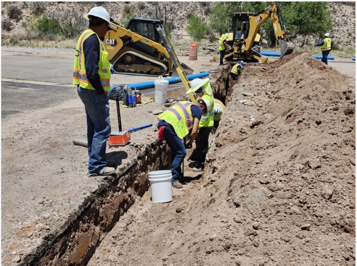
Summit Testing taking densities on backfill over 6" C-900 on Malachite Ave.
