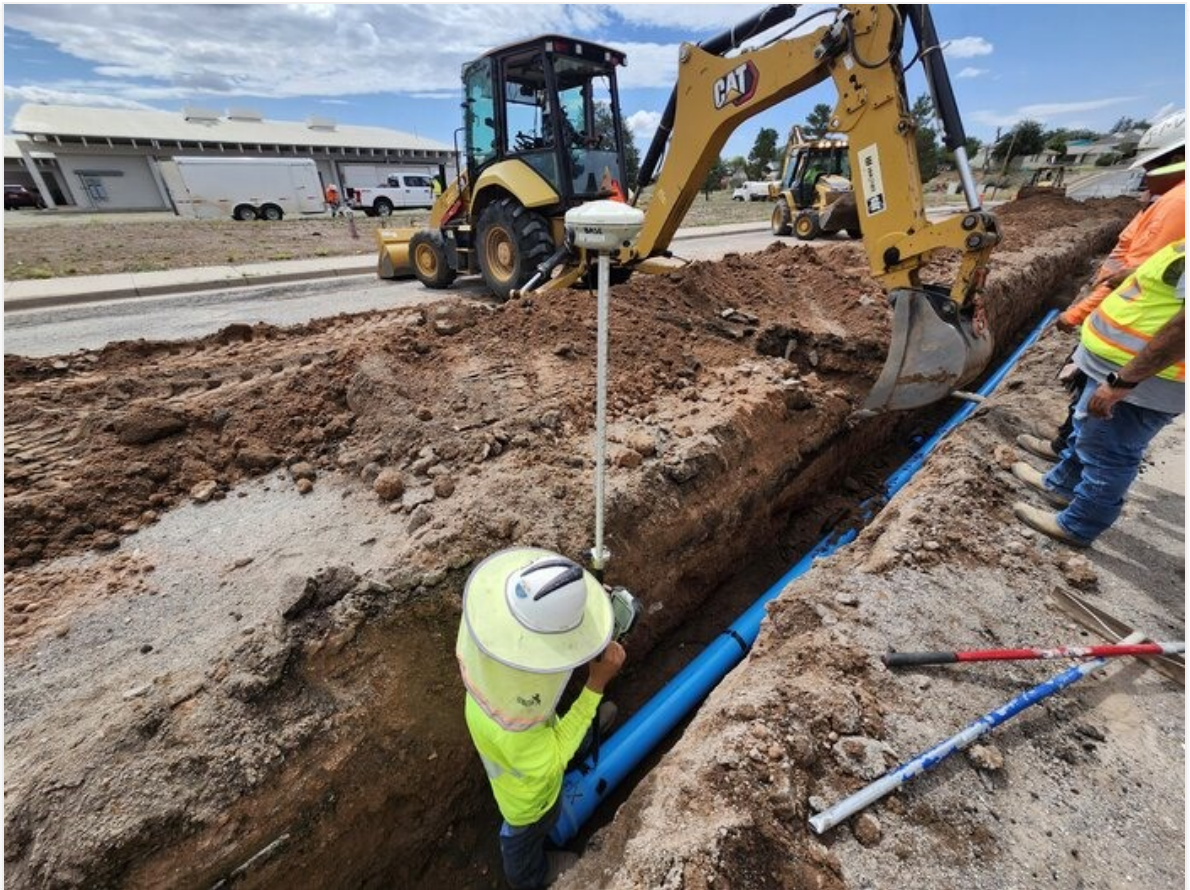
As-built survey taken on top of pipe. 6" Malachite Ave.
