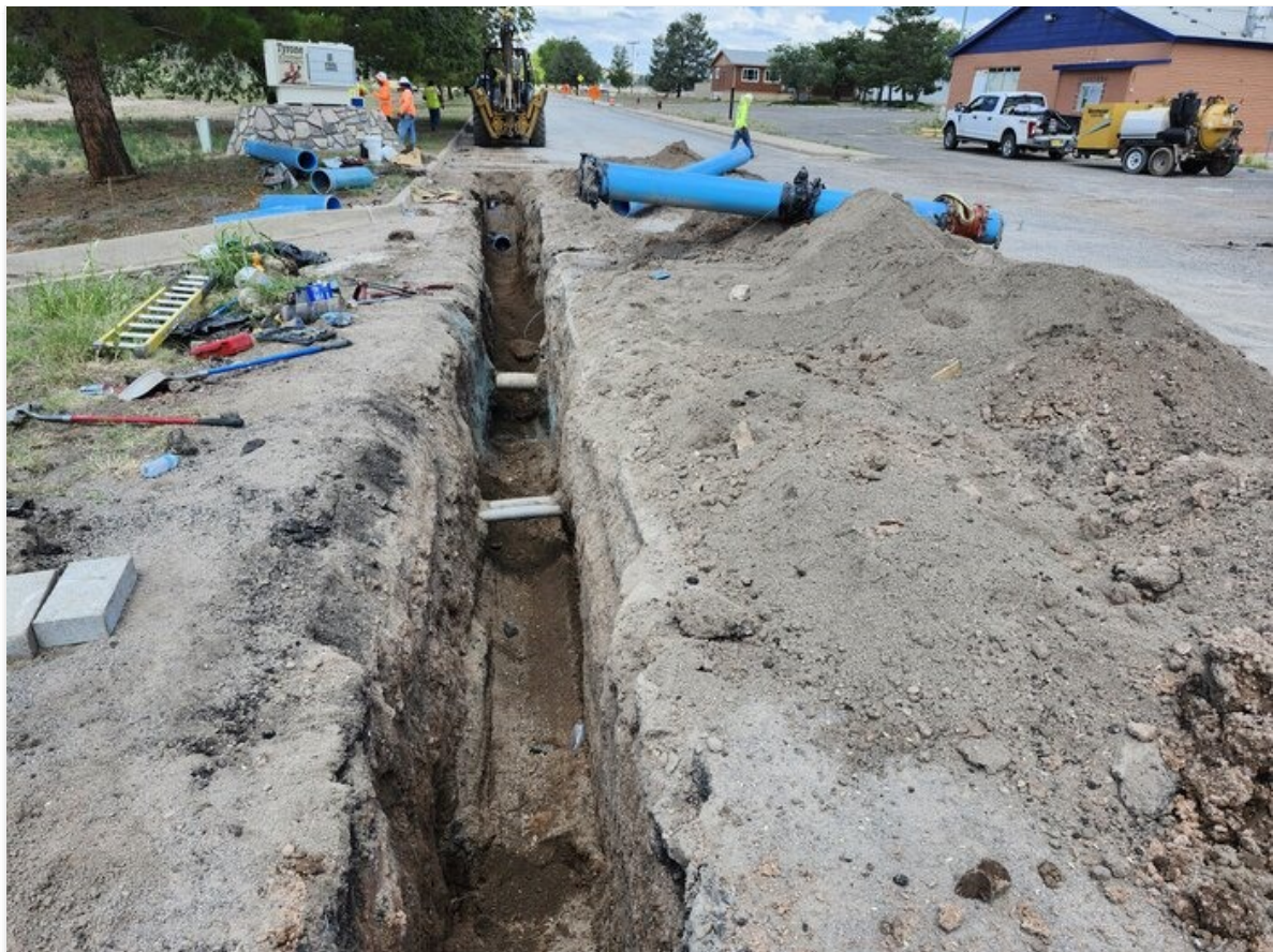
Removed 12" C-900 on Copper Dr. tie-in as per RFI #14.
