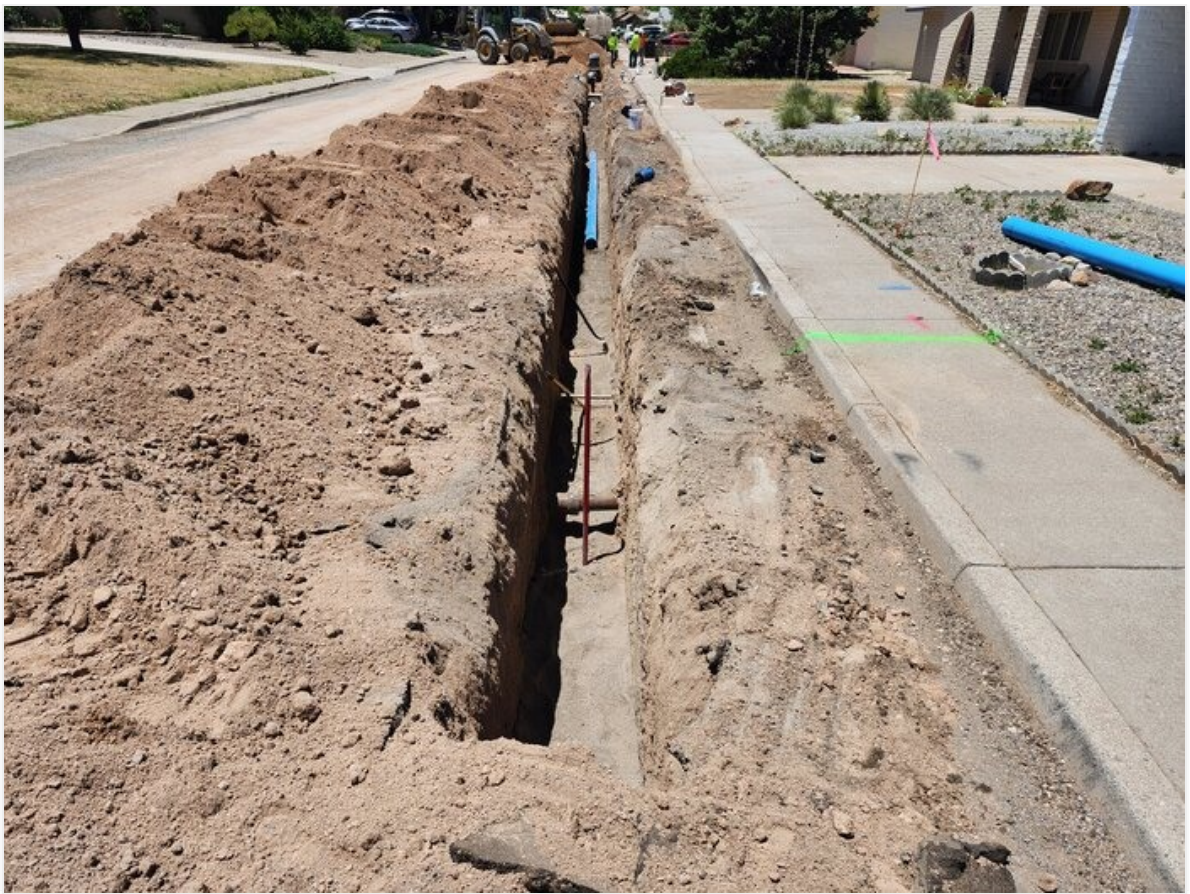
6" pipe in trench on Cuprite St.
