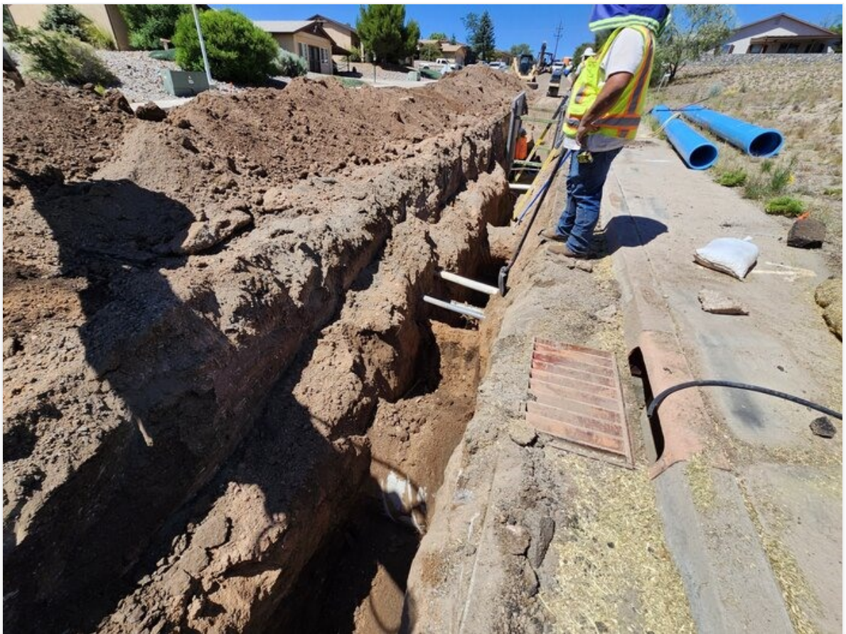
12" excavation on Cooper Dr. at sta. 22+60
