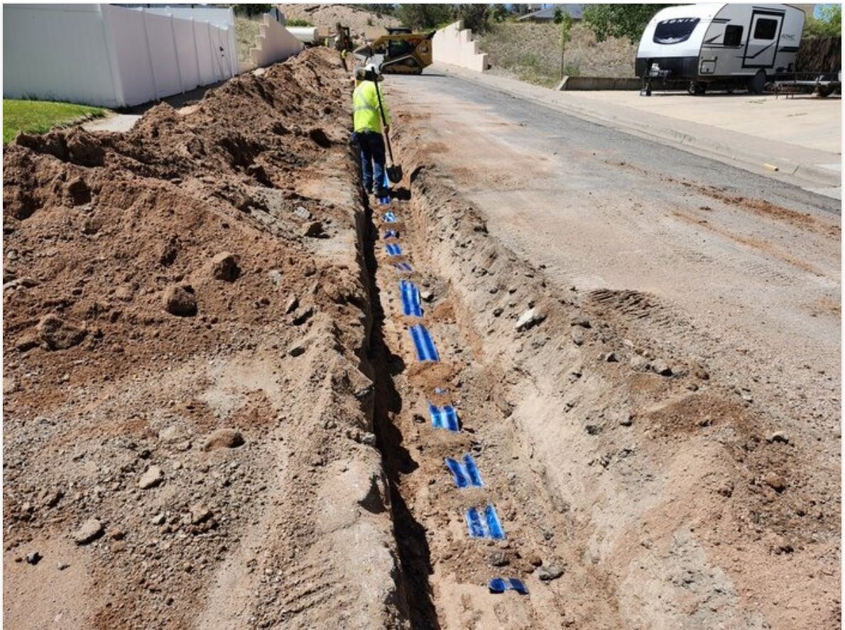
Caution tape placed in trench on Melaconite.
