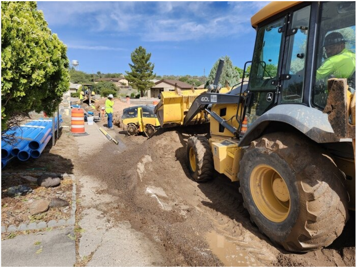
6" excavation operations on Covellite Dr.
