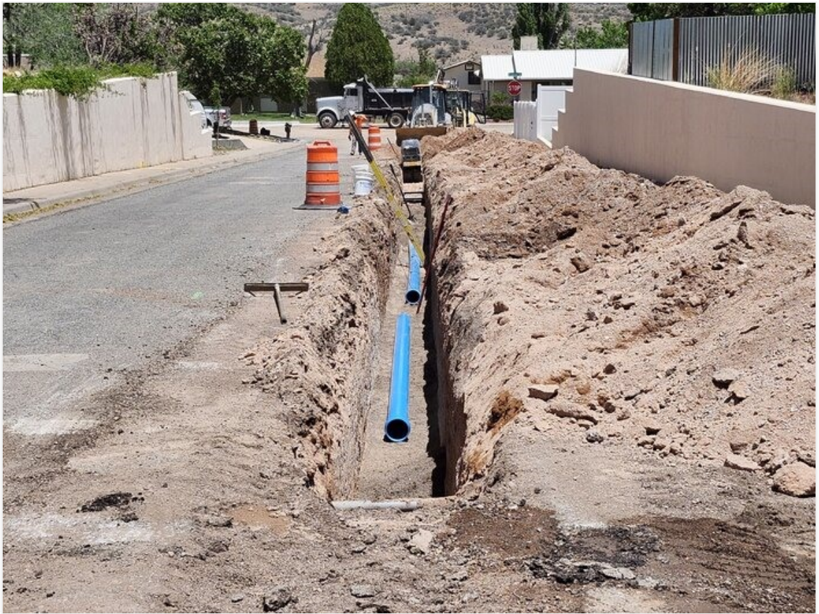
6" C-900 pipe placed in trench on Melaconite.
