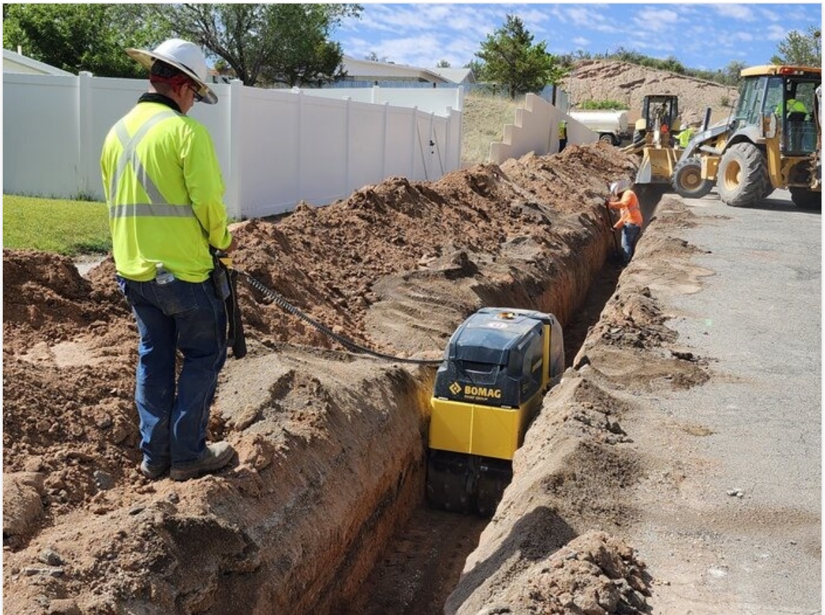
Compaction efforts at Melaconite.
