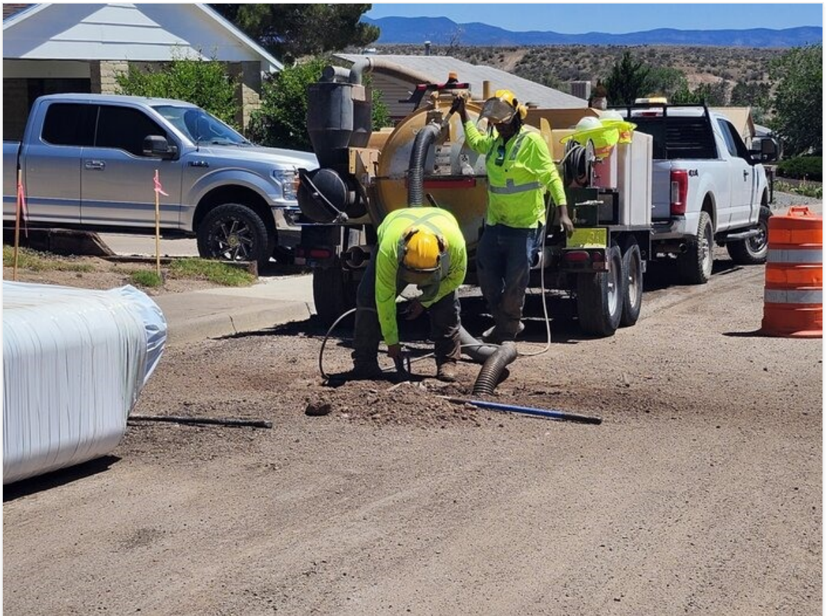
Potholing for existing utilities on Cuprite St.
