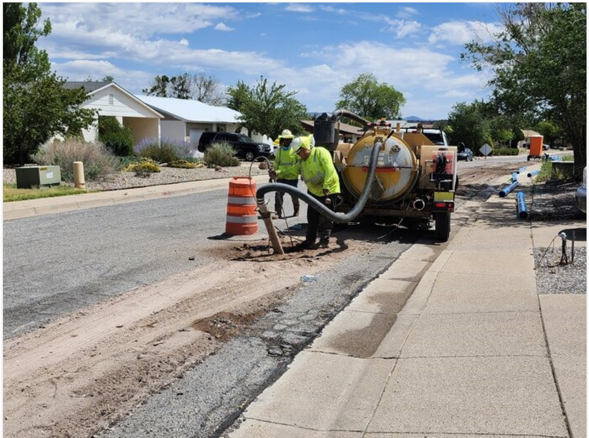
Potholing for existing utilities.
