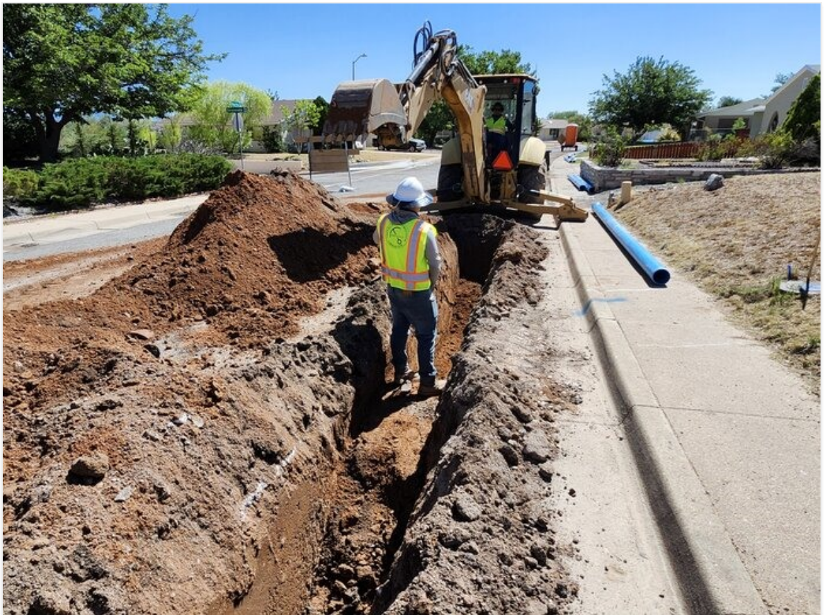
Excavation for 6" C-900 on Cuprite St.
