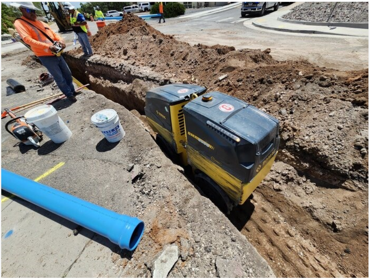
Compaction efforts over processed backfill.
