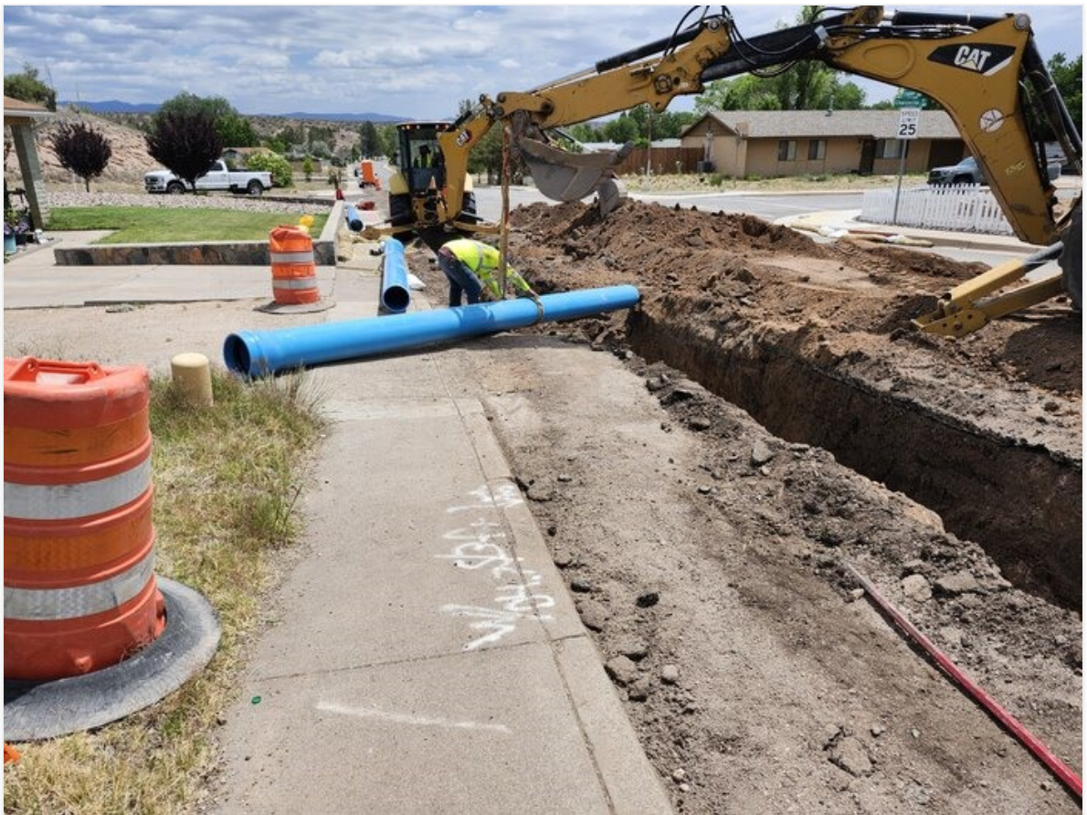
Contractor moving 12" C-900 into trench on Copper Dr.
