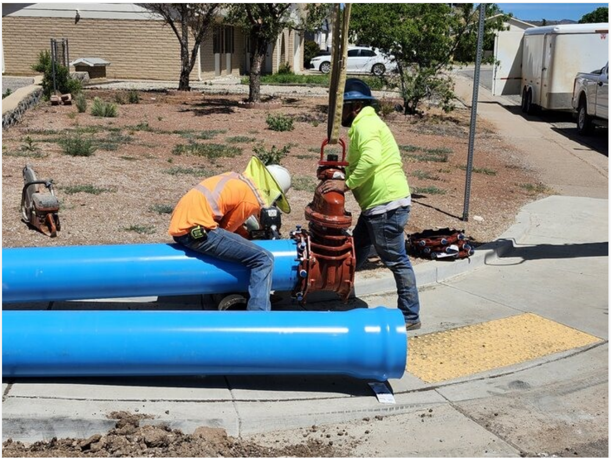
Installing GV on the 12" C-900 on Copper St.
