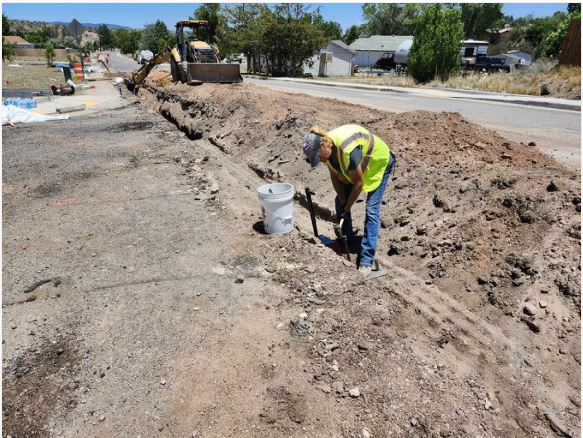
Density being taken on 6" C-900 on Cuprite St.
