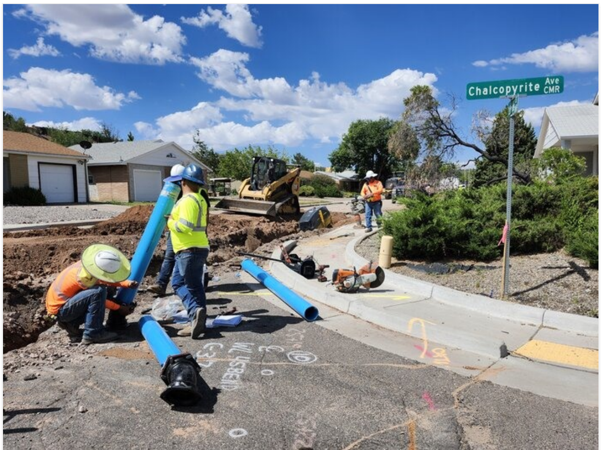
Connecting a DI 22 bend on Cuprite St.
