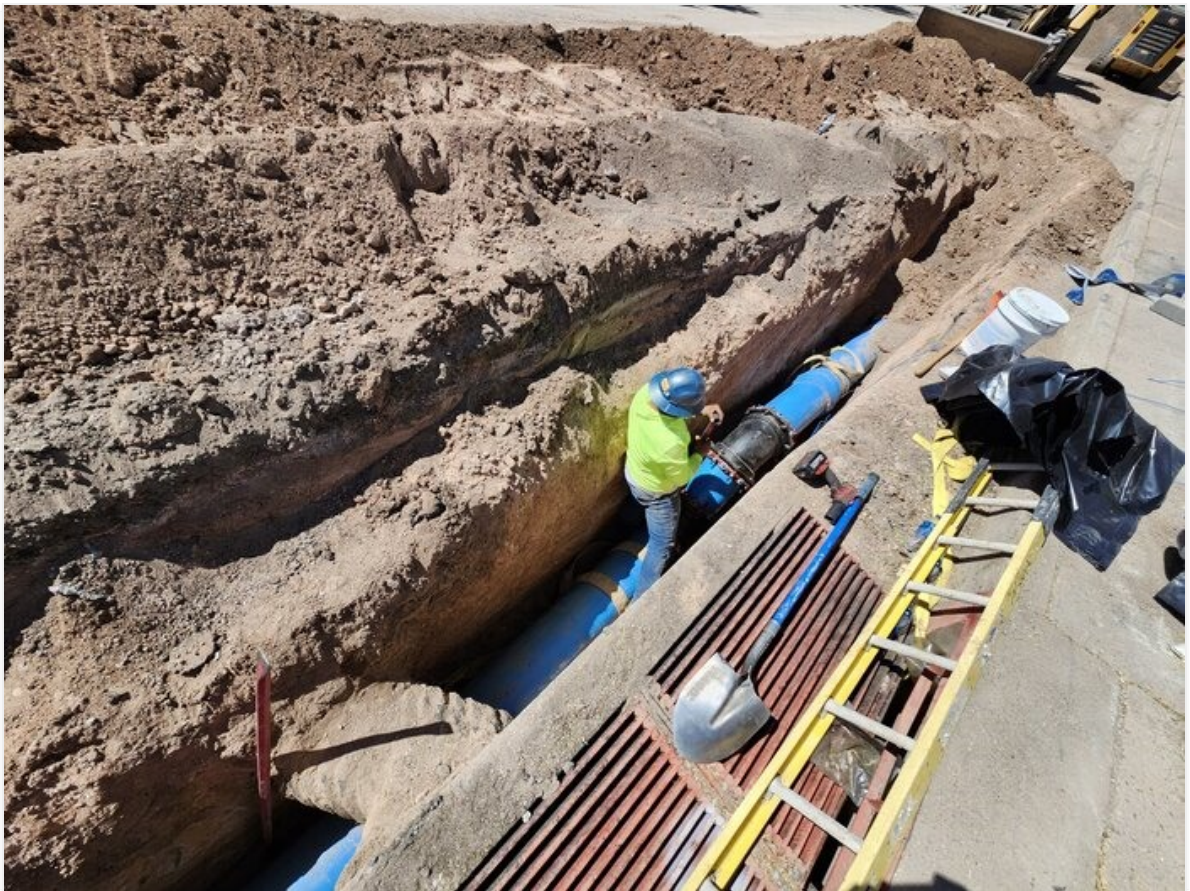
DI 45 bends going under an existing storm drain on Copper St.
