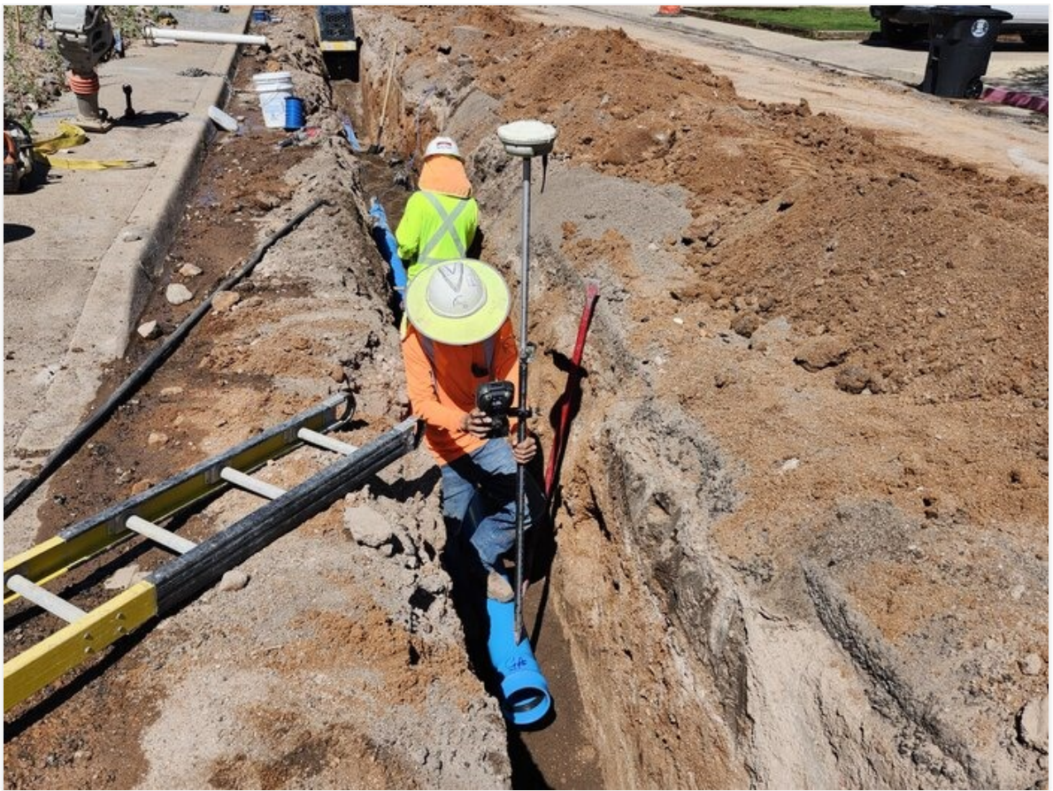
As-built survey shot on 6" C-900 pipe run
