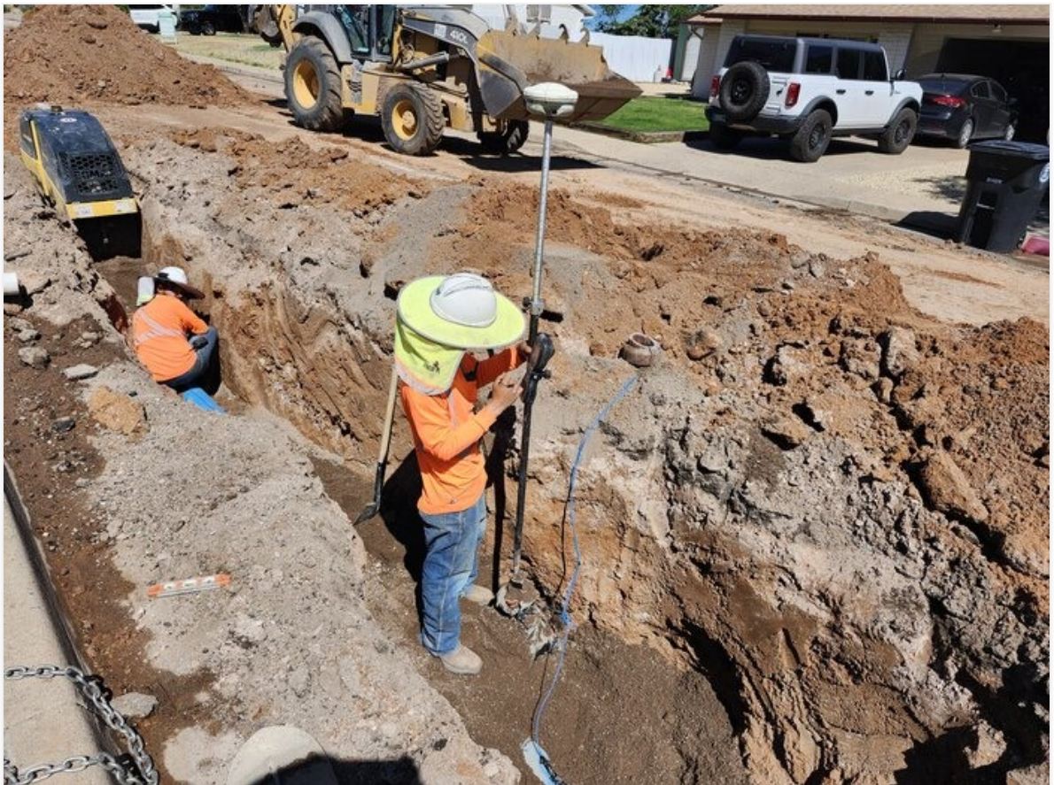
As-built survey on valve on Cuprite St.
