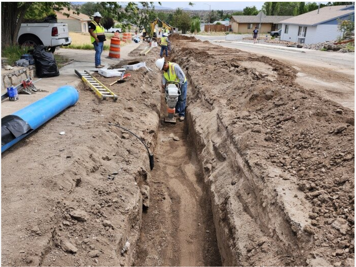
Compaction efforts for 12" C-900 on Copper Dr.
