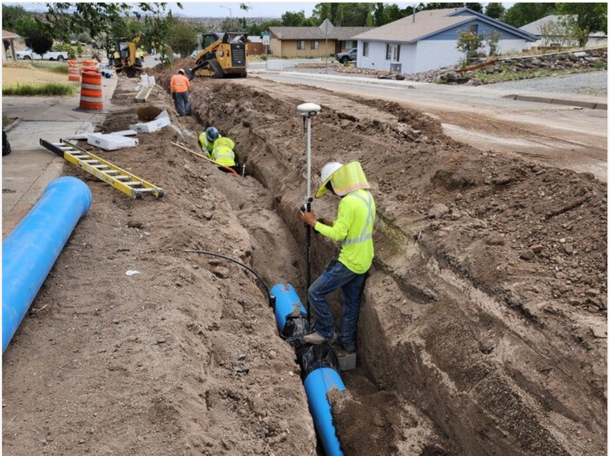
As-built survey shot being taken on DI fitting for 12" C-900
