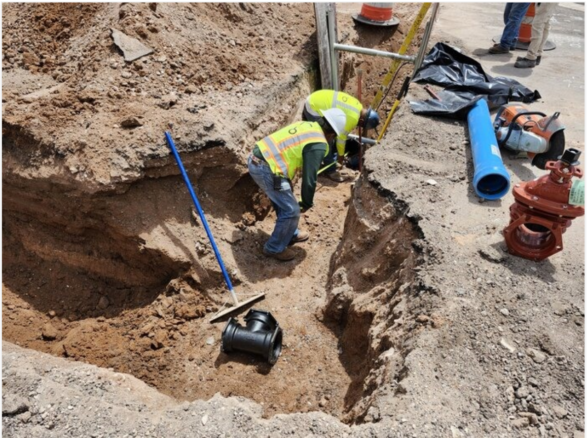
Crew getting measurements for DI 6x6x6 tee on Cuprite St. and Chalcopyrite Ave.
