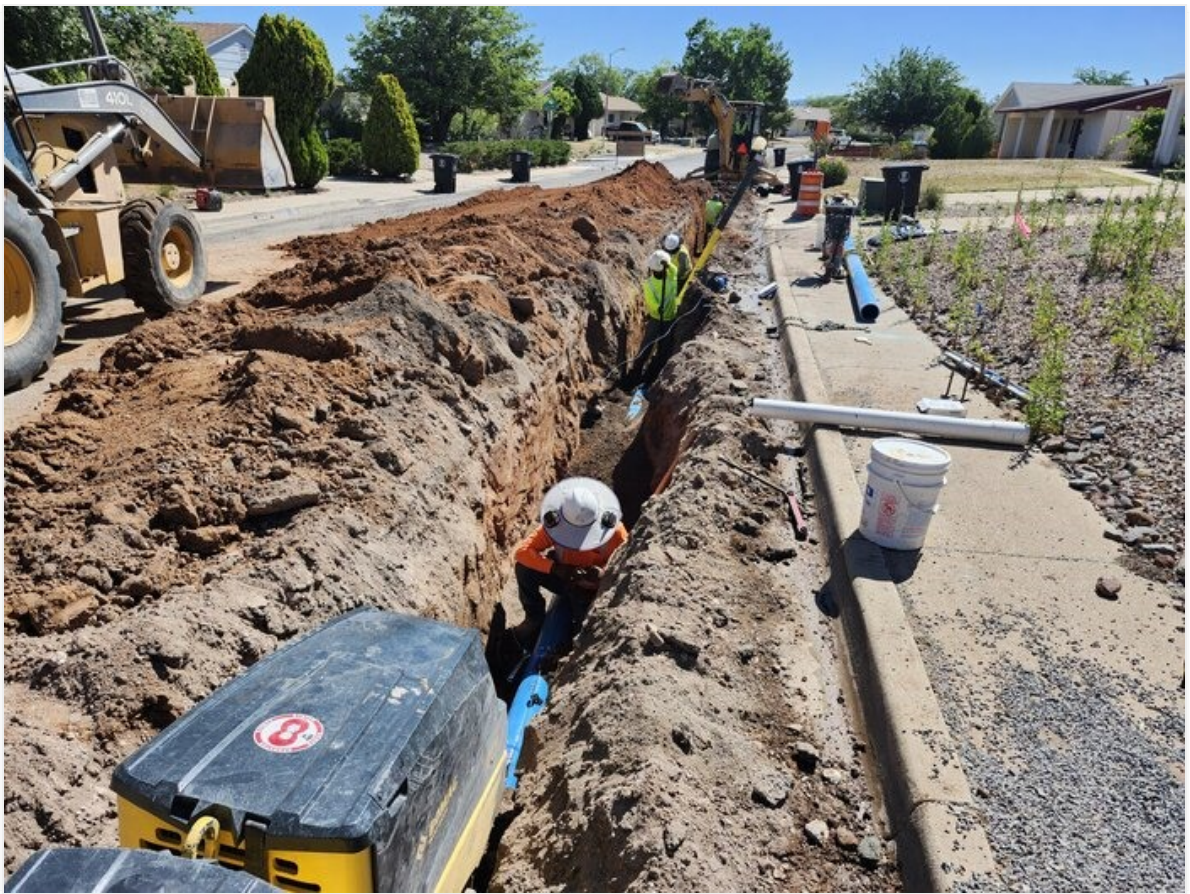
6" pipe crew placing on Cuprite St.
