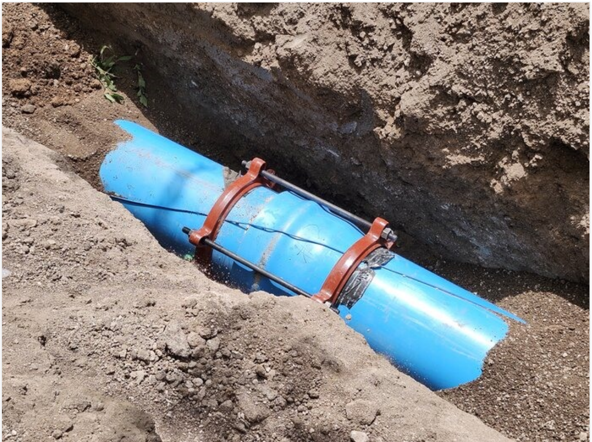
12" C-900 bell restraint on Copper Dr.
