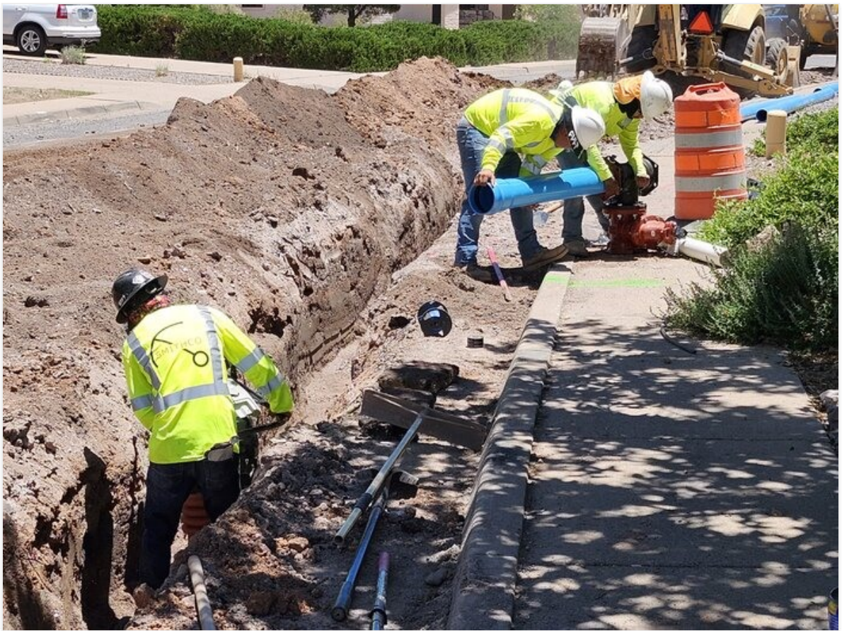
Compaction and valve assemble for 6" C-900 on Cuprite St.
