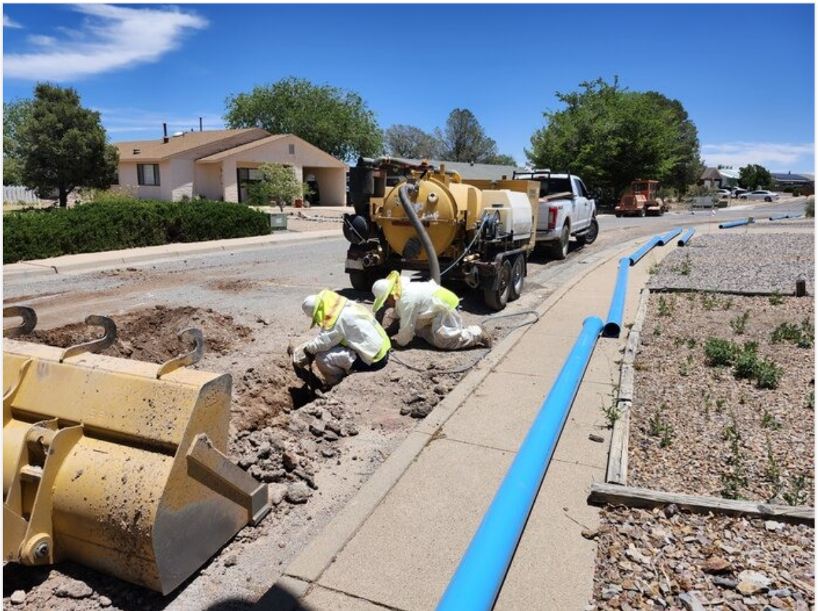
Potholing ahead of excavation for existing utilities on Cuprite St.
