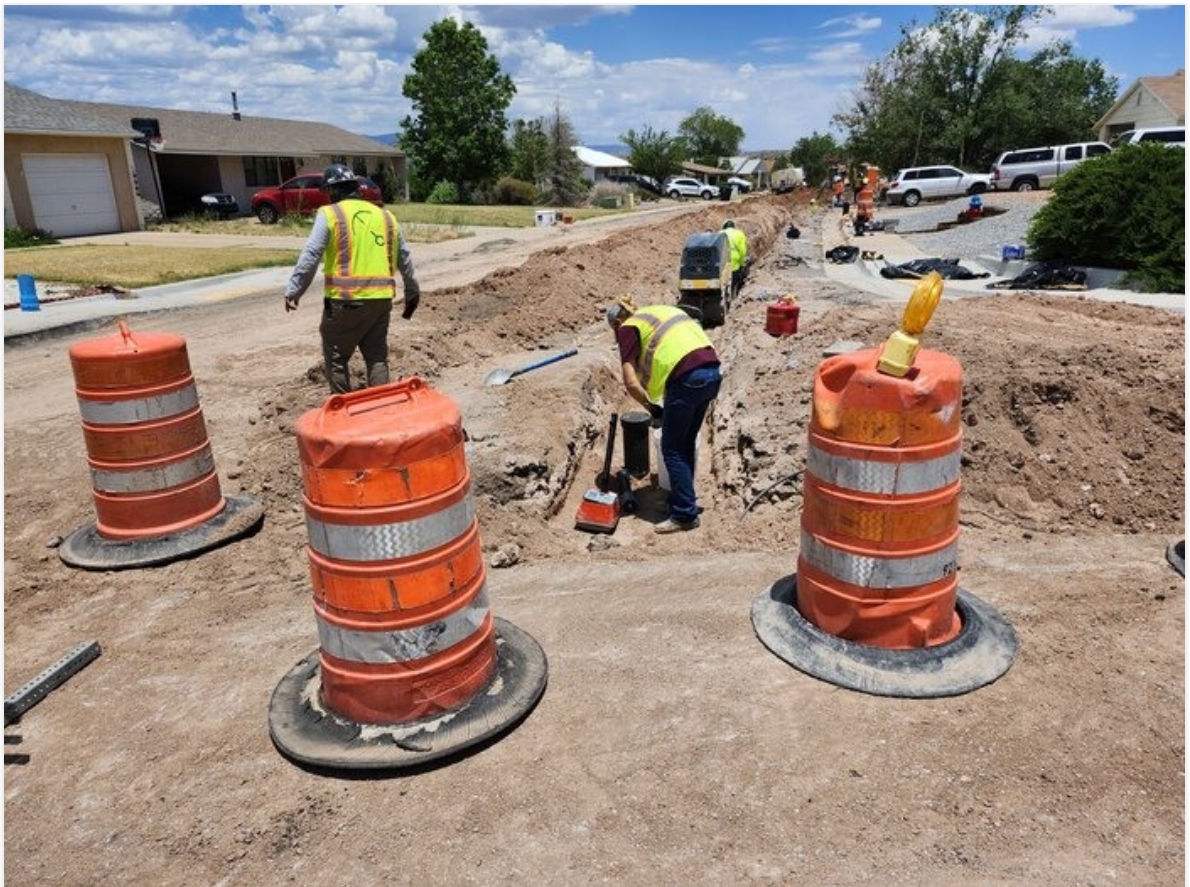
Density being taken on Cuprite St. for 6" C-900.
