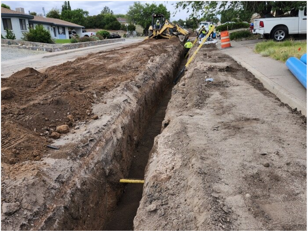
Trench for 12" C-900 on Copper Dr.
