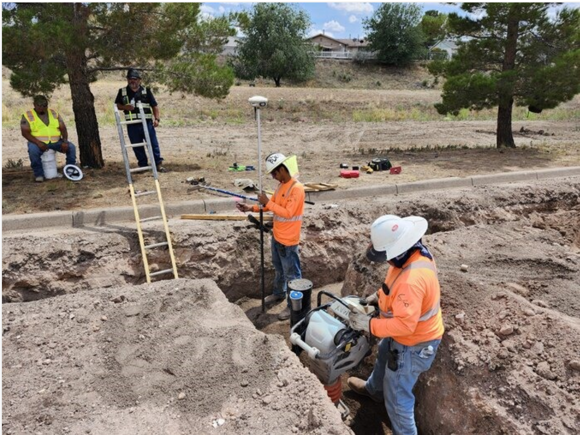
Survey as-built shots on 12x6 tee. (Copper Dr.)
