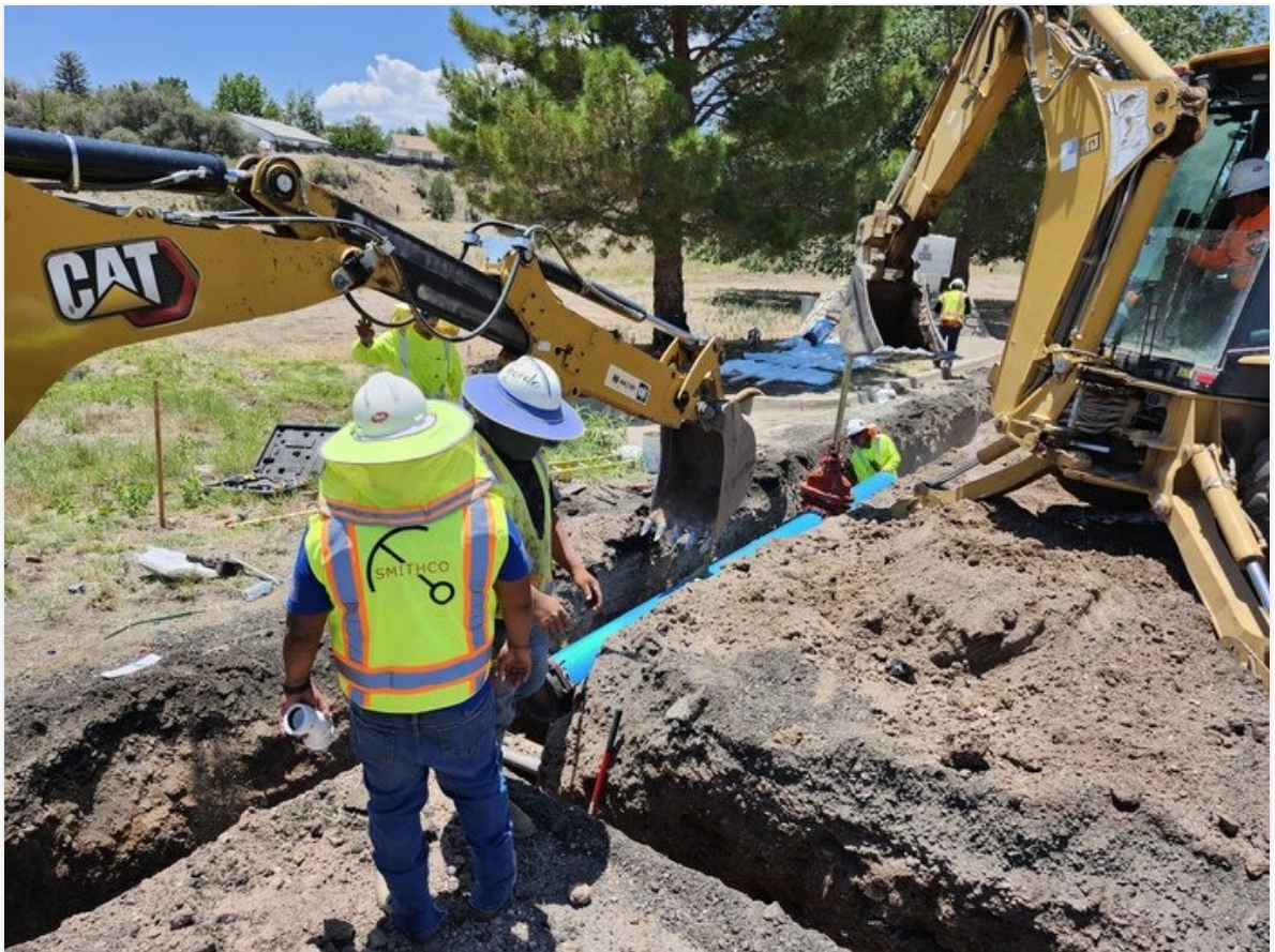
Placing valve and cap into open trench.
