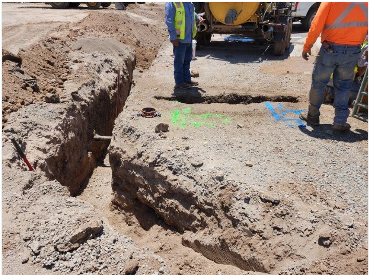
Moved 45 bend due to existing utilities in conflict at tie in on Chrysocolla Ave.
