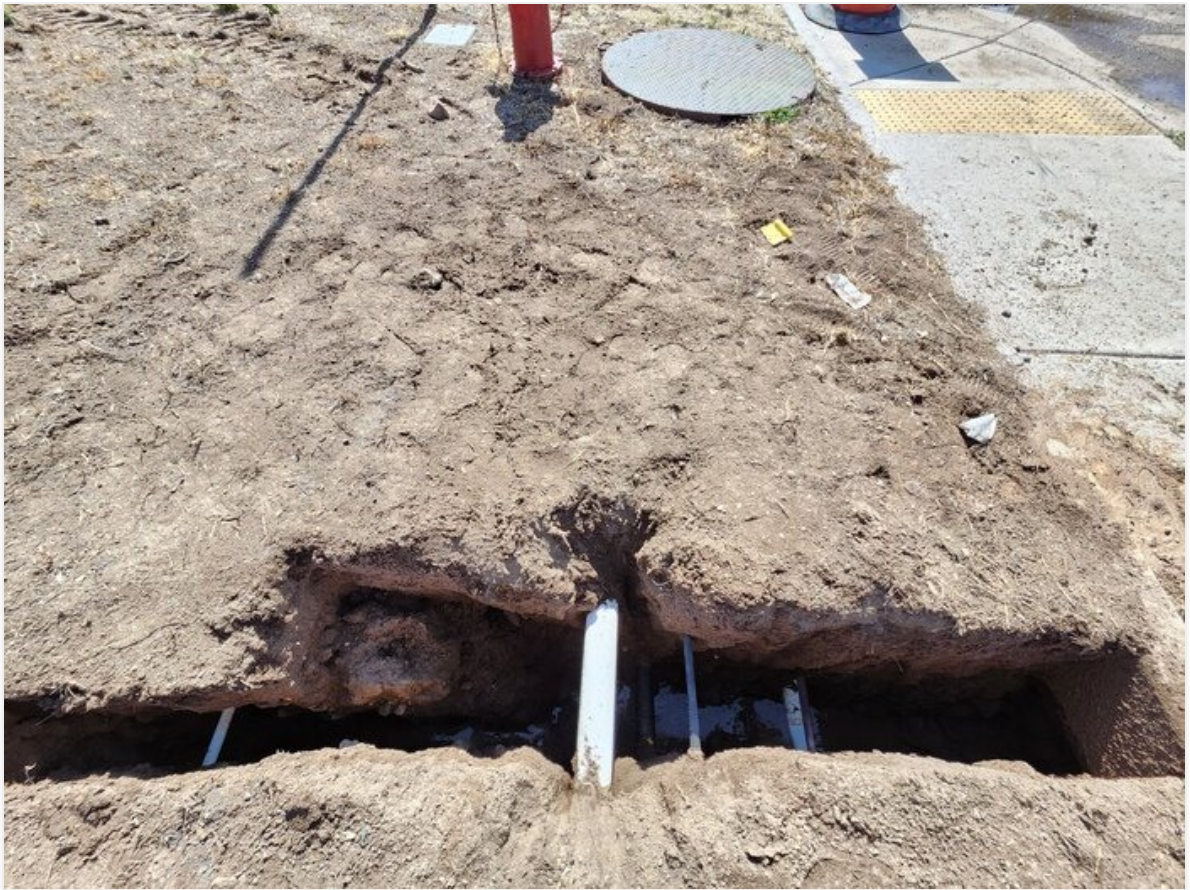
Existing utilities in proposed hydrant location on Copper Dr. sta. 59+87.
