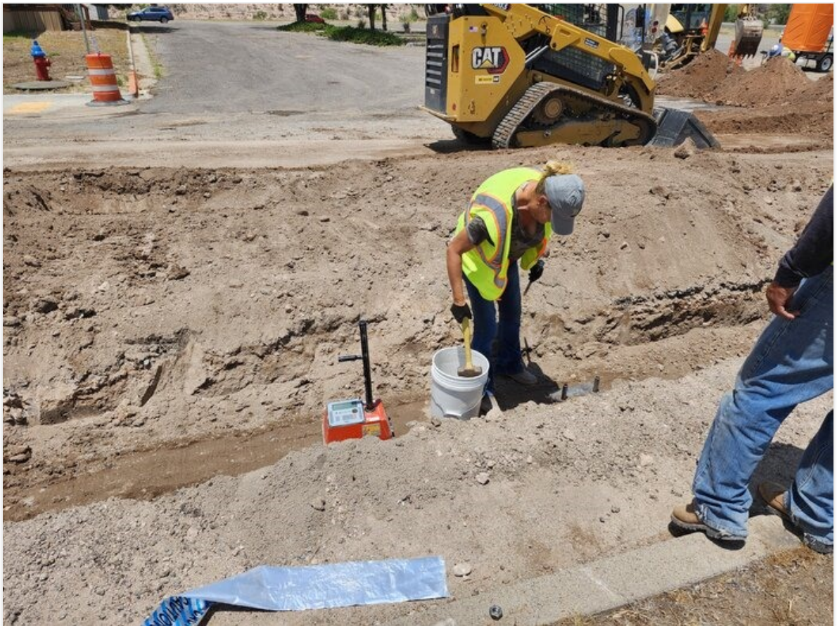
Summit Testing taking backfill densities over 12" C-900 on Copper Dr.
