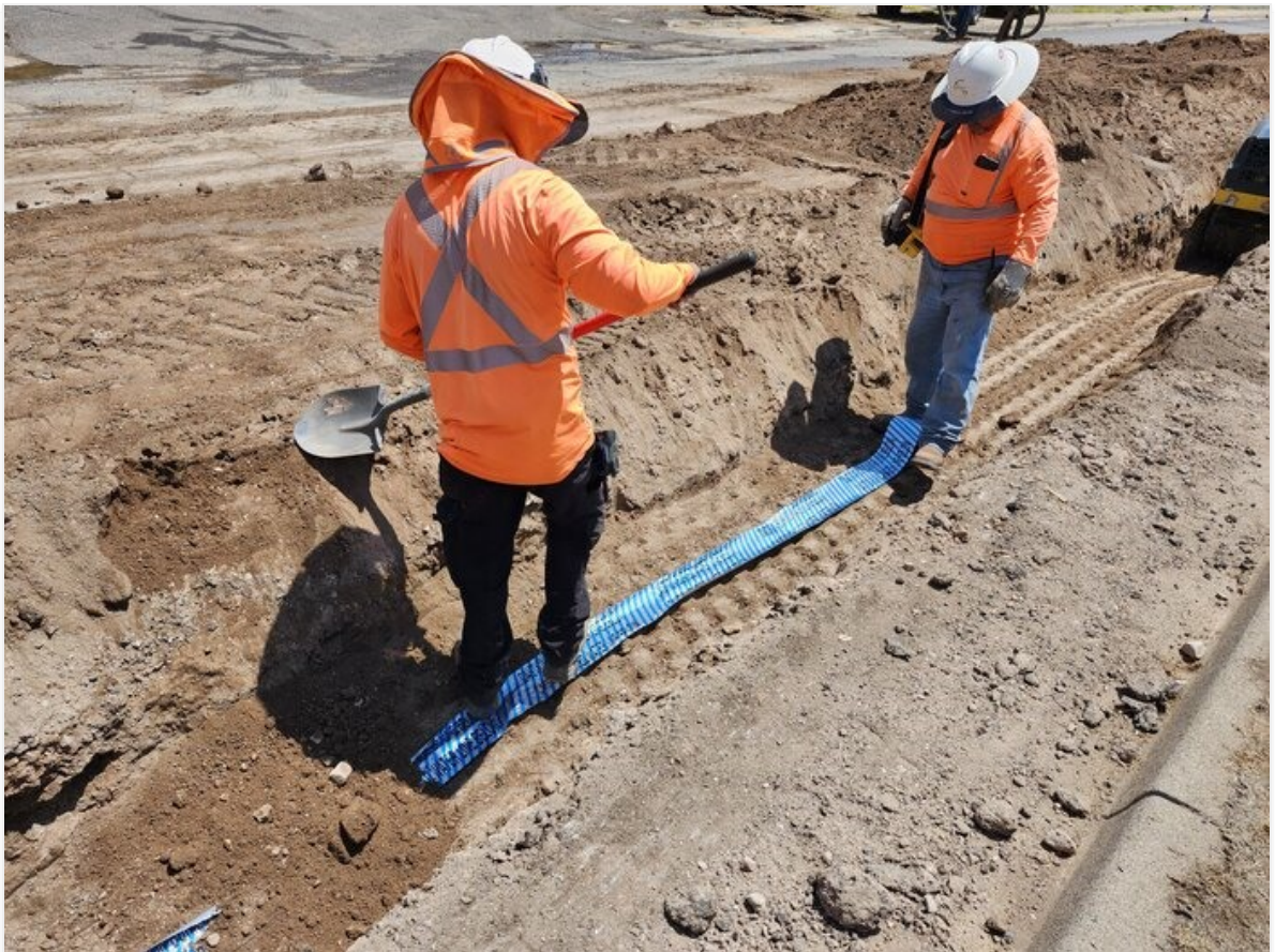
Detectable warning tape over 12" C-900 on Copper Dr.
