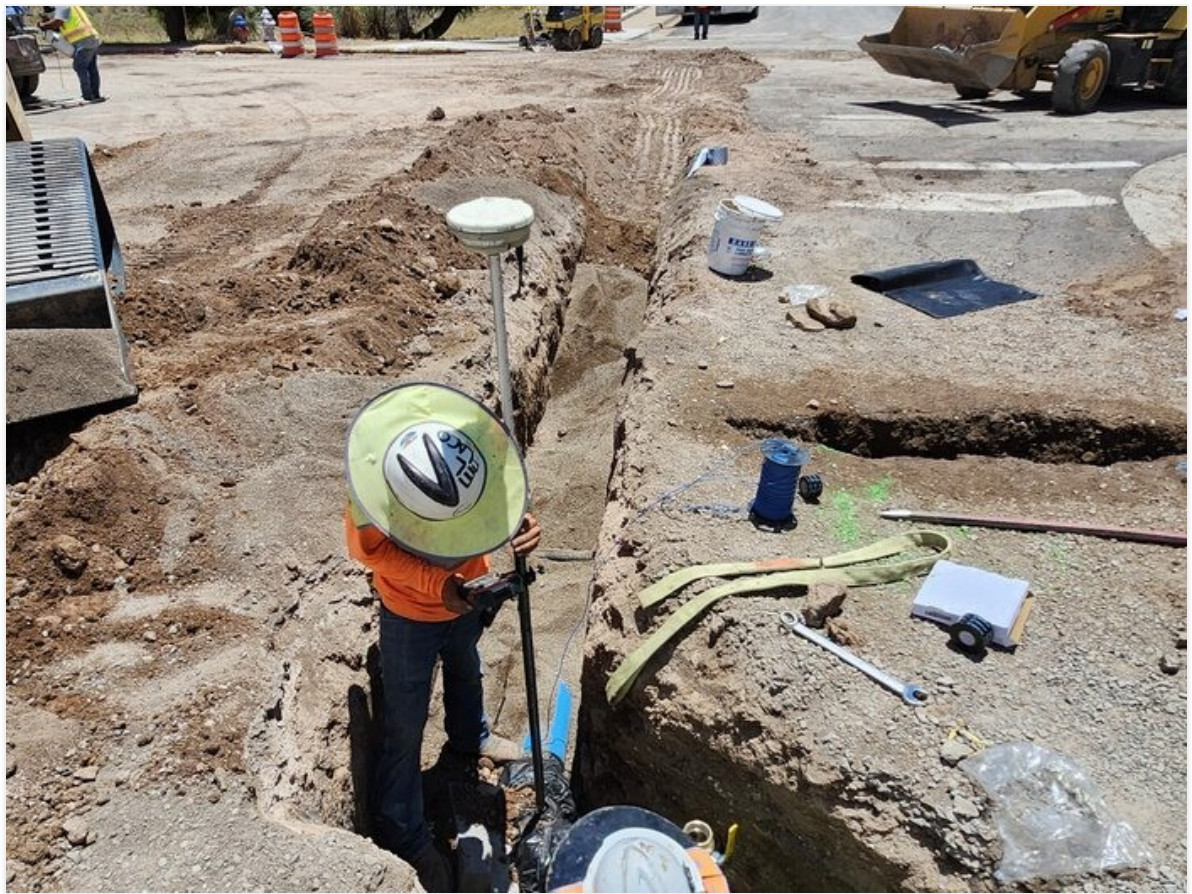
As-built survey shot of 45 Di bend on Chrysocolla Ave,
