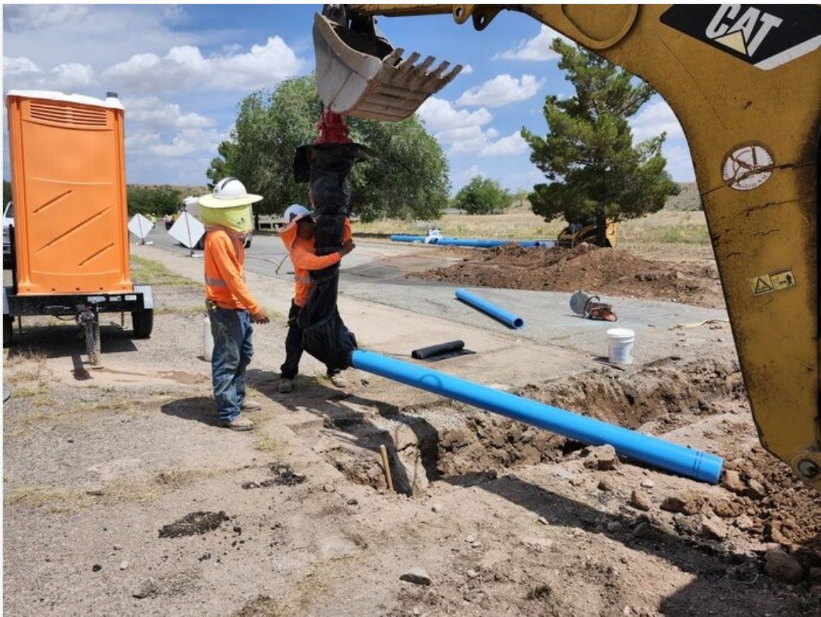
Fire hydrant being placed as per detail plan. Copper Dr.
