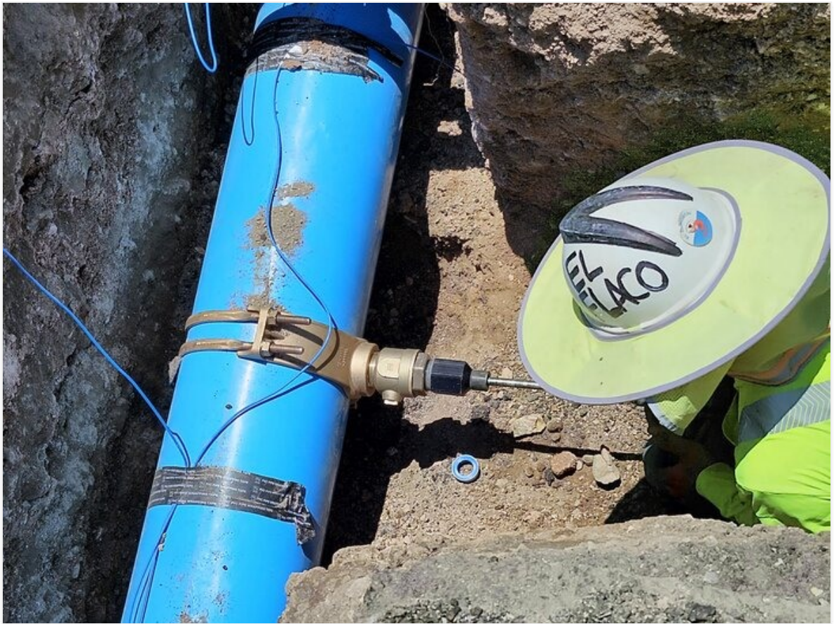
Drilling 2" saddle tap on 12" C-900 on Copper Dr.
