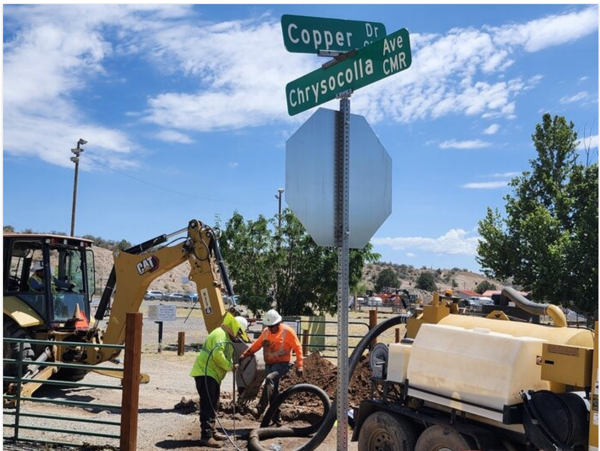
Potholing for existing water line.
