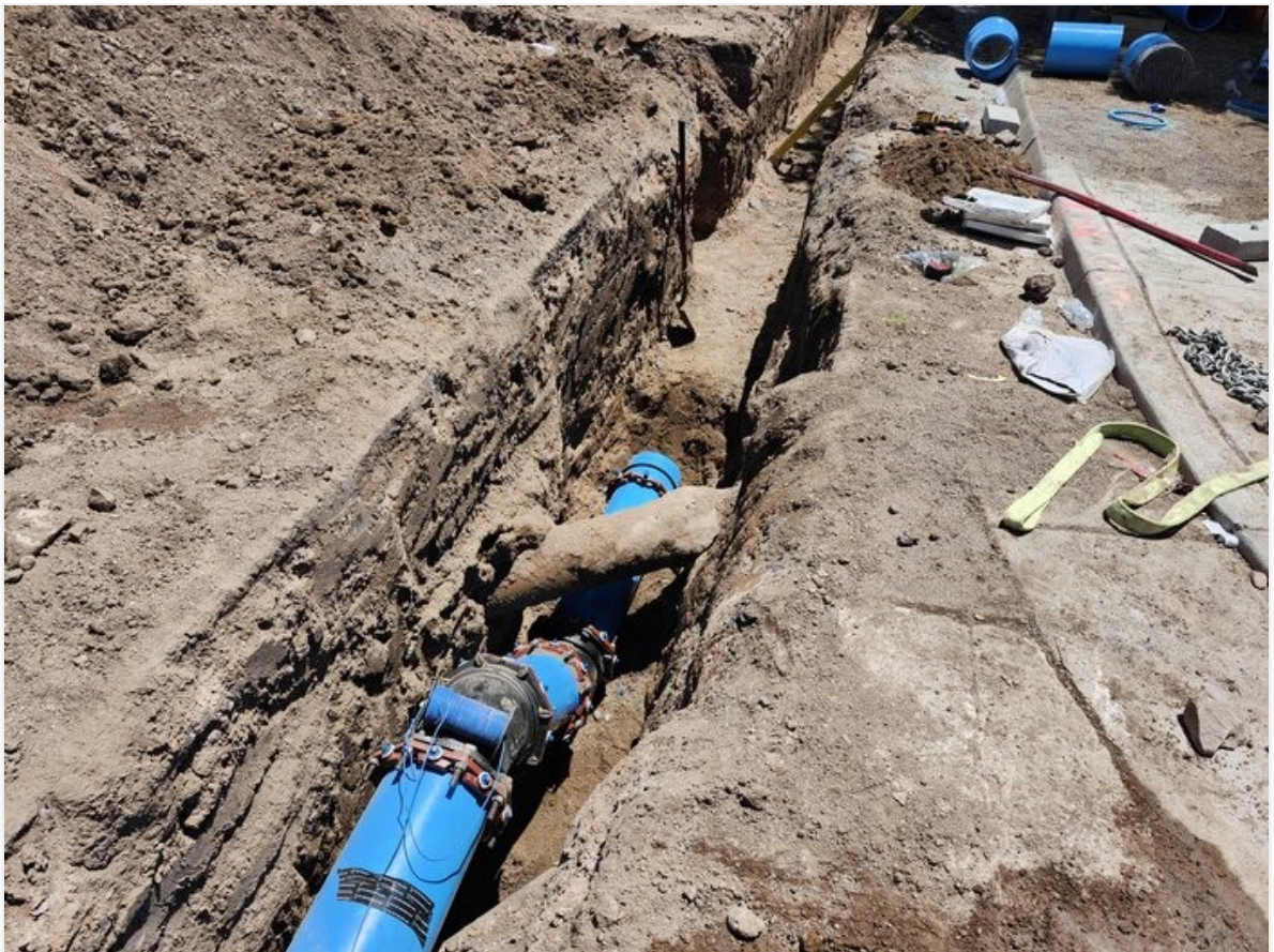
DI 45 bends being placed under unknown 10" clay pipe on Copper Dr. sta. 56+47.
