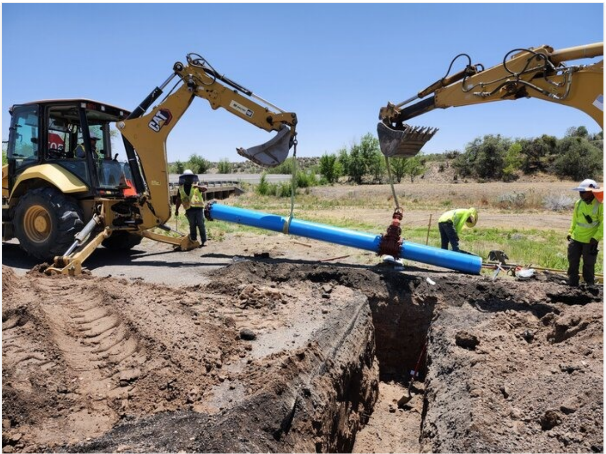
Valve and 12" cap at the EOP of Copper Dr.
