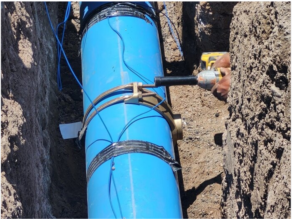
Tightening 2" double strap saddle onto 12" C-900
