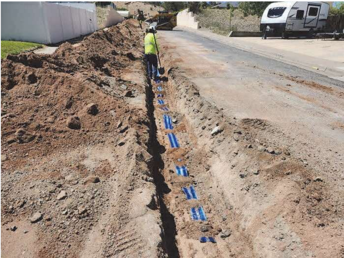
Caution tape placed in trench on Melaconite.
