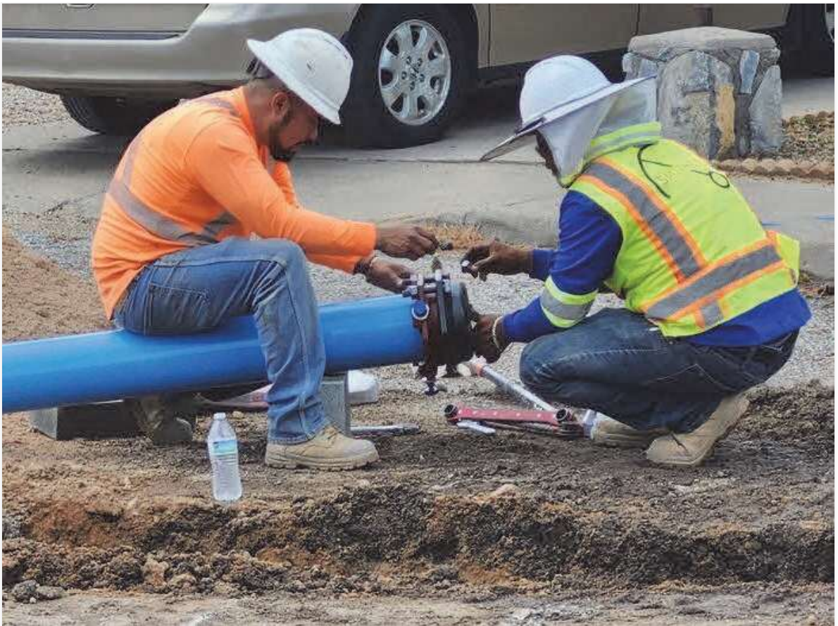
DI cap being placed on 6" C-900 on Covellite Dr.
