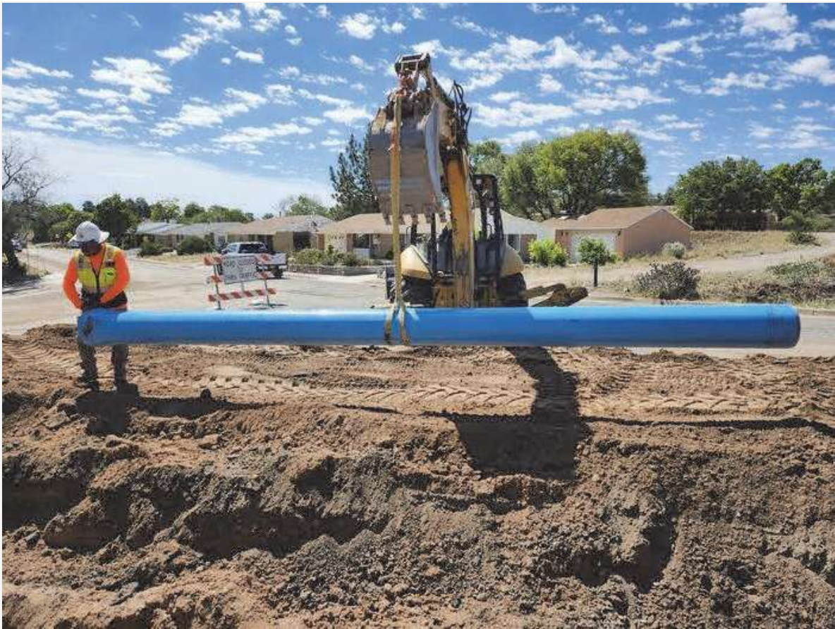
12" C-900 being placed into trench on Cooper Dr.
