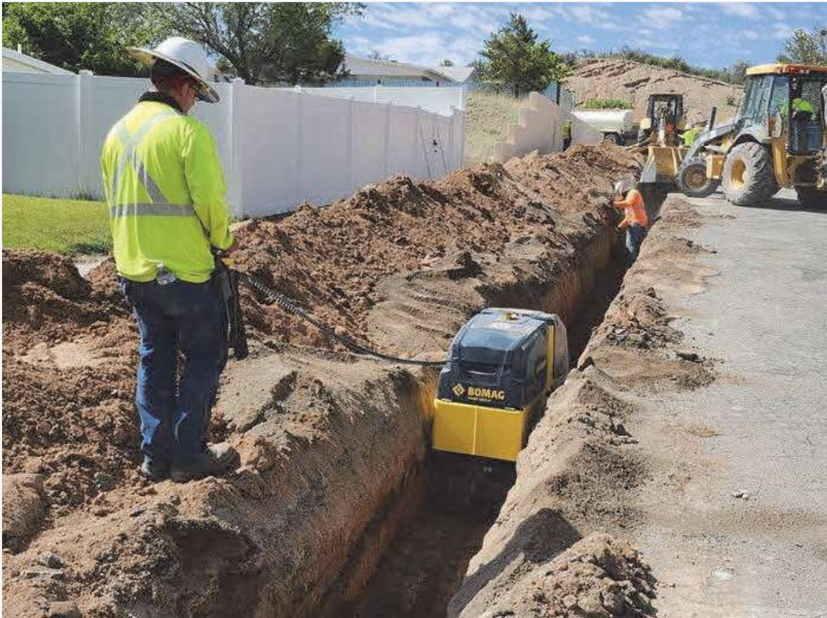
Compaction efforts at Melaconite.
