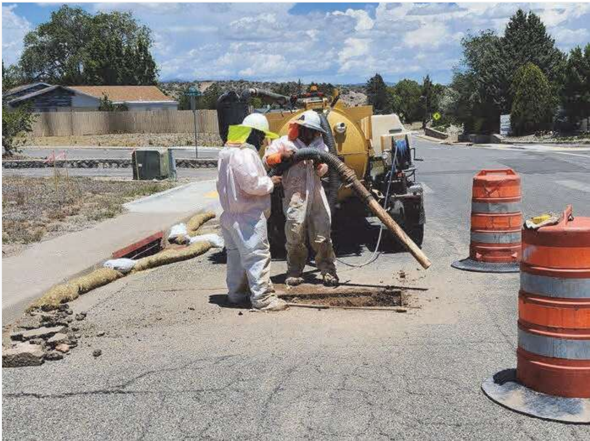
Potholing on Copper Dr. for existing water line.
