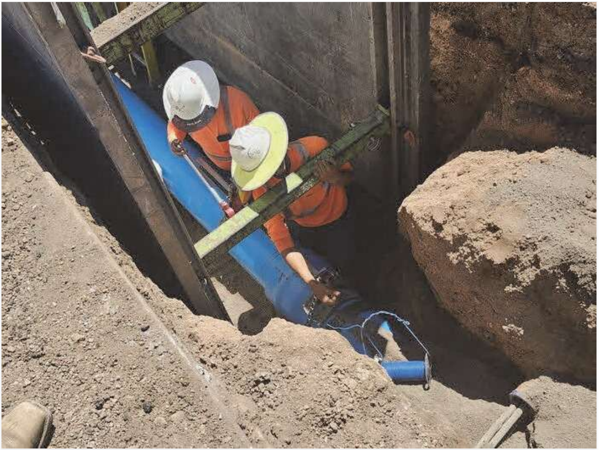
Crew using special tool to pull 12" C-900 together at the bell.
