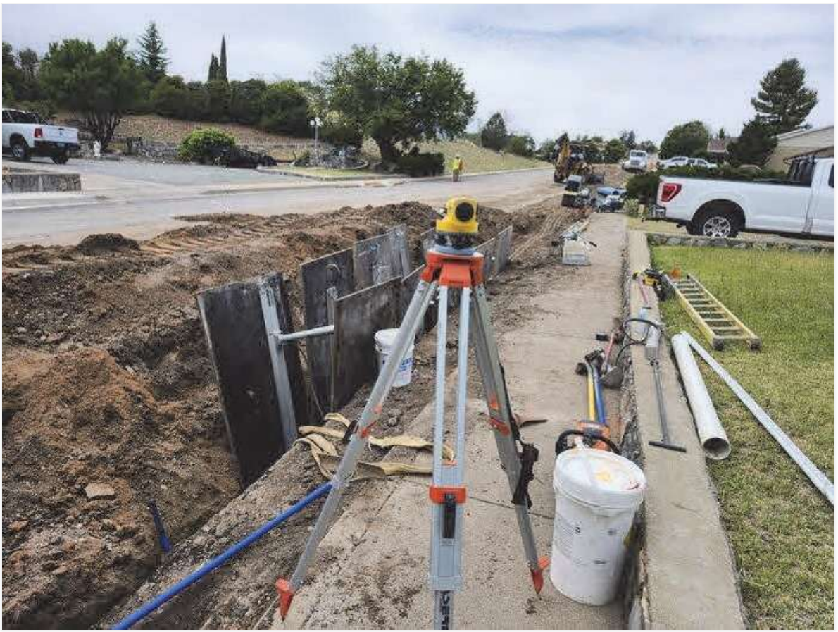
Shoring needed on Cooper Dr. for the placement of 12" C-900.
