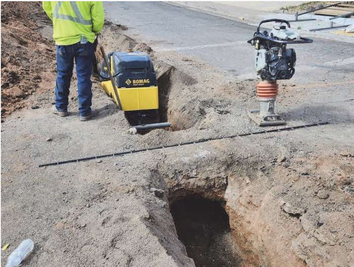
Compaction efforts at Melaconite and Cuprite St. intersection.
