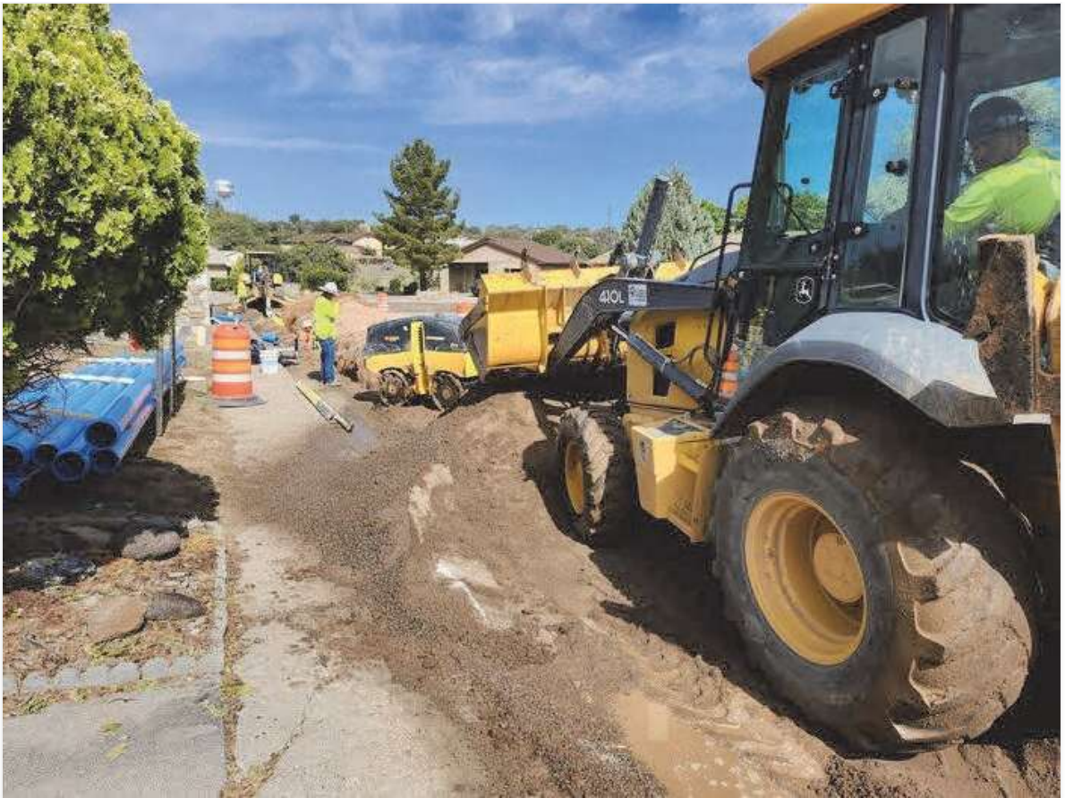
6" excavation operations on Covellite Dr.
