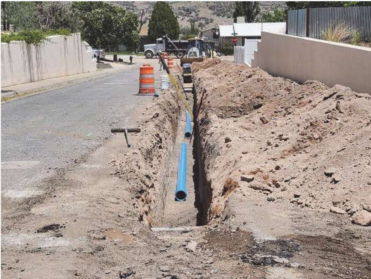
6" C-900 pipe placed in trench on Melaconite.
