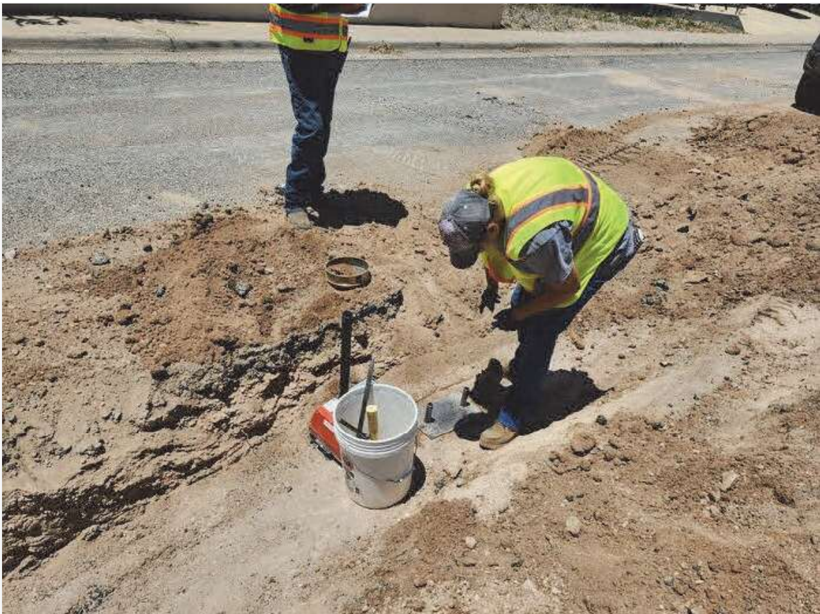
Summit testing technician taking densities on 12" C-900.
