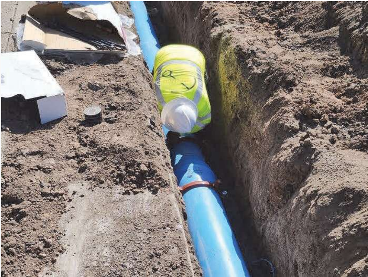
12" C-900 pipe restraint being installed after a GV.
