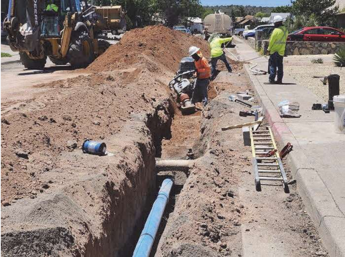
6" C-900 backfill and compaction efforts on Cuprite St.
