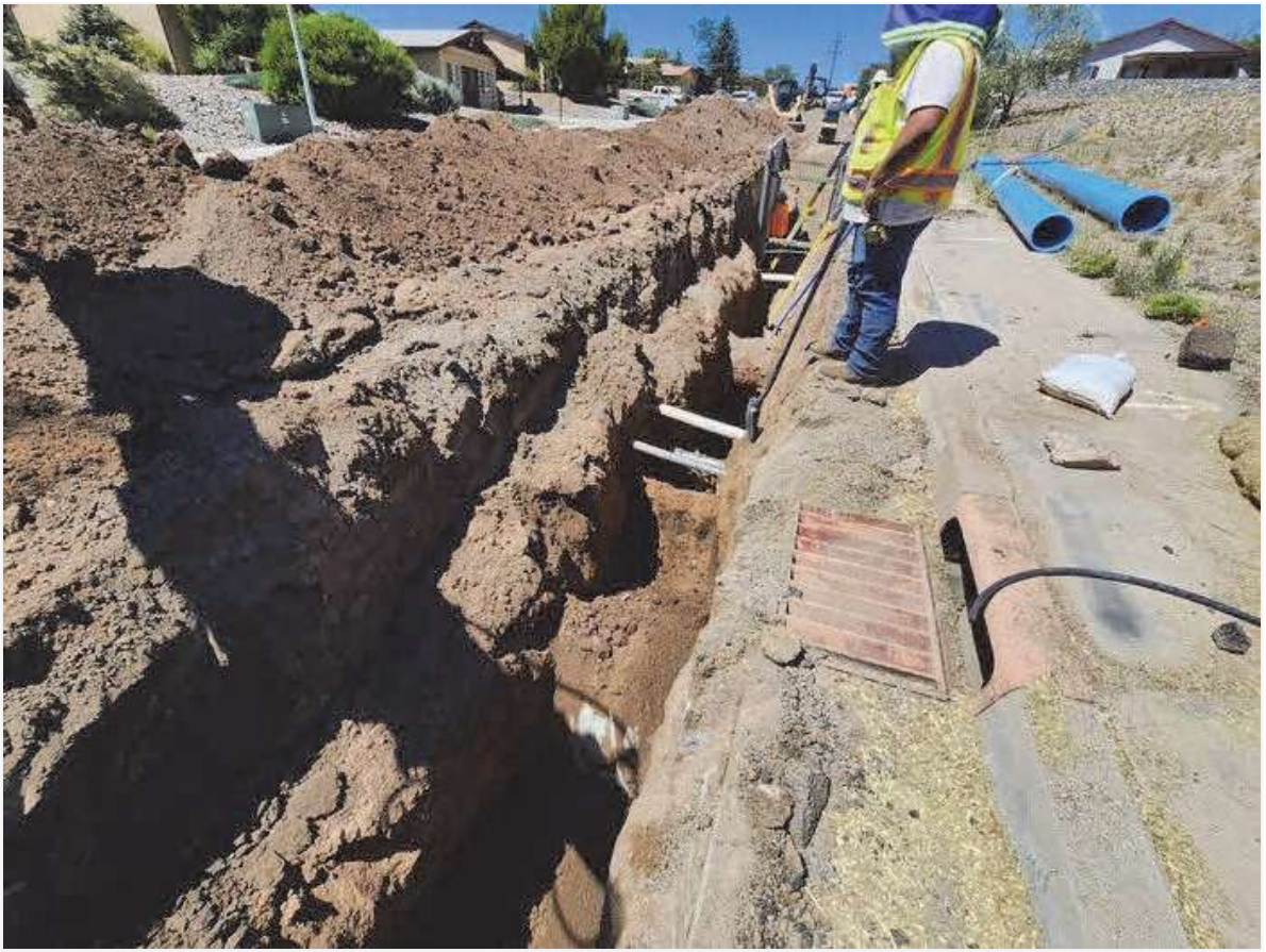
12" excavation on Cooper Dr. at sta. 22+60
