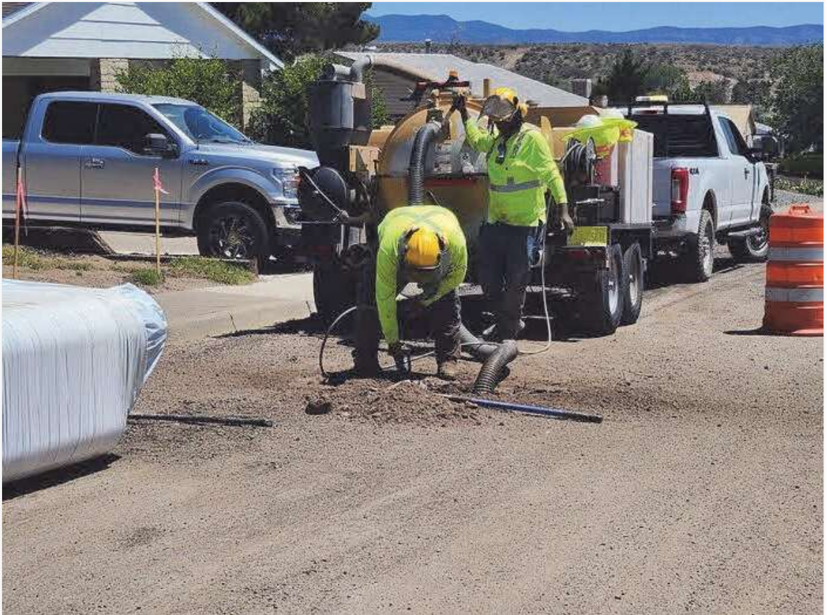
Potholing for existing utilities on Cuprite St.
