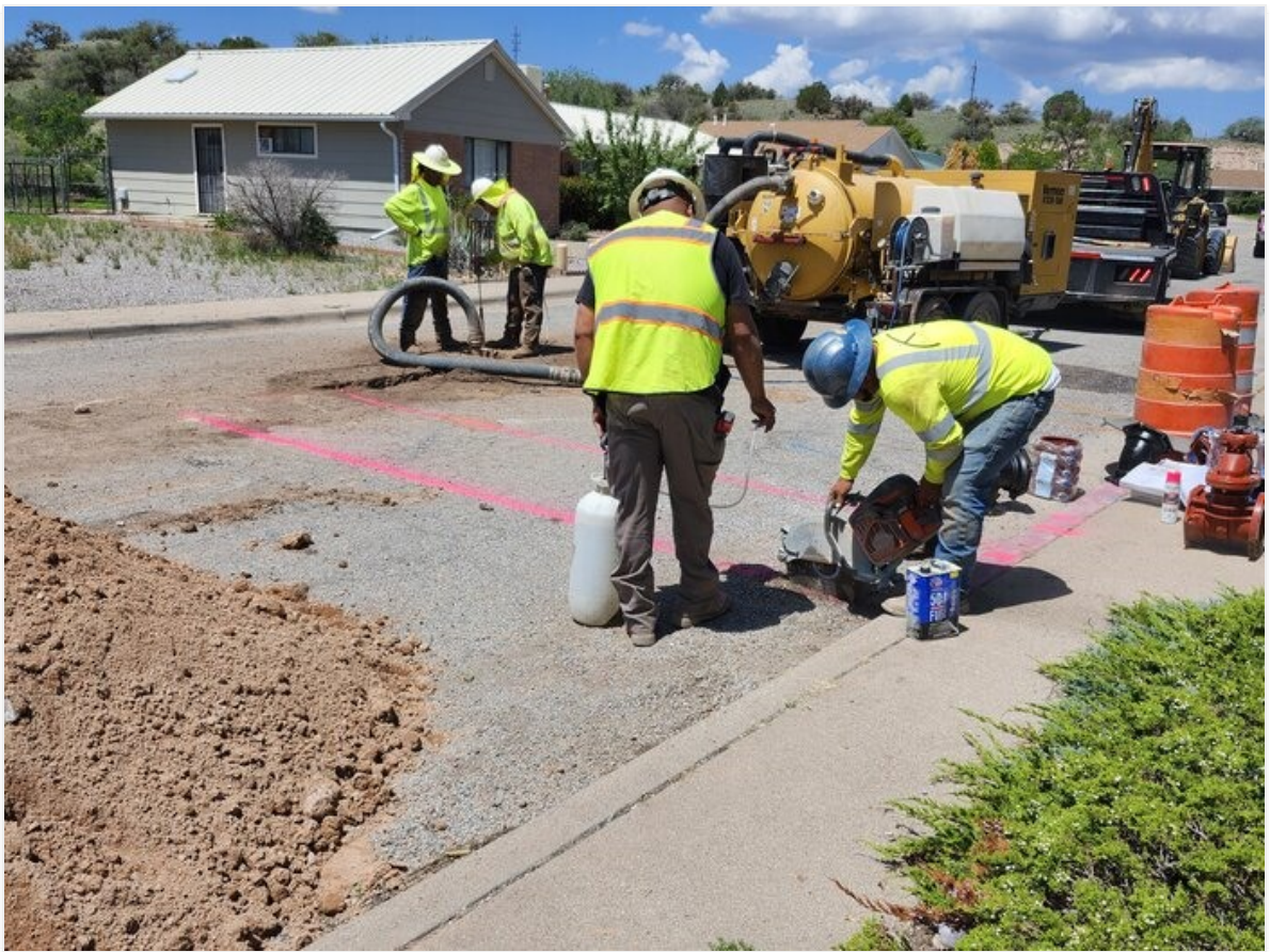
Saw cutting roadway for hydrant #11.
