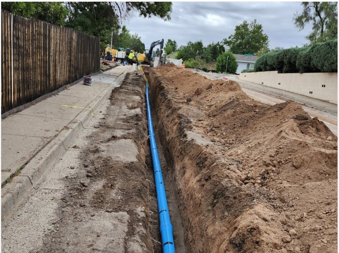
6" C-900 on Chalcopyrite Ave.
