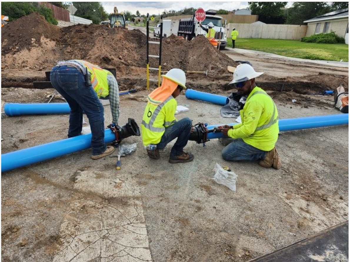
45 DI bends to go under existing 48" storm drain at Chalcopyrite and Copper.
