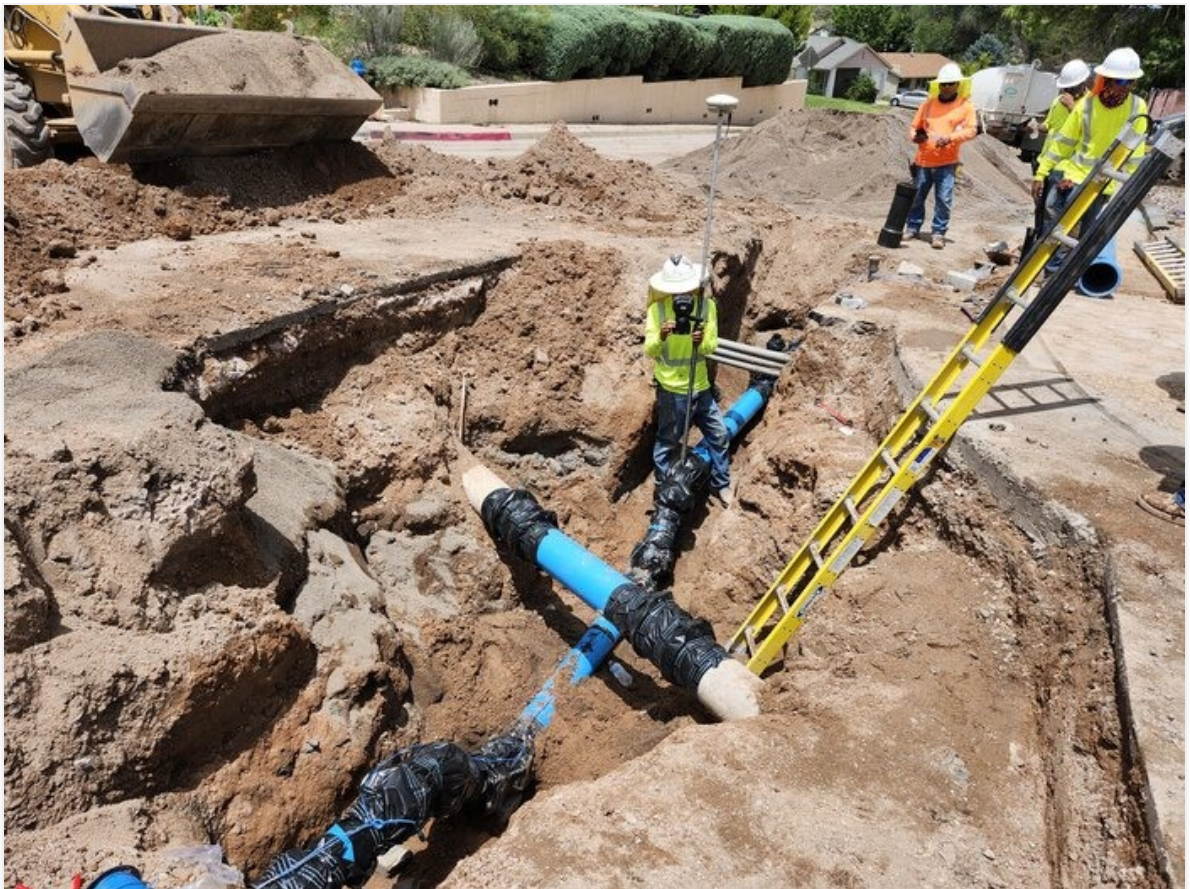
6" C-900 with 45 DI bends under repaired 8" AC line on Cuprite and Chalcopyrite.
