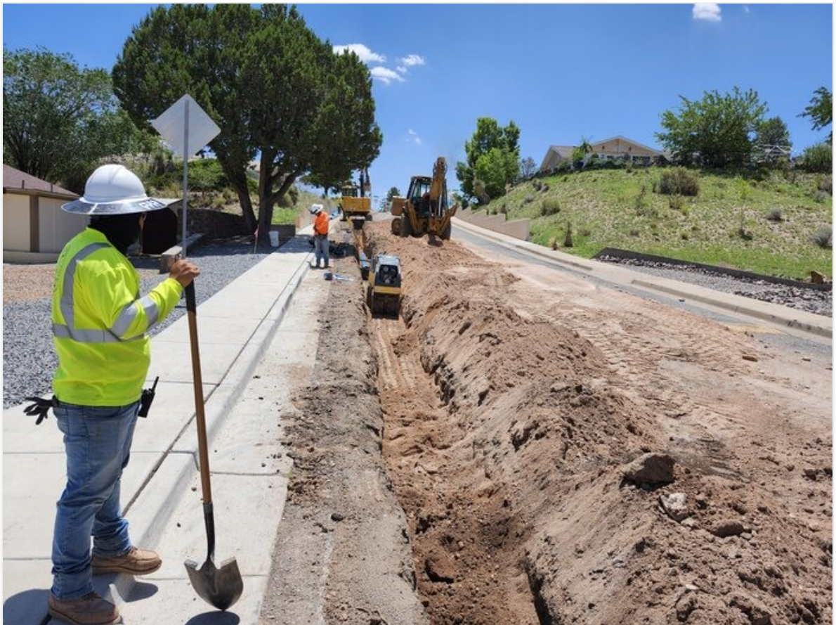
Compaction efforts on Chalcopyrite south.
