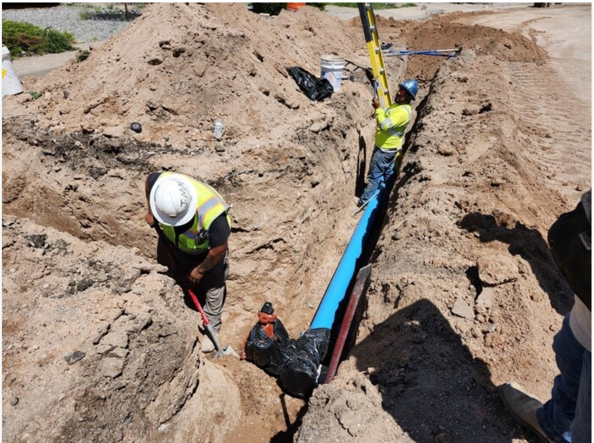
6" C-900 and GV for hydrant on Chalcopyrite Ave.
