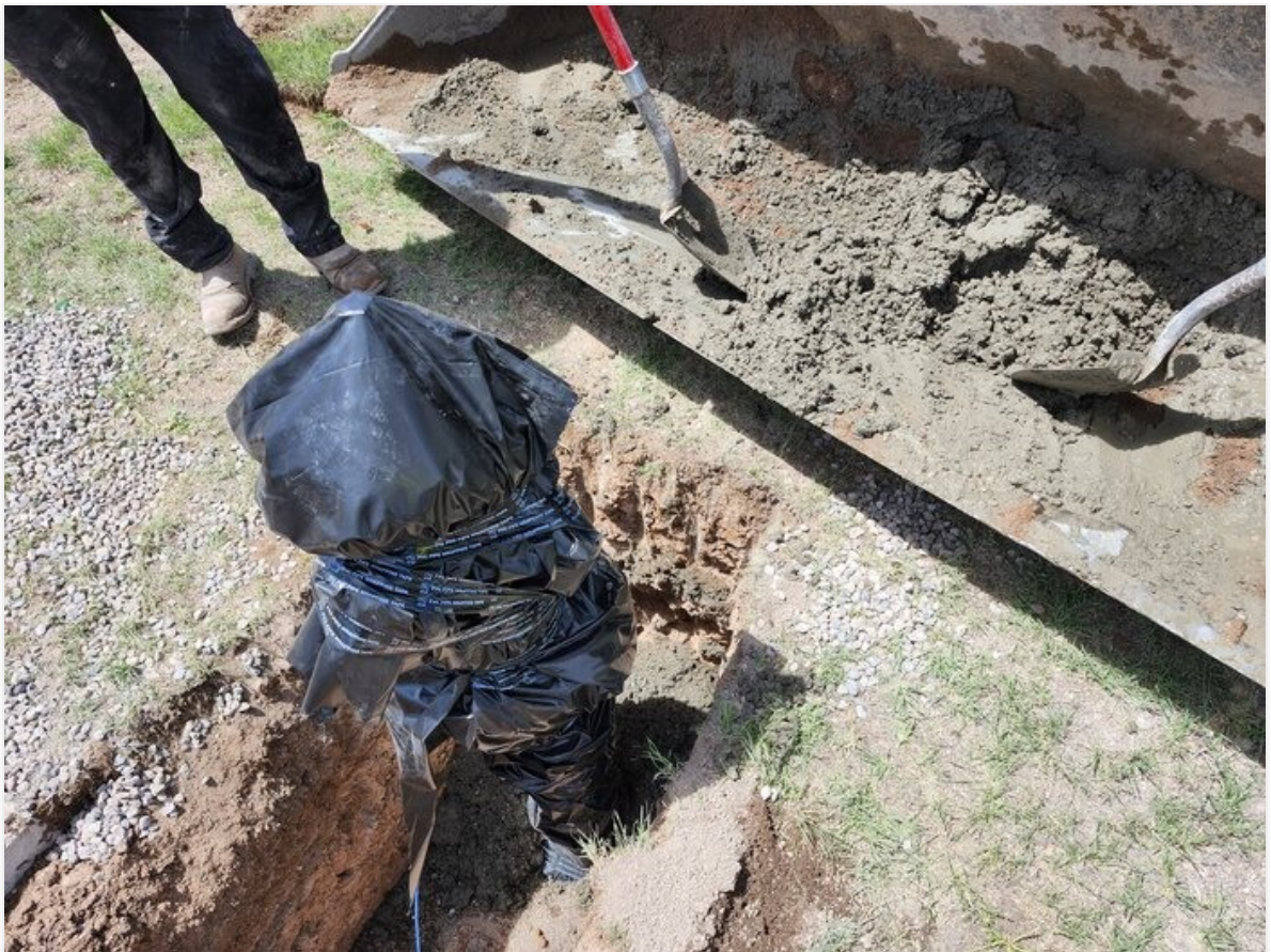
Concrete mixing and placement for thrust block on Toberite Ave.
