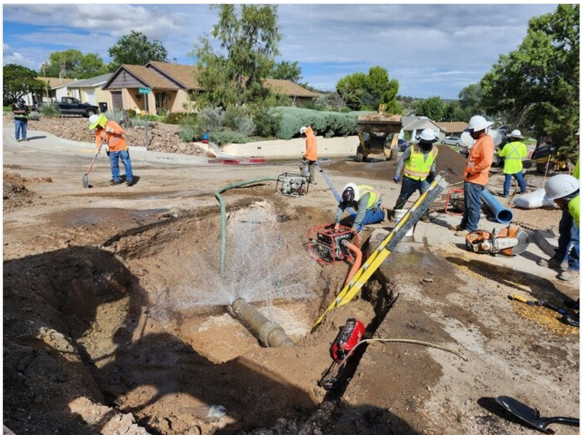
Saw cut existing ac water line to relieve pressure.
