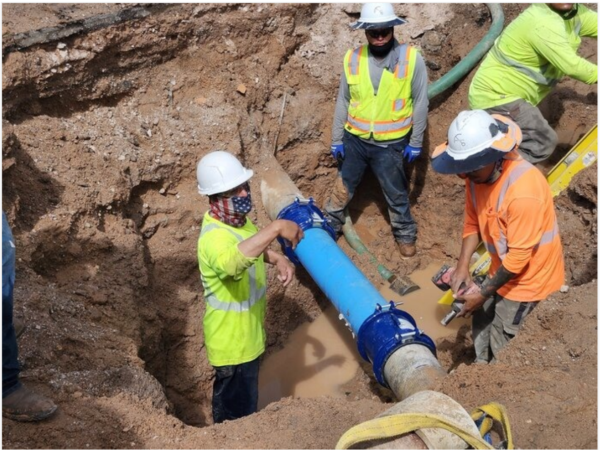
Repaired 8" AC line with 8" C-900 and two Hymac couplings.
