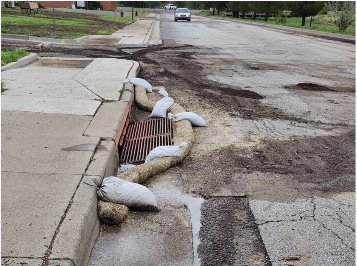
Smitcho replacing old wattles damaged to rain events.
