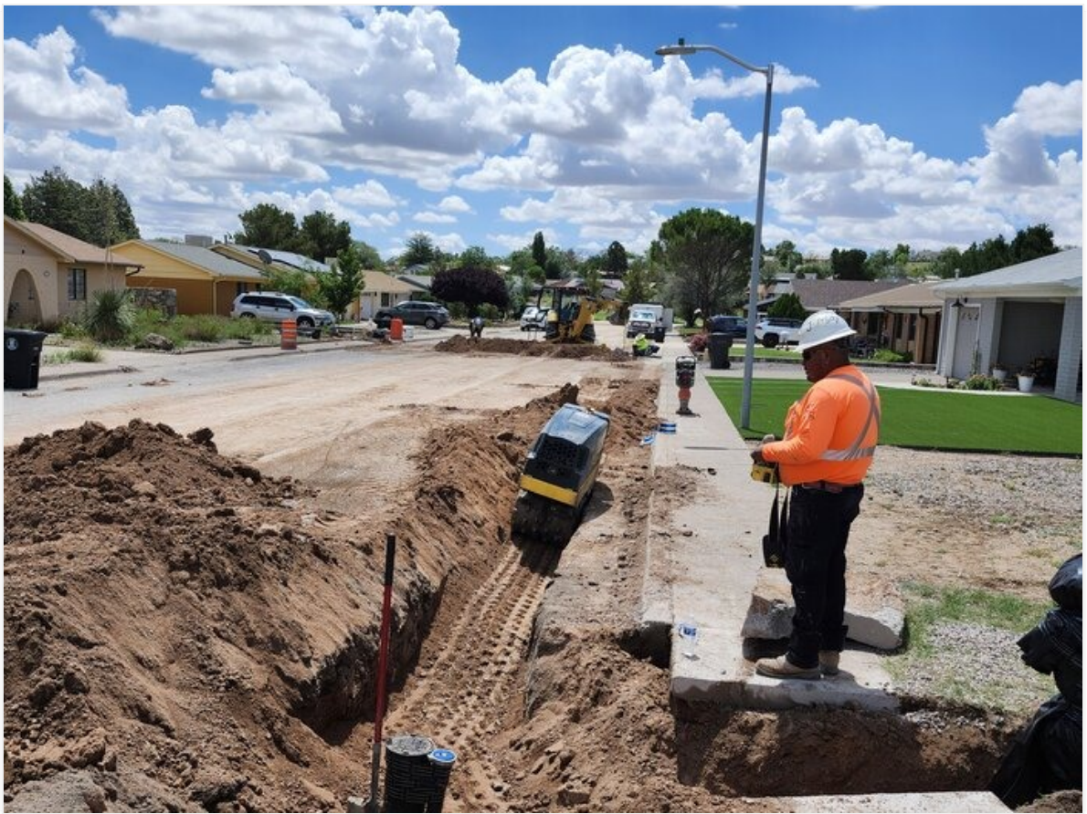
Compaction efforts on Tobernite Ave.
