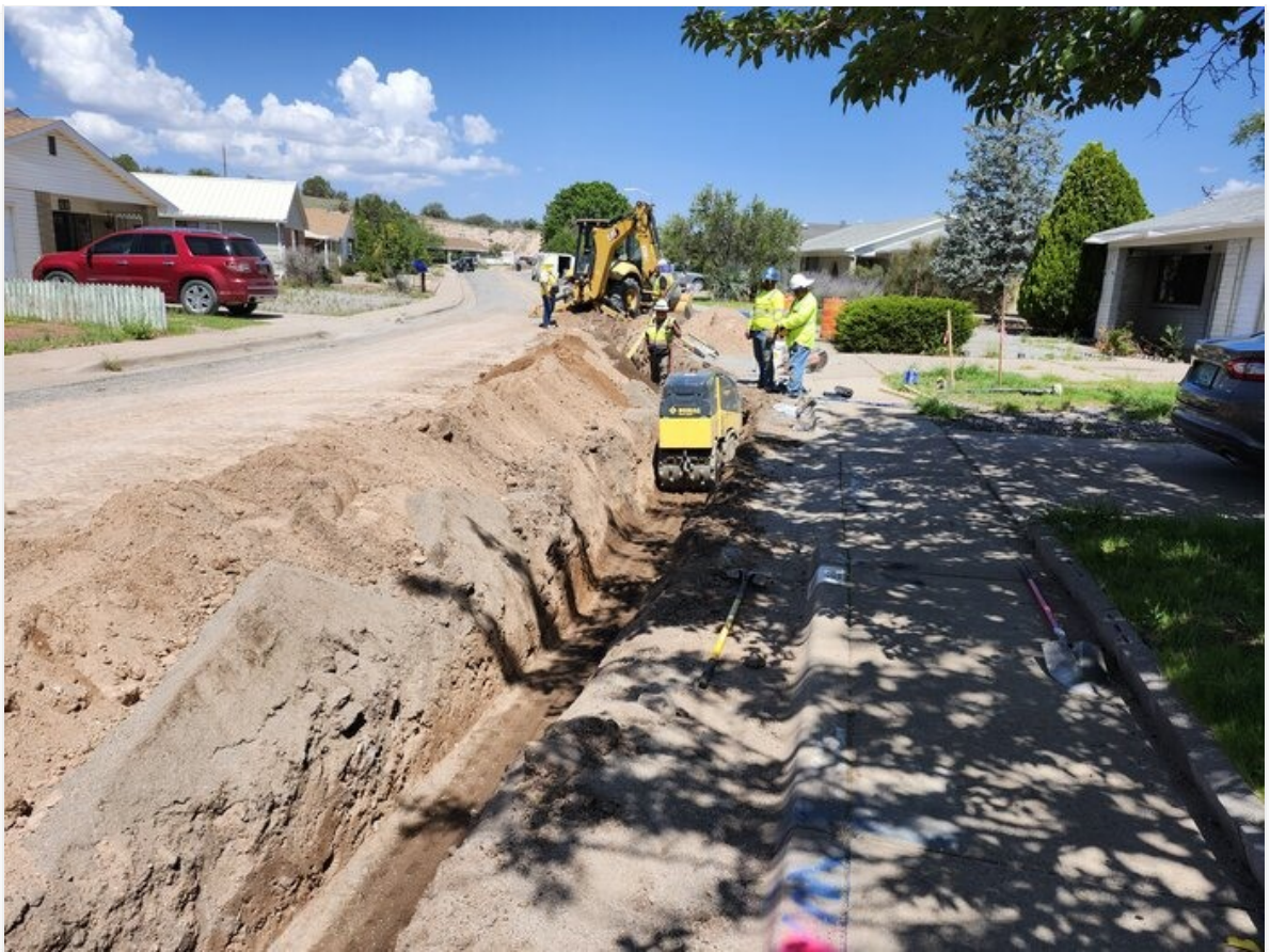
Backfill compaction efforts on Chalcopyrite Ave.
