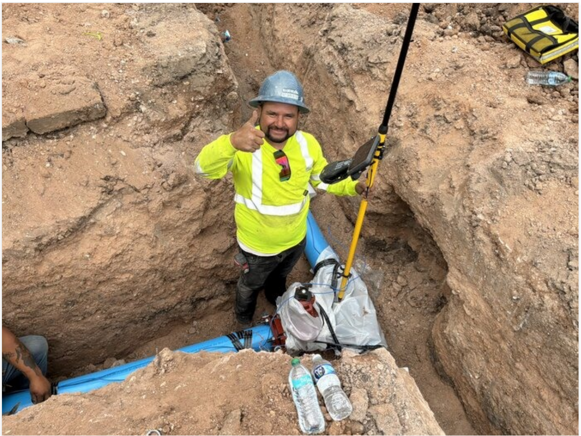
Survey as-built shot being taken for GV on Bornite St.
