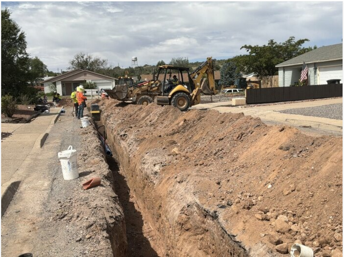
Backfill operations on Bornite St.
