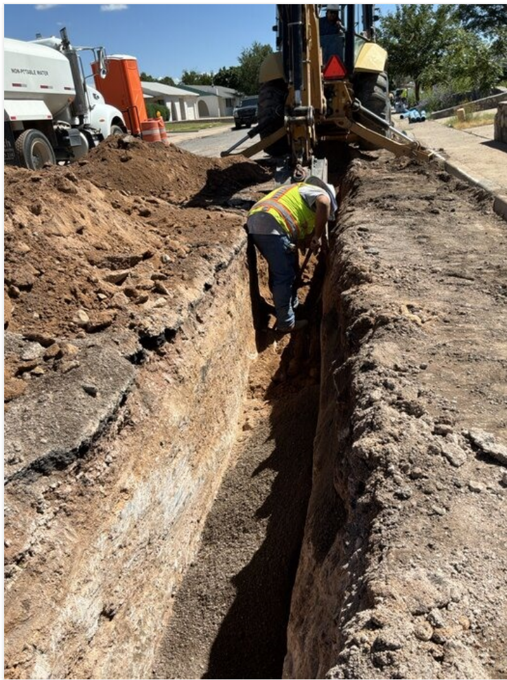
Excavation operations on Bornite St. for 6" C-900.
