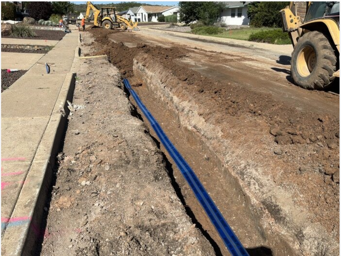
Caution tape being placed in trench as per plan.
