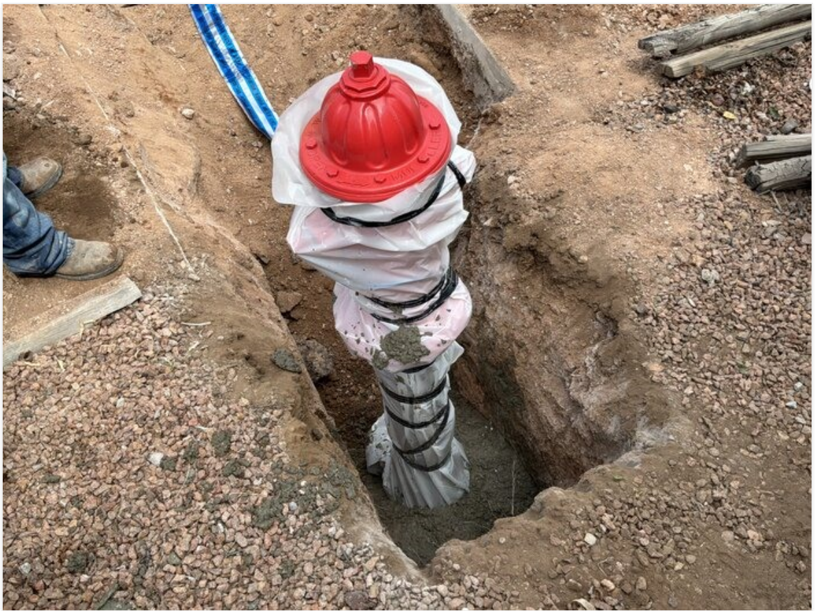
Fresh concrete thrust block for new fire hydrant on Bornite St.
