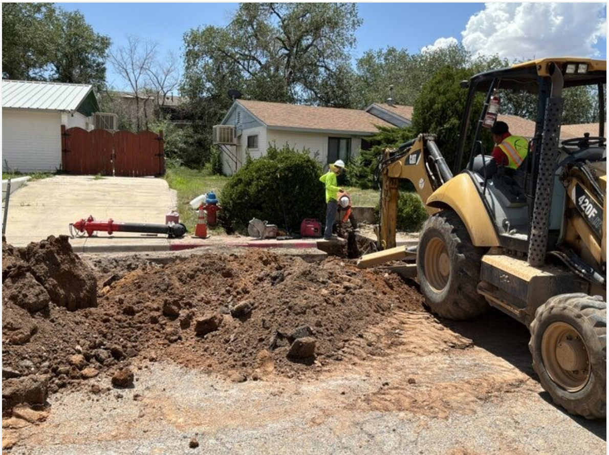
Excavating for new hydrant #49
