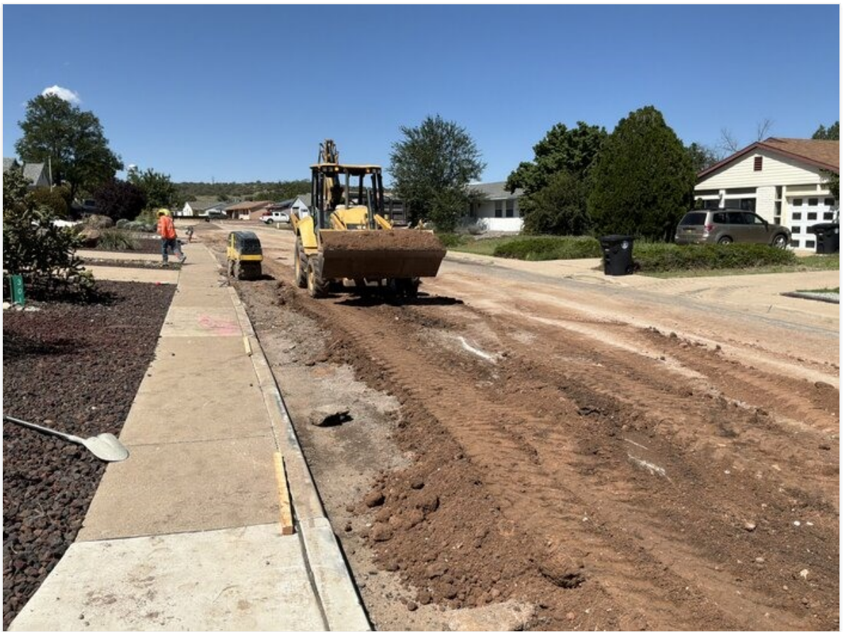
Wheel rolling finished subgrade for 6" C-900 trench on Bornite St.
