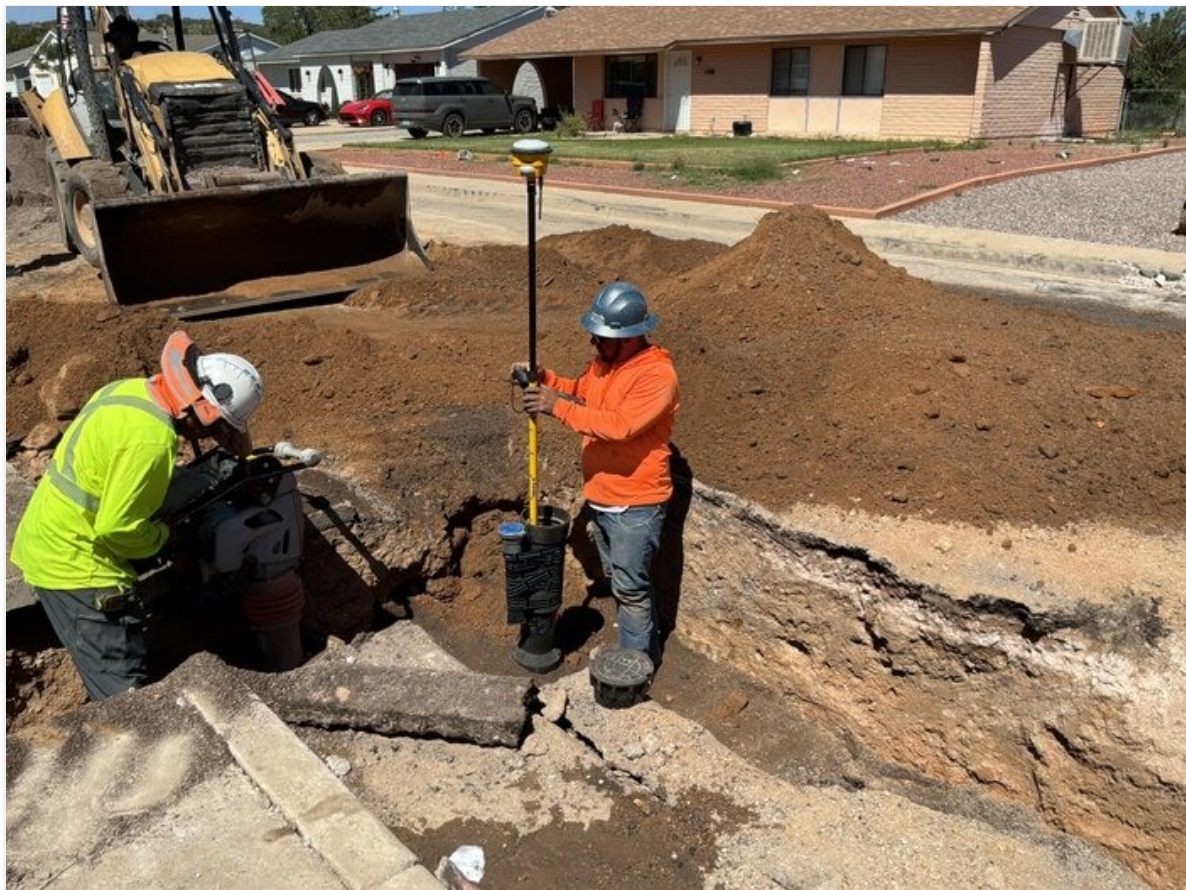
Survey as-built shot being taken on GV on Bornite St.
