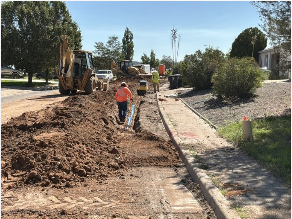
Caution tape being placed as per detail
