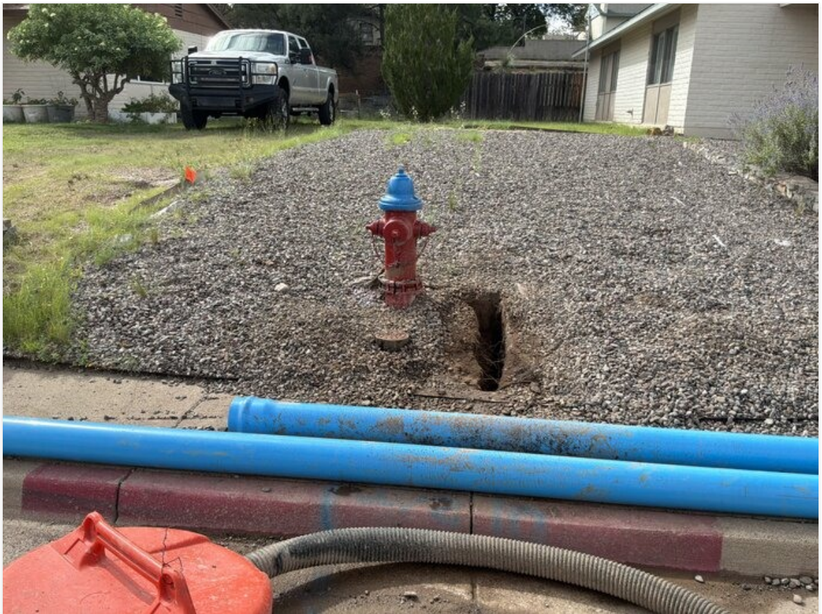
Potholing for existing utilities for new hydrant placement Bornite St.
