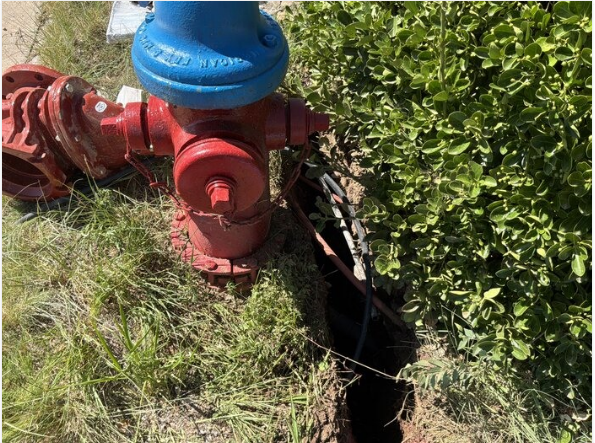
Communication lines next to existing hydrant #49.
