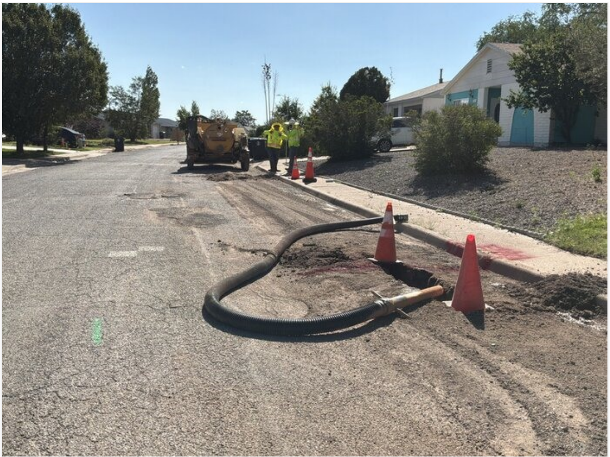
Potholing operations ahead of excavation on Bornite St.
