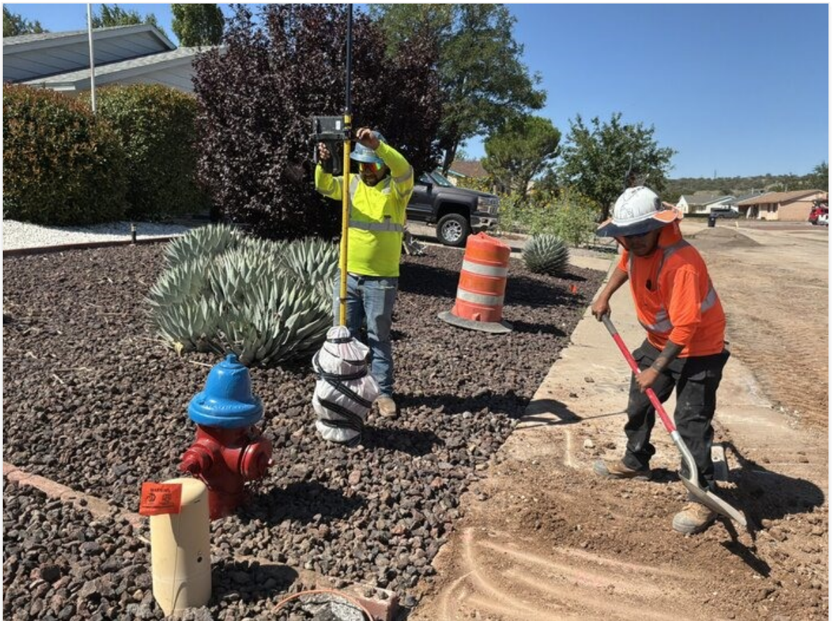
Survey as-built shoot on new hydrant on Bornite St.
