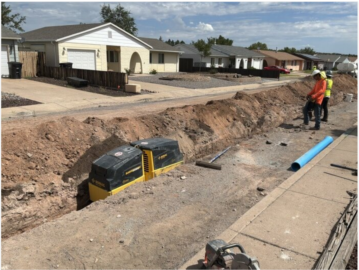
Compaction efforts on Bornite St.
