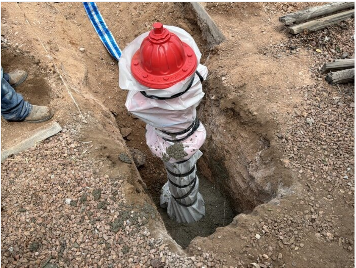
Fresh concrete thrust block for hydrant on Bornite St.
