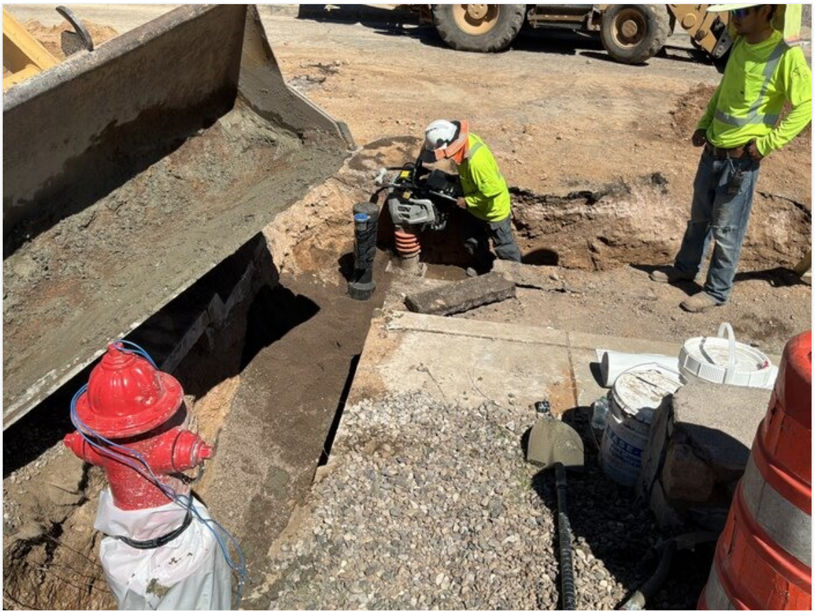
Compaction around GV for fire hydrant on Bornite St.
