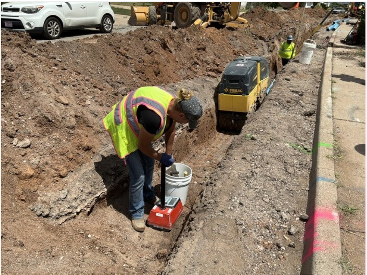
Backfill densities being taken.
