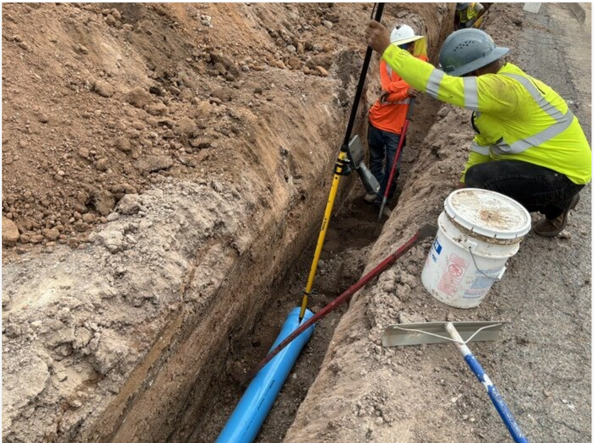
Survey as-built shot on 6" C-900 on Bornite St.
