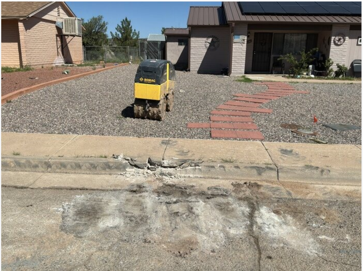
Fresh concrete thrust block for new fire hydrant on Bornite St.
