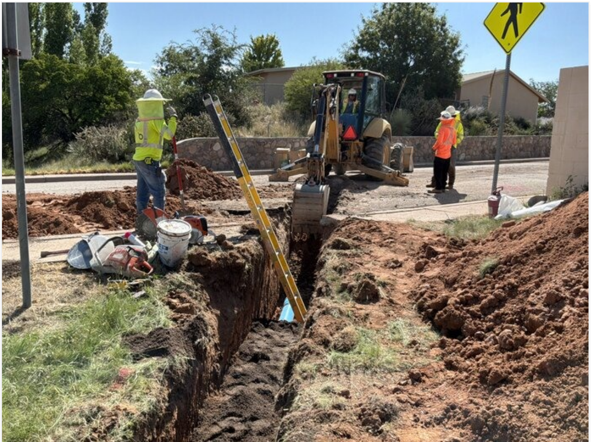
Excavating for 6" C-900 on Chrysocolla Ave.
