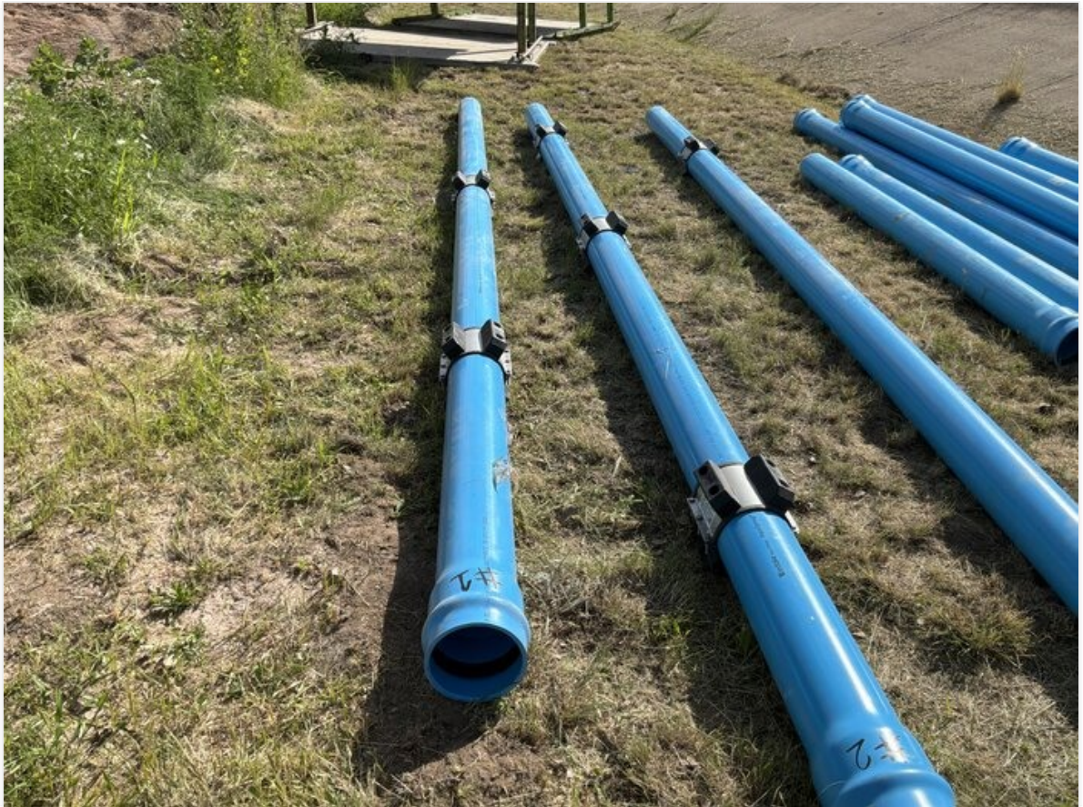
6" C-900 with pipe spacers as per pipe recommendation
