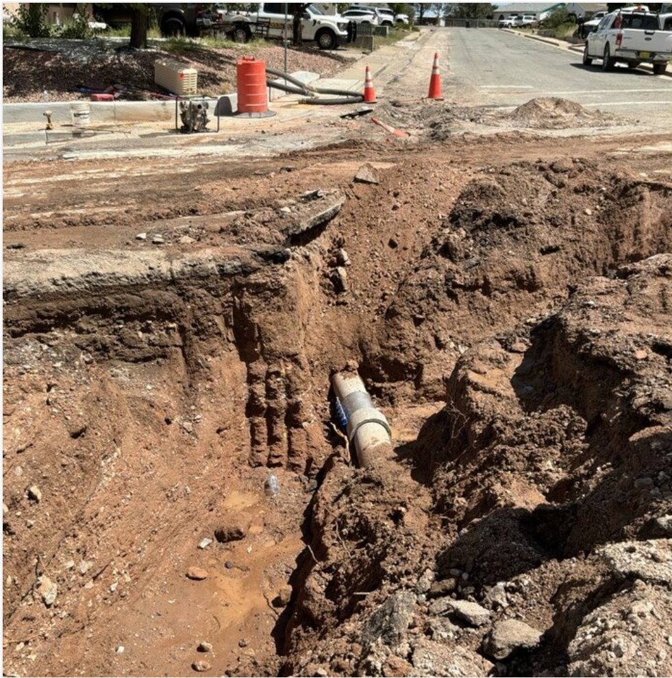
repair coupling on existing 8" AC line on Bornite st.
