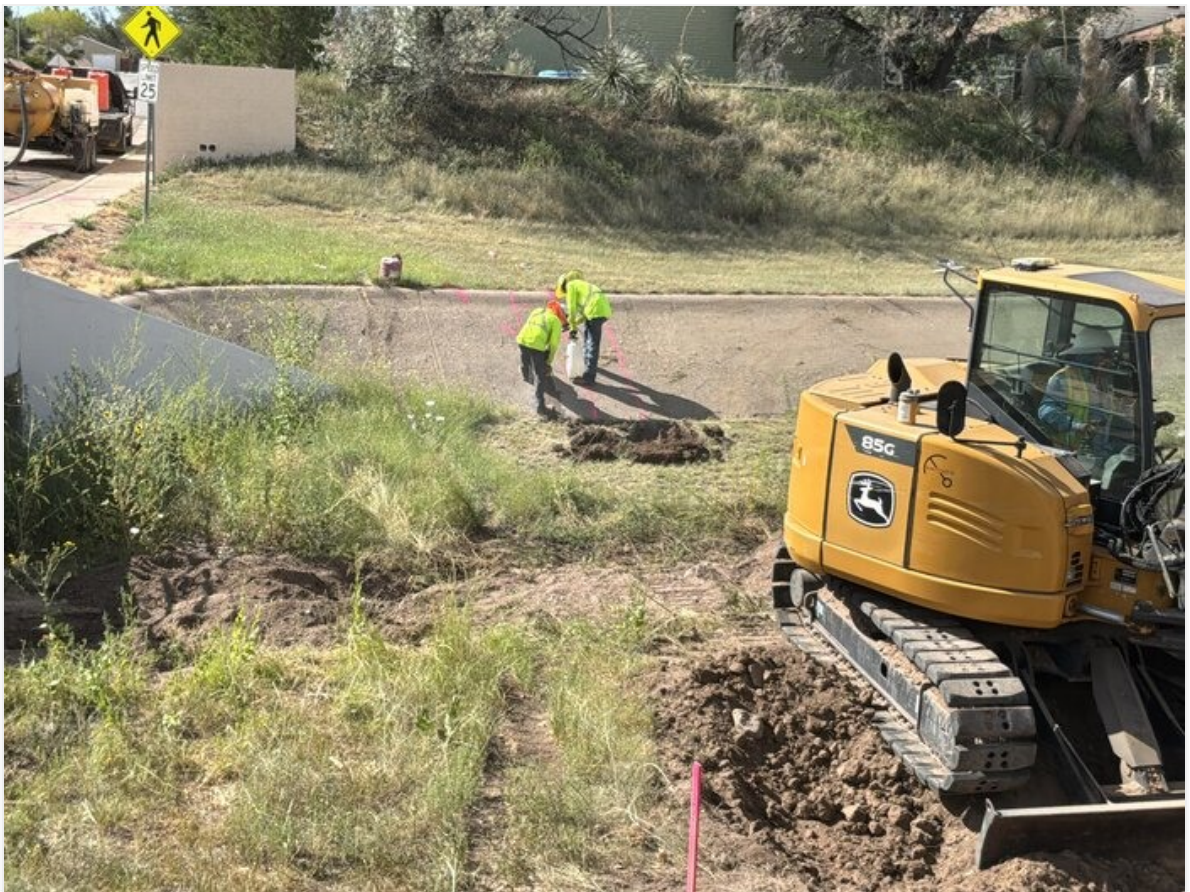
Saw cutting sloped concrete blanket at sta. 11+48
