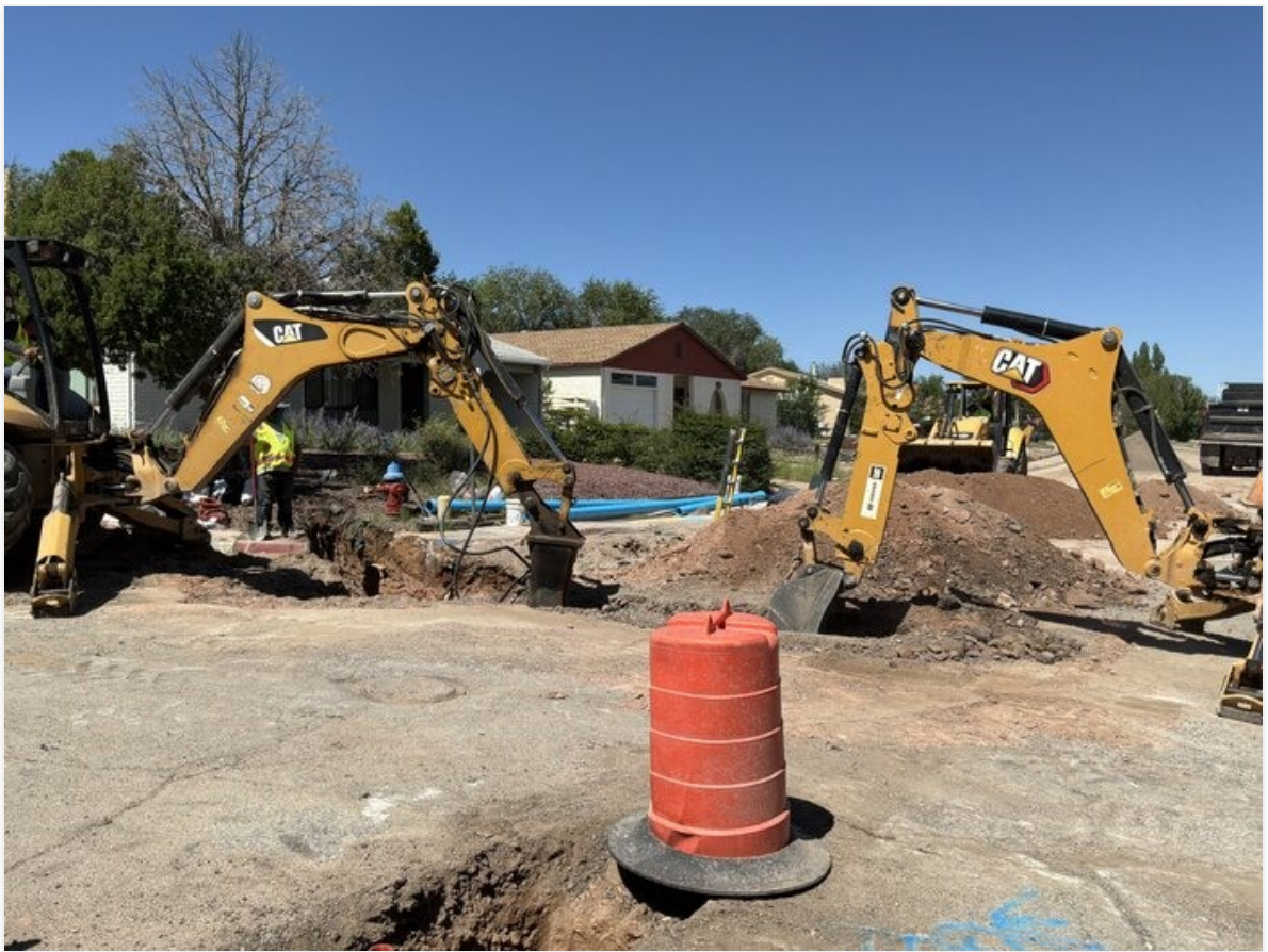
Hammer attachment and backhoe needed to excavate hard soil.
