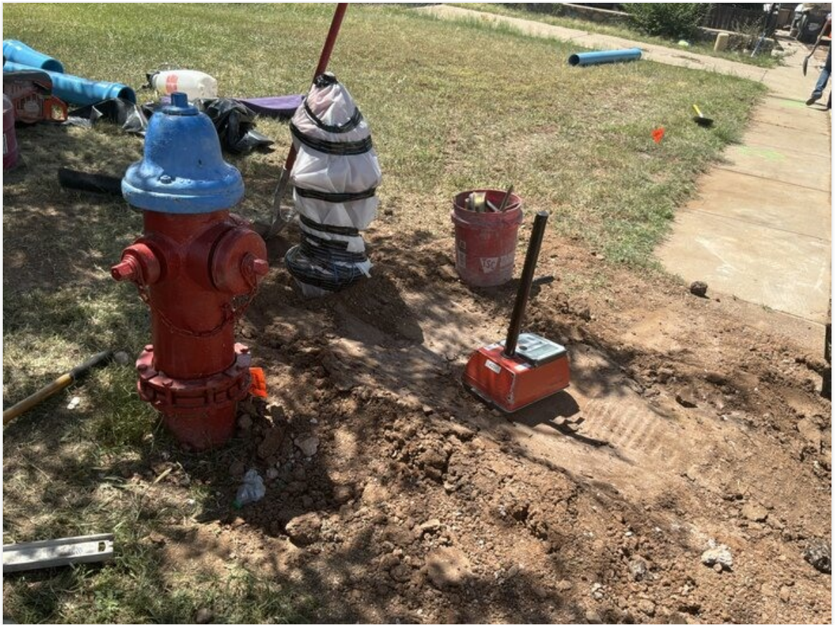
Fire line backfill density on Bornite St.
