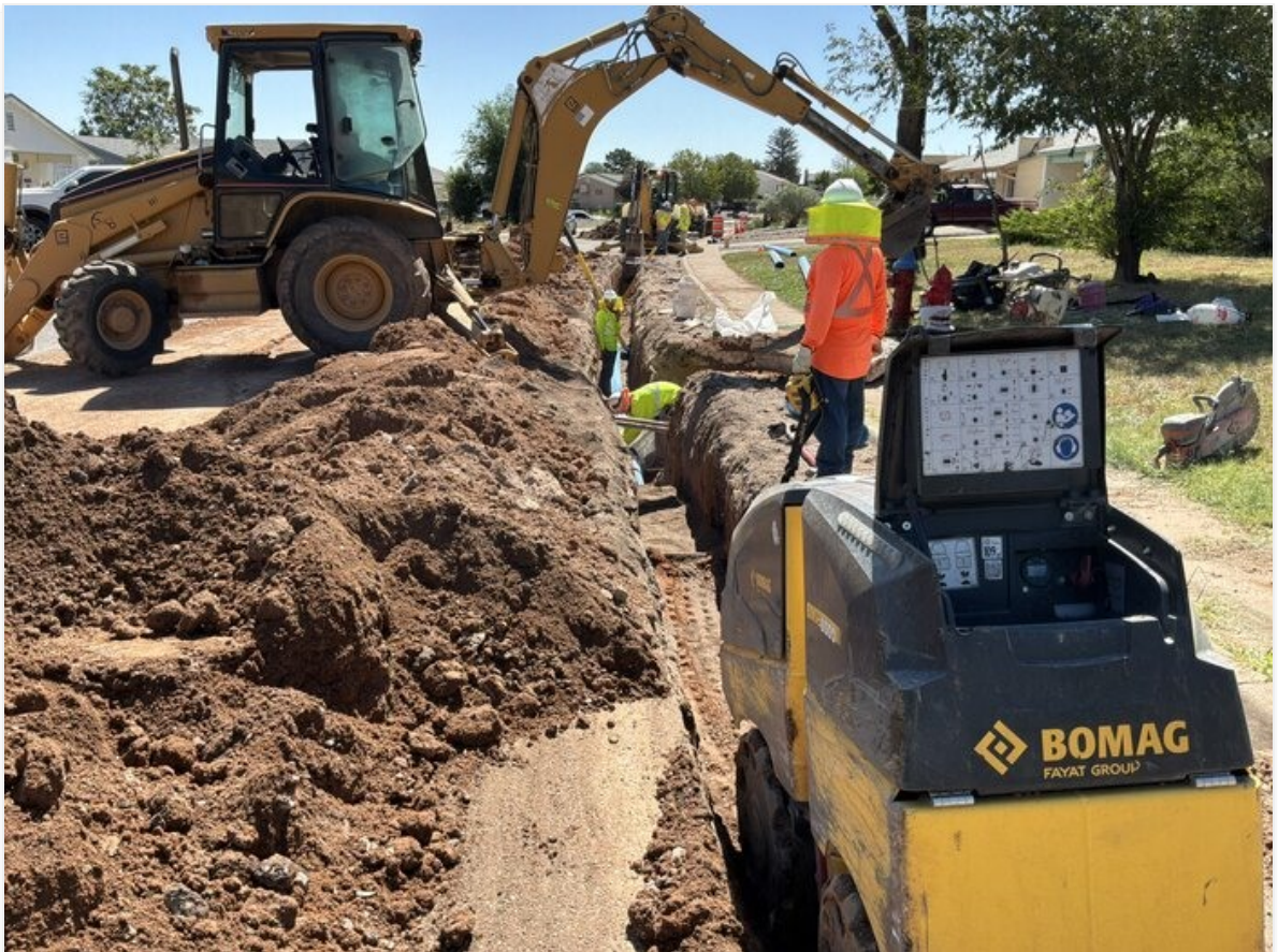
Compaction and hydrant placement on Bornite St.
