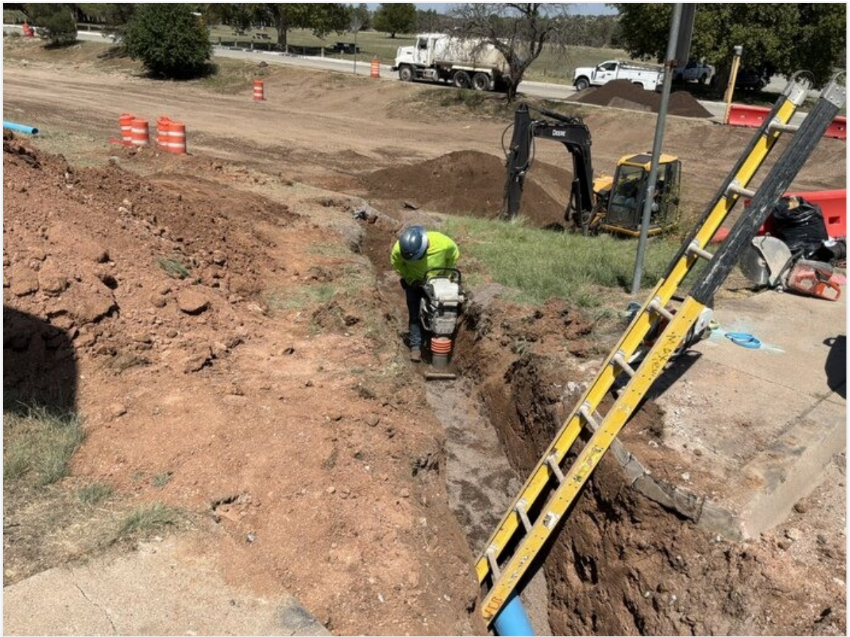
Compaction over 6" c-900, first lift.
