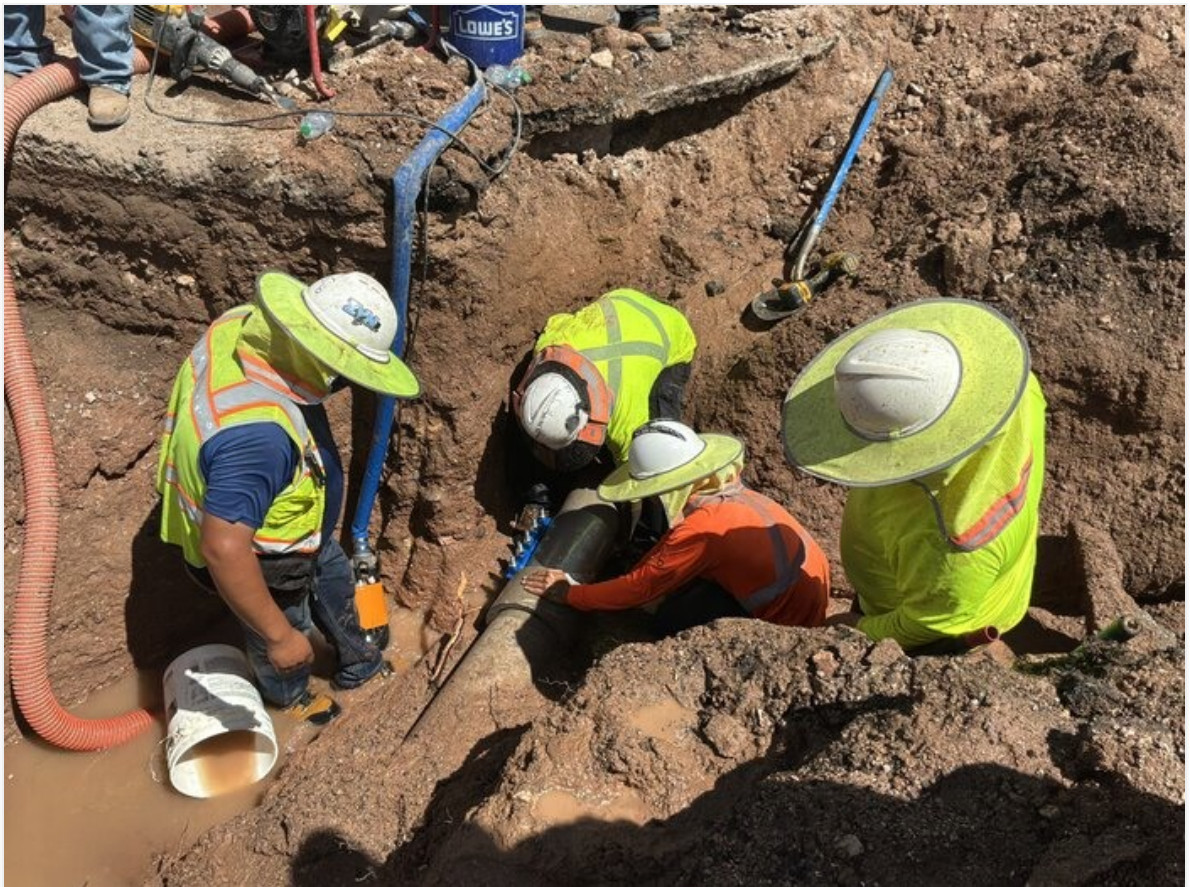
Installing repair coupling over 8" water line.
