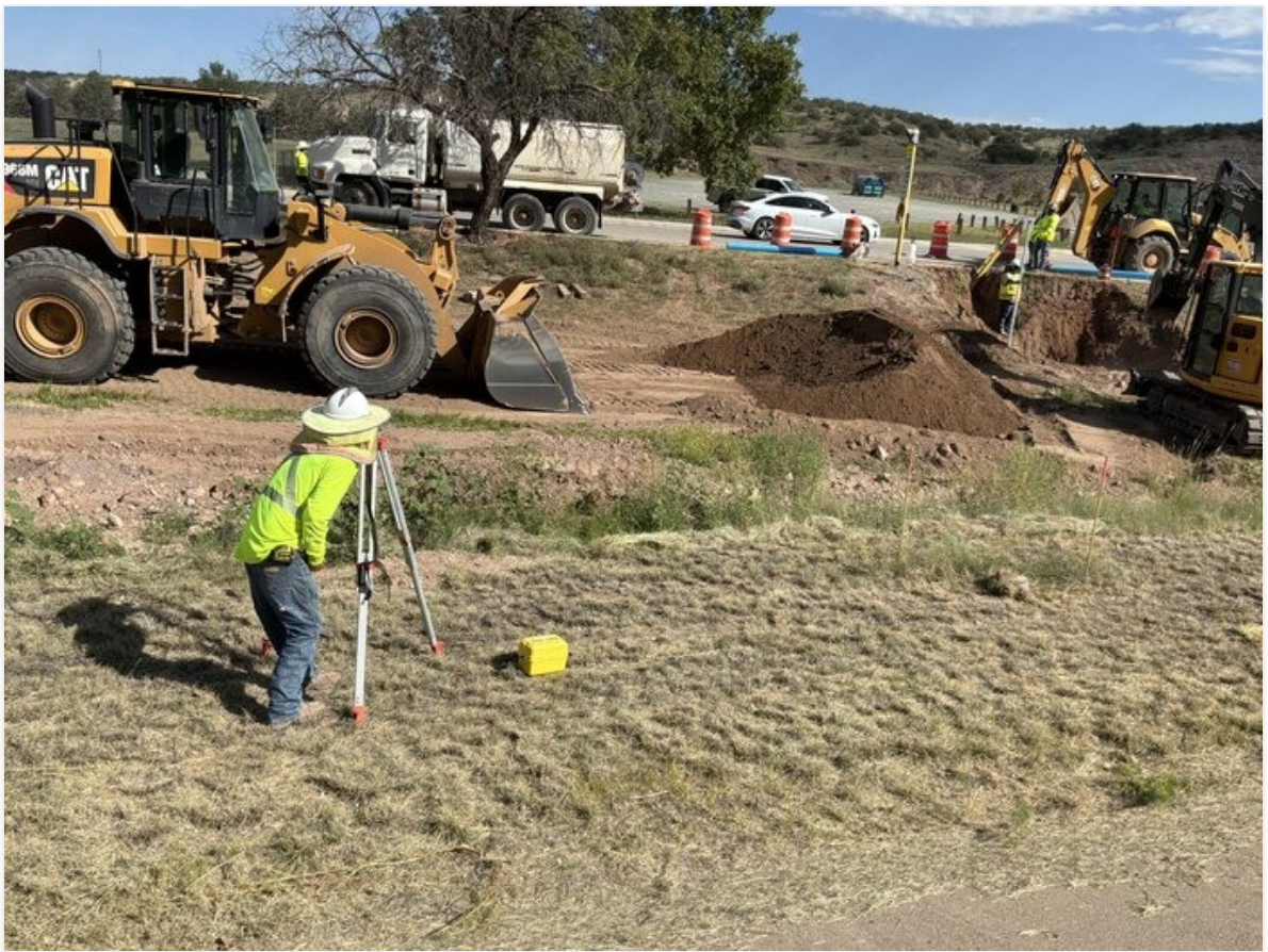
Taking elevation shots foe steel casing.
