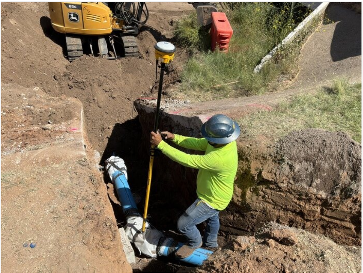
As-built survey shots on DI 45 fittings.
