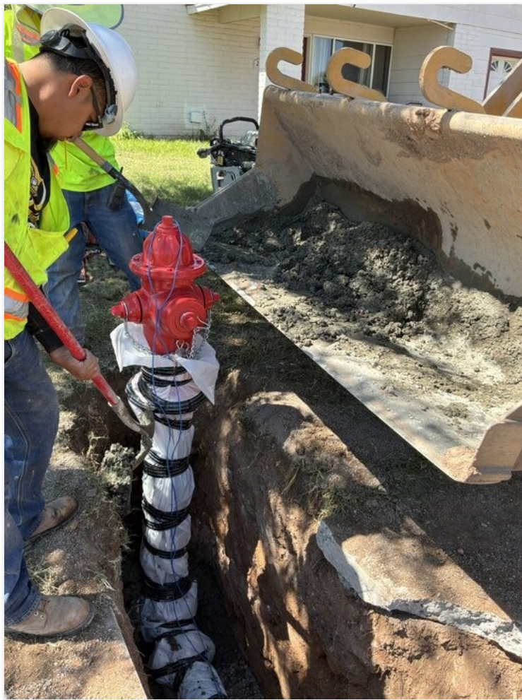
Placing fresh concrete for hydrant thrust block.
