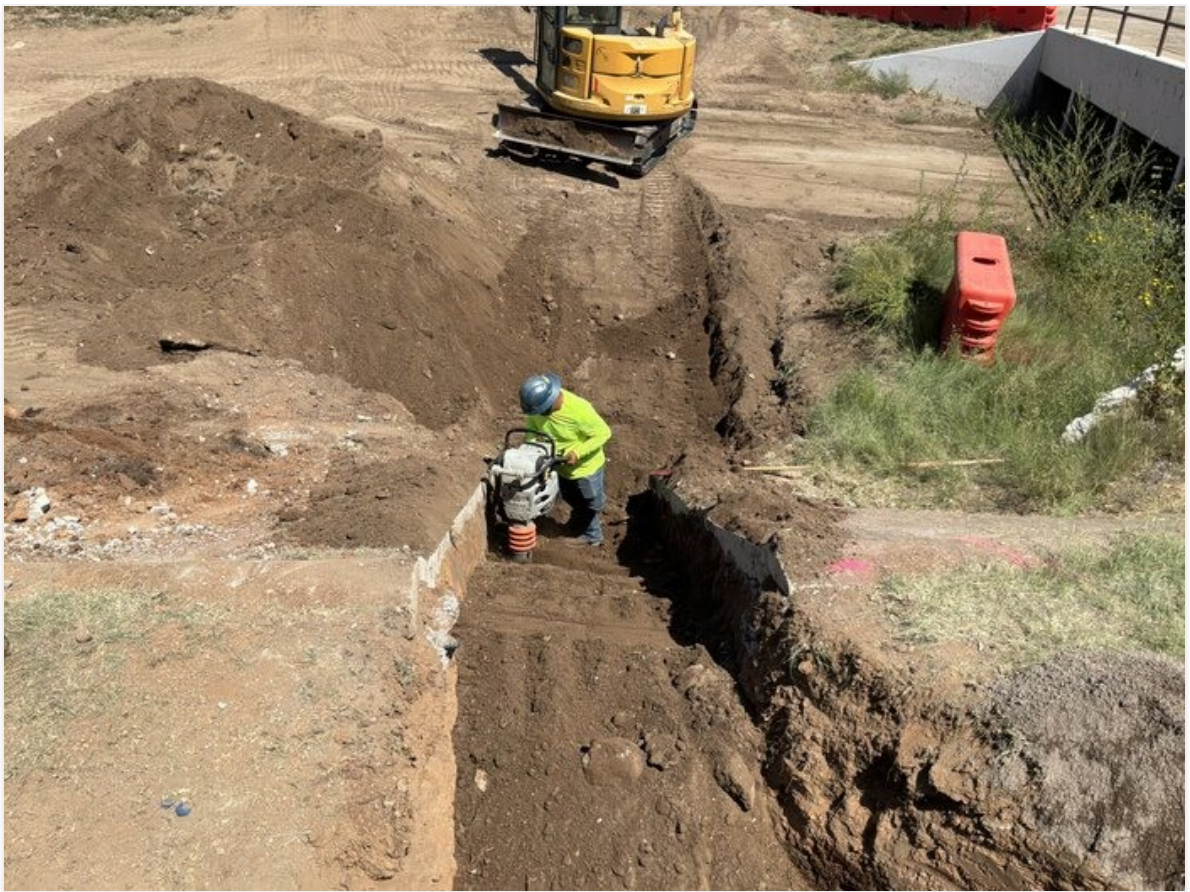
Compaction at removed sloped blanket at arroyo.
