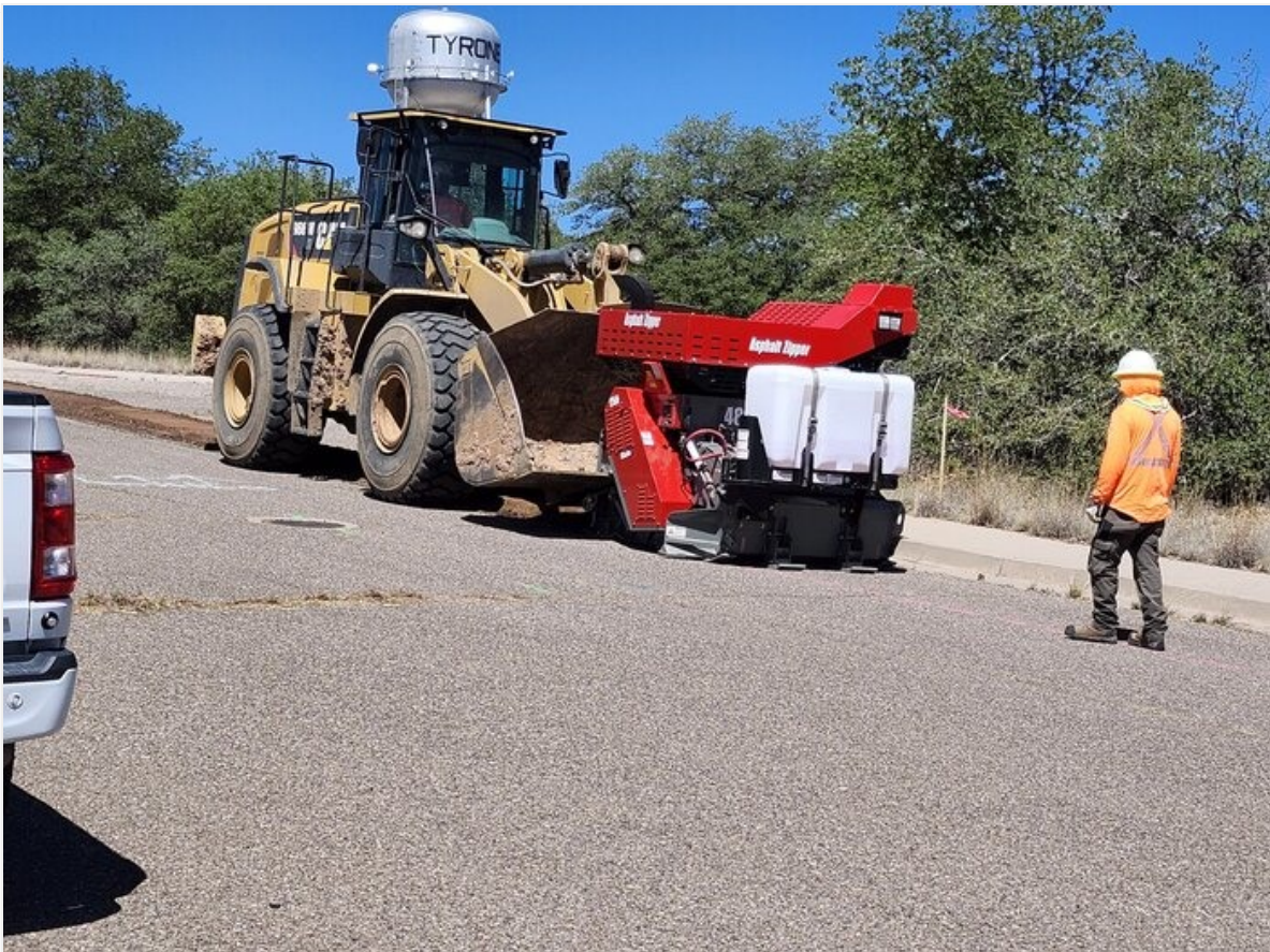
Milling 6' along Cooper Dr. for 12" pipe alignment.
