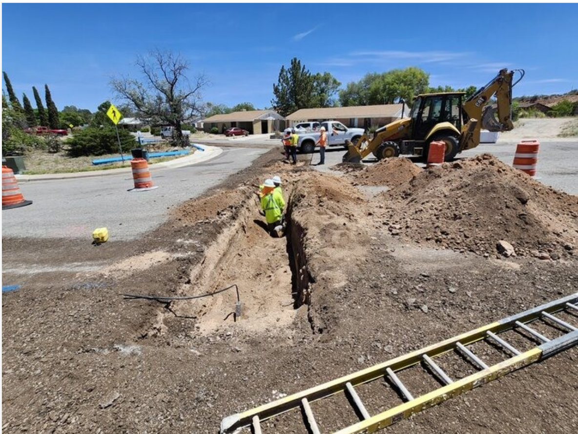
Potholing at Cuprite St. and Cooper Dr. for existing utilities.
