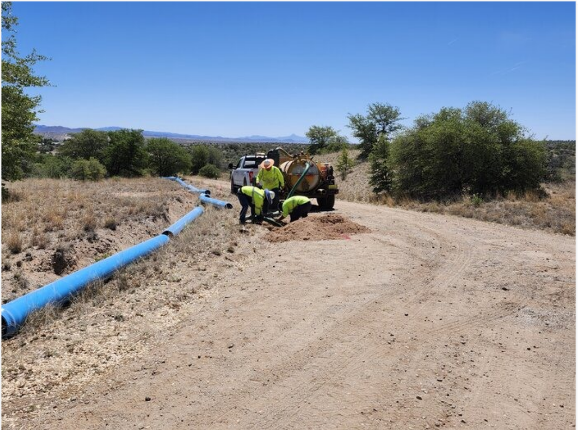
Potholing operations along Cooper Dr. (tank site)
