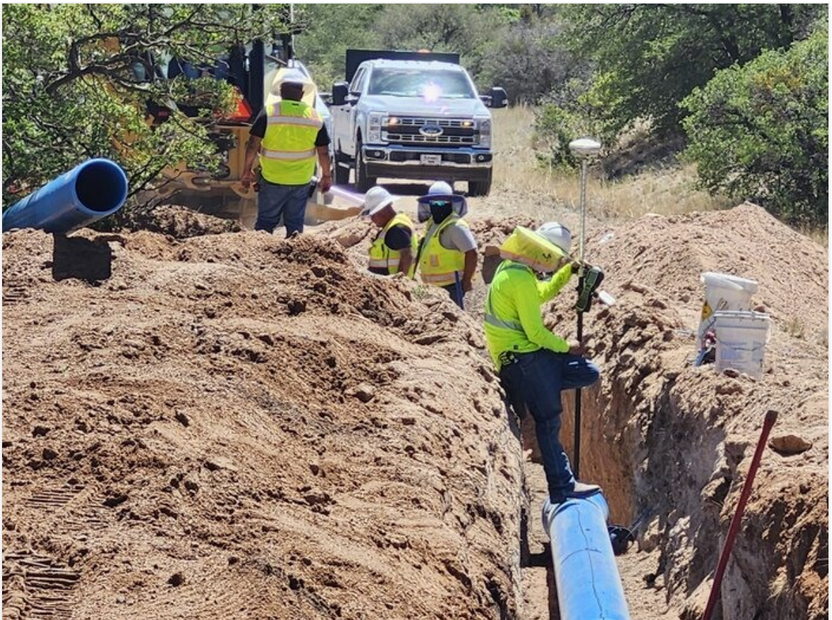
Survey as-built on 12" C-900.
