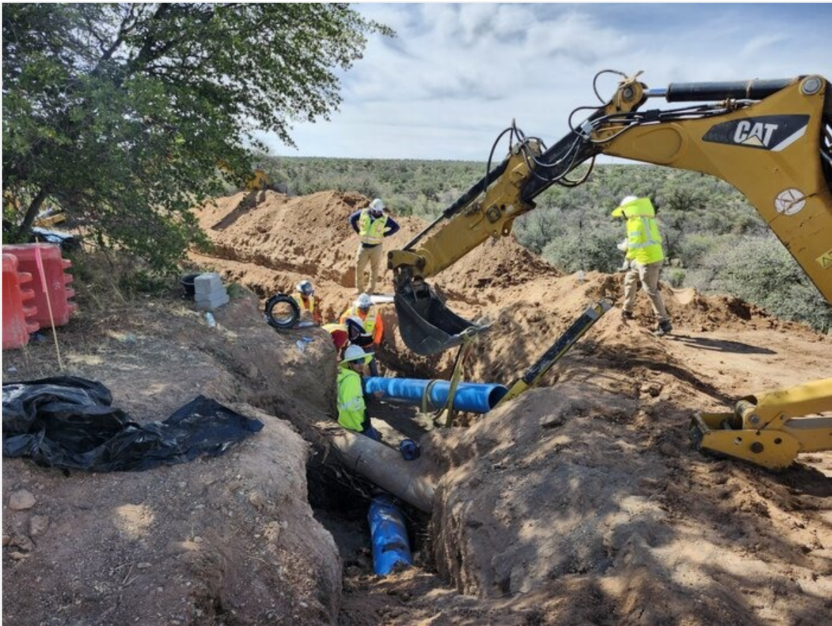
Placing new 12" C-900 under existing AC water line at approx. sta 11+00.
