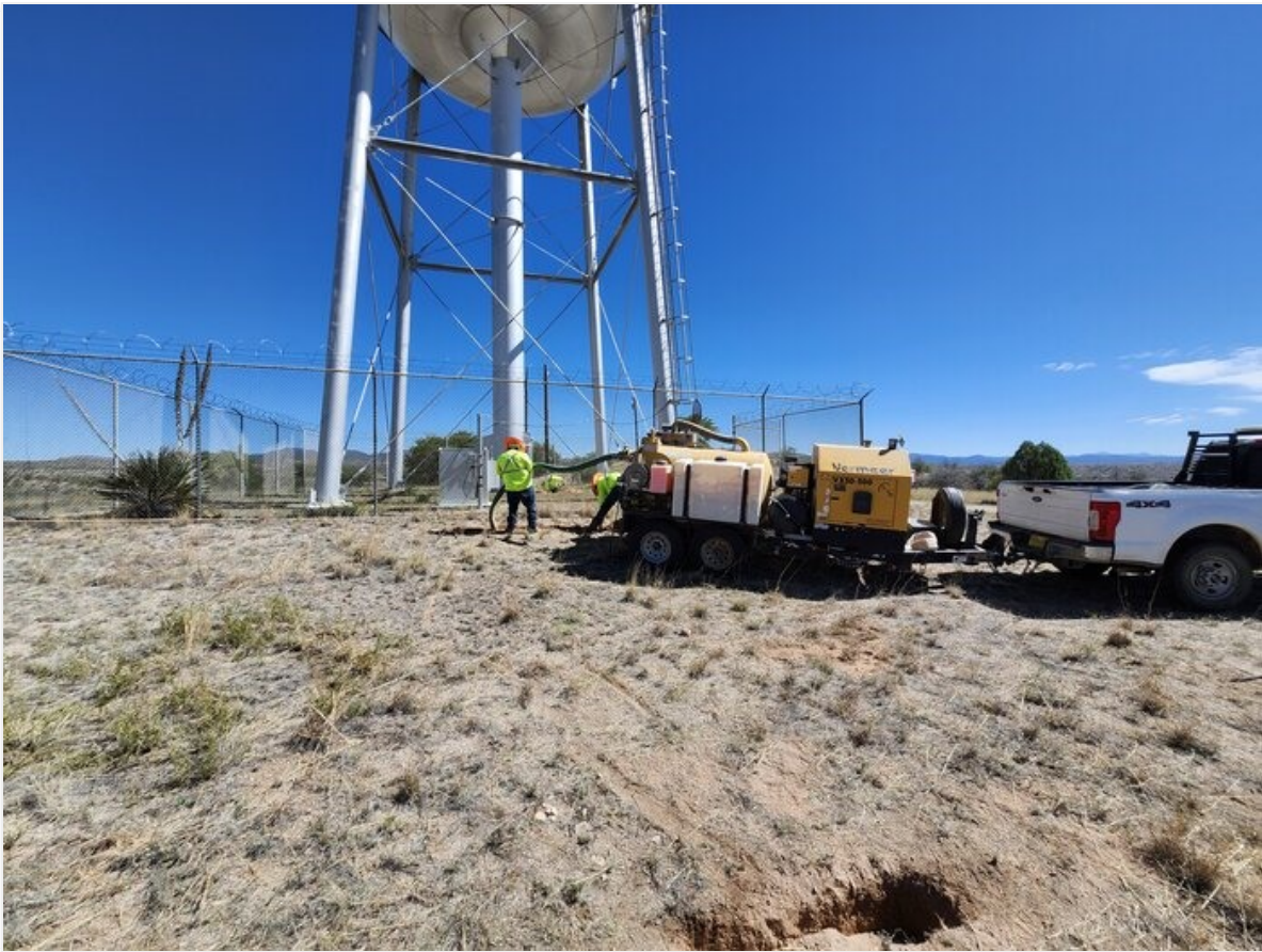
Potholing for exiting water line at tank site.
