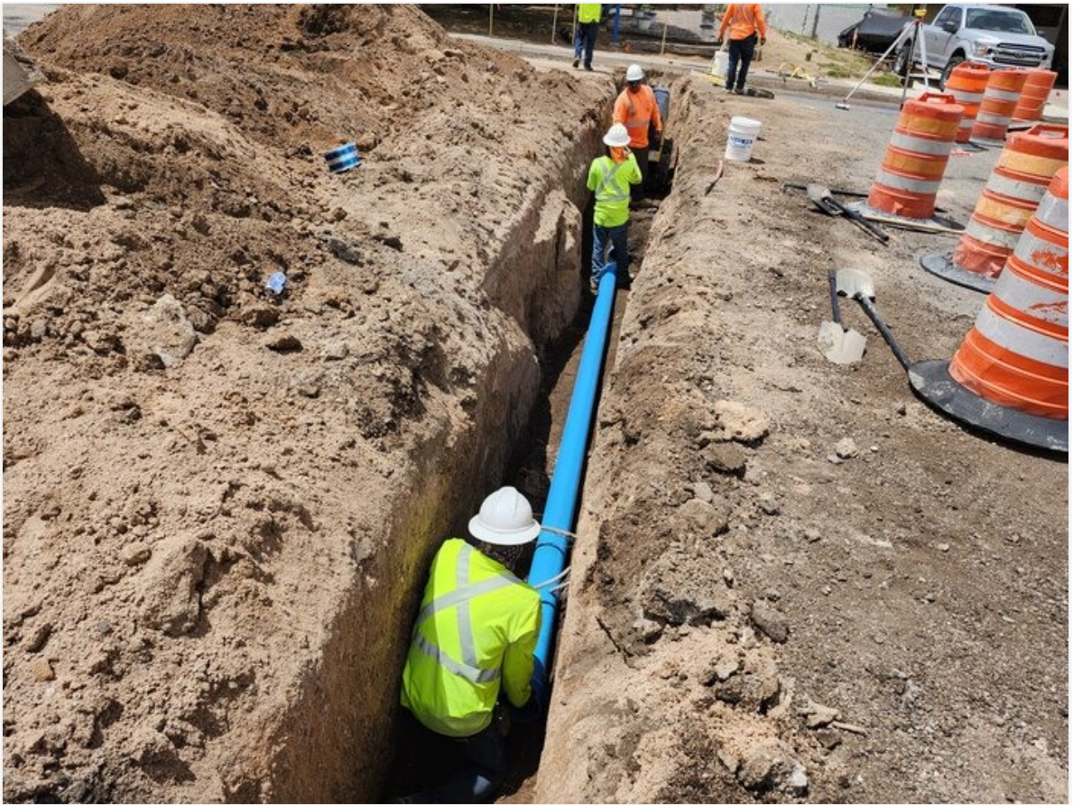
placing 6" C-900 across Cooper and Cuprite St.
