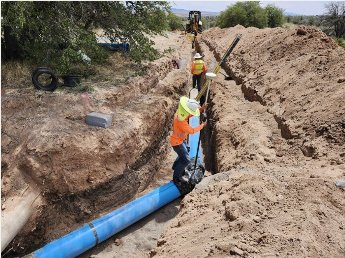
Smithco taking survey as-built shot on top of DI 45 bend.
