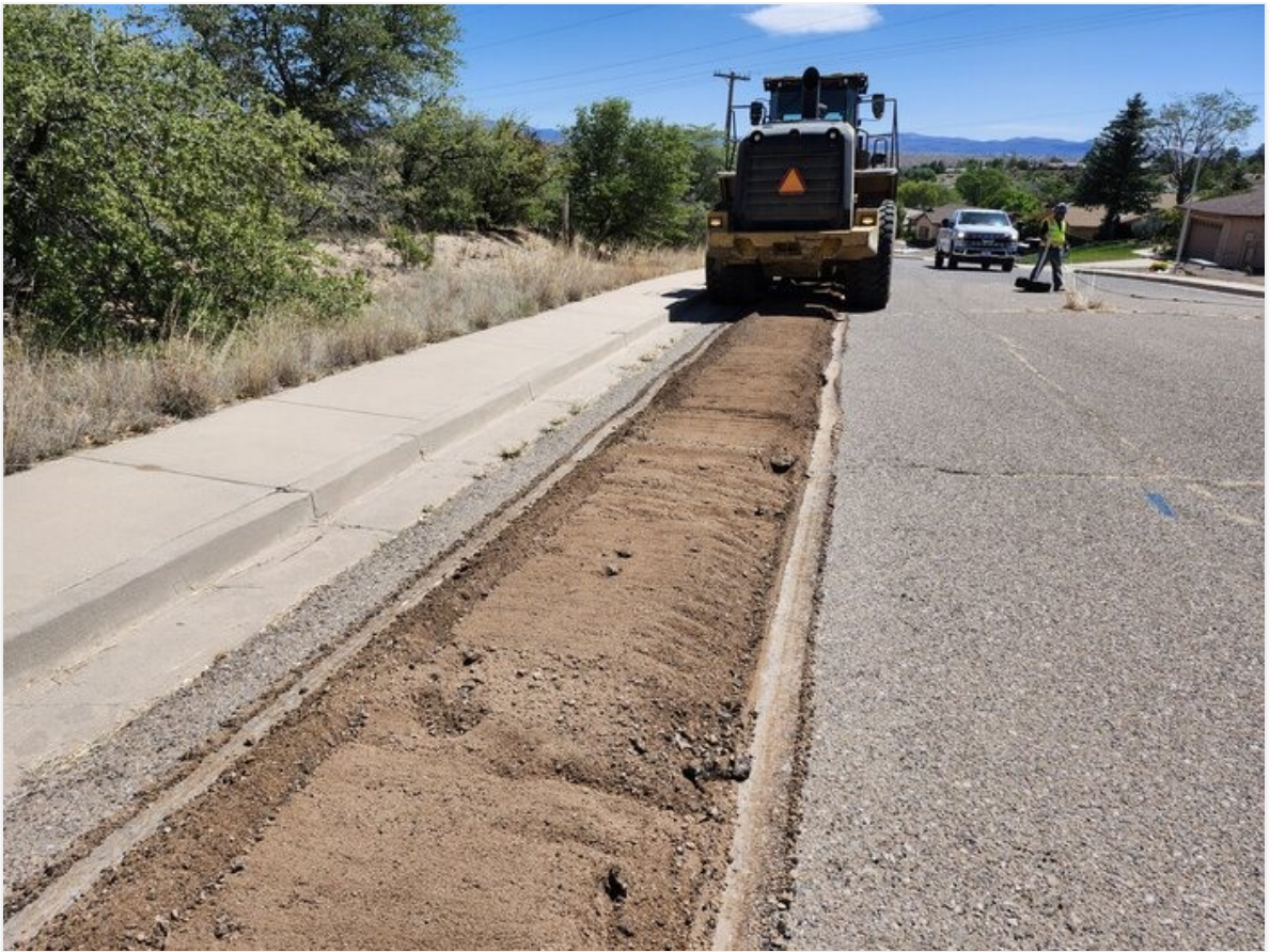
Milling 6' along Cooper Dr. for 12" pipe alignment.
