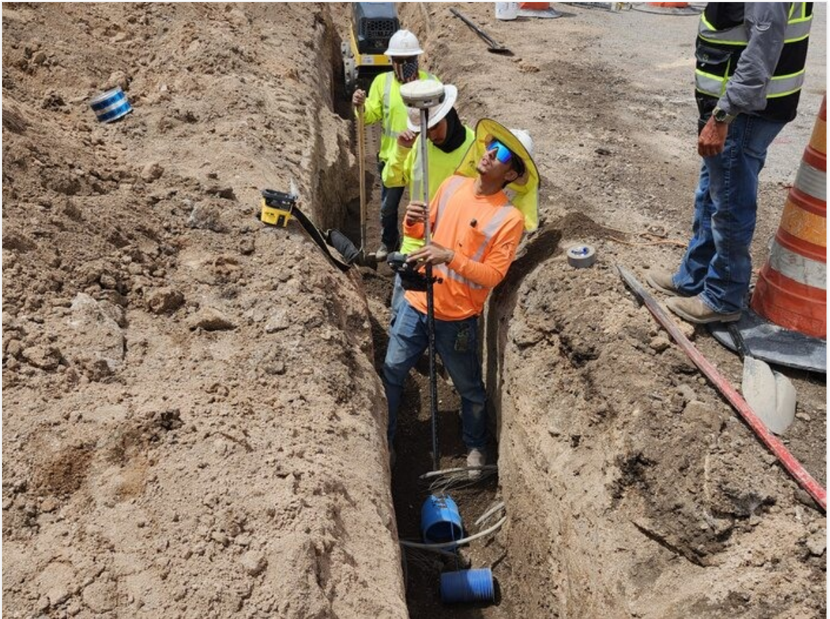
Top of pipe survey as-built shot on 6" C-900
