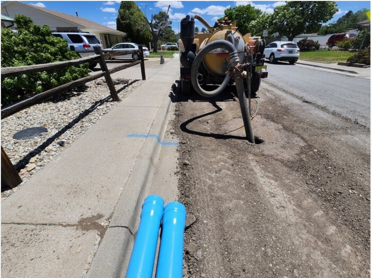
Potholing water services ahead of excavating on Cuprite St.
