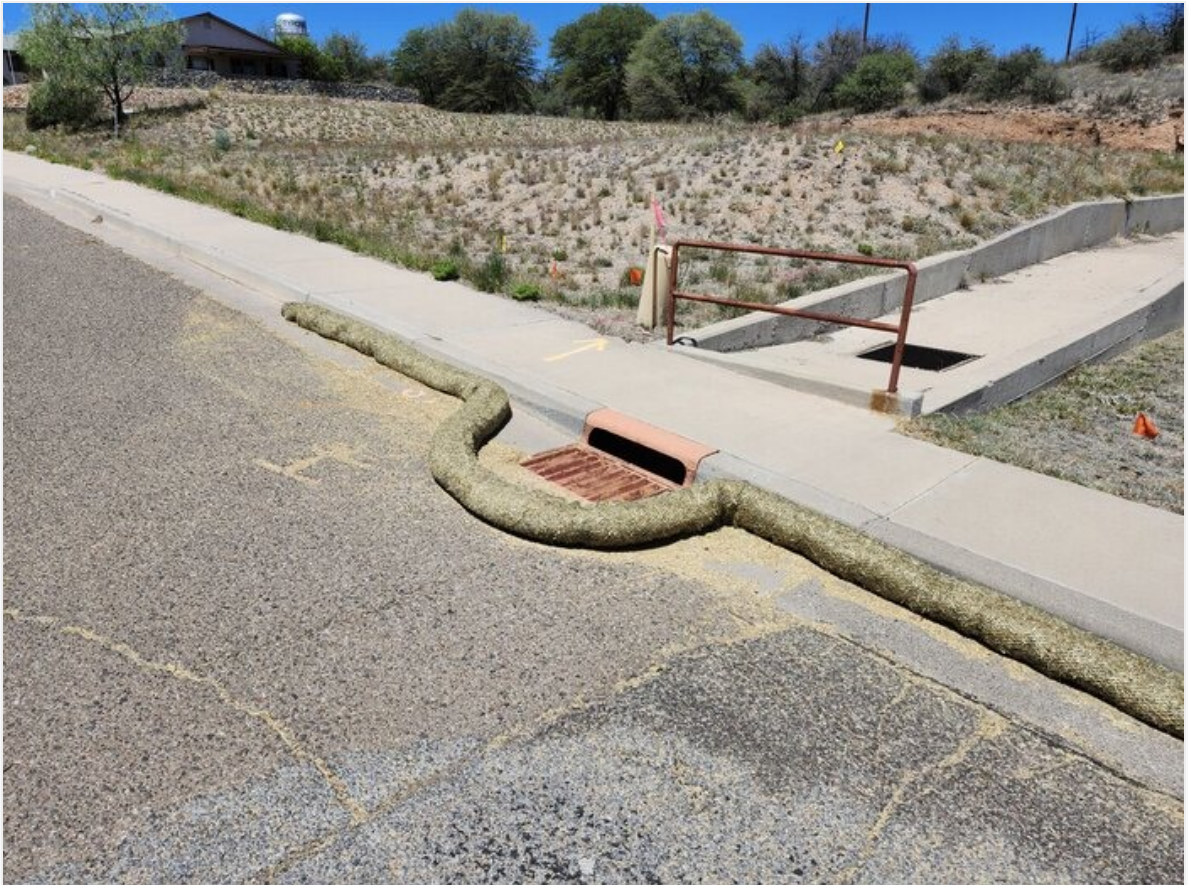
Implementing the SWPPP with BMP along Cooper Dr.
