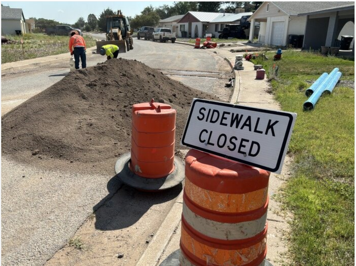
Sidewalk closed sign for pedestrian safety.
