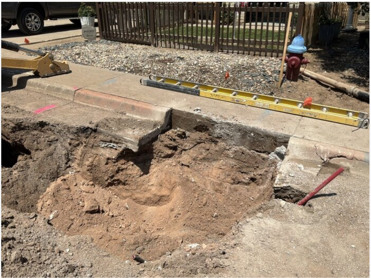
Excavation for GV on Cooper Dr. sta 25+55
