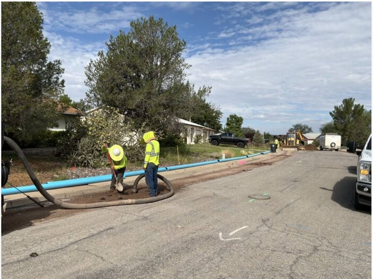
Potholing for existing utilities ahead of excavation on Chalcocite St.
