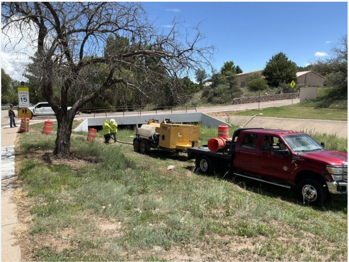
Potholing for power line in arroyo.
