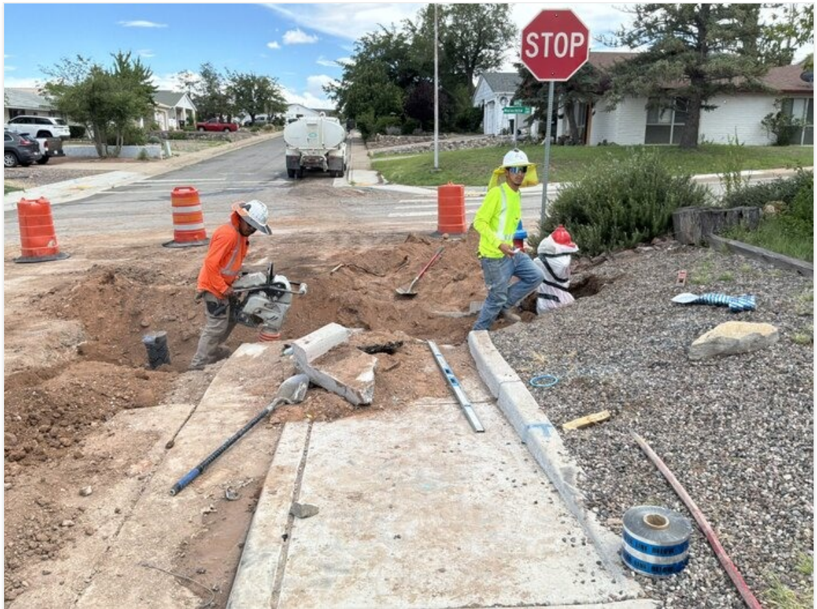
Compaction of hydrant fire line on Chalcocite St.
