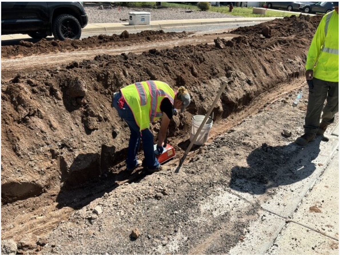
Summit Lab taking backfill densities.
