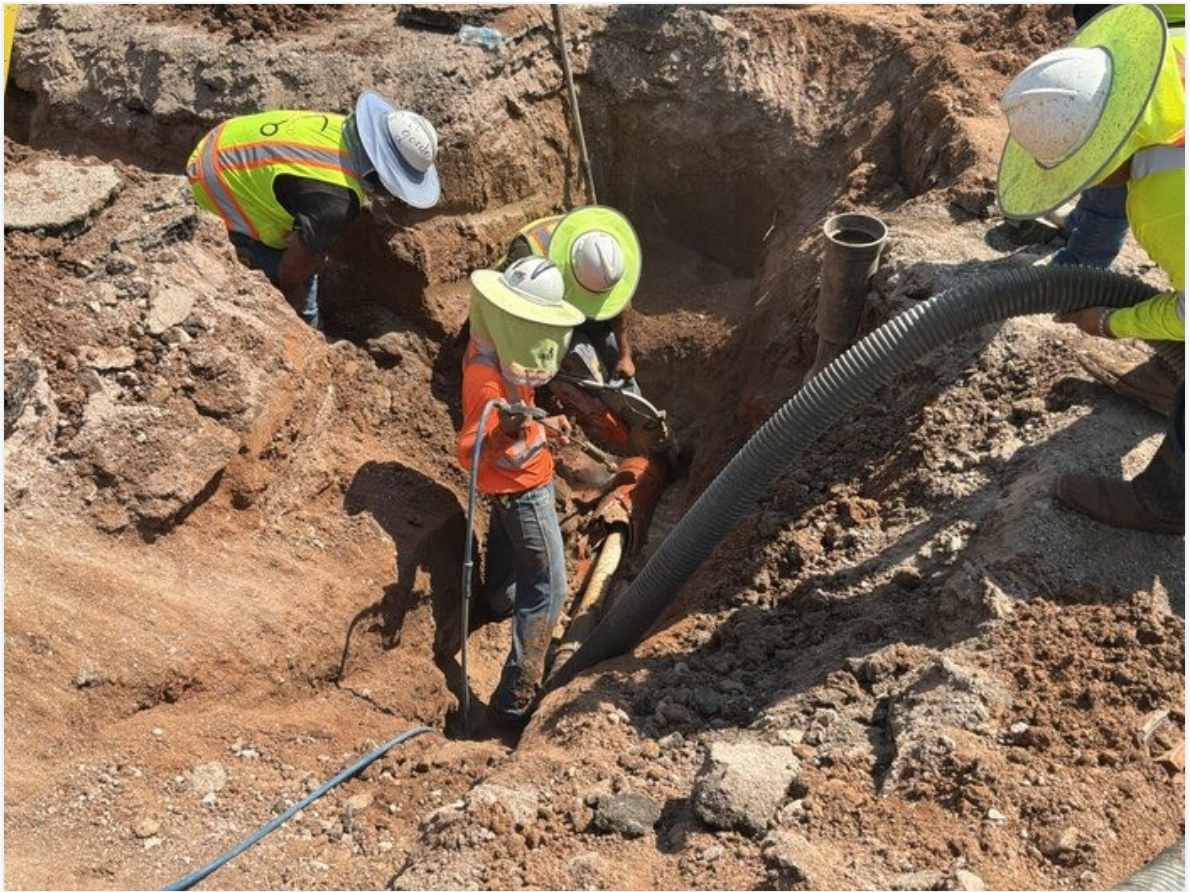
Vacuum the sewer sludge on cuprite St. at sta 29+17
