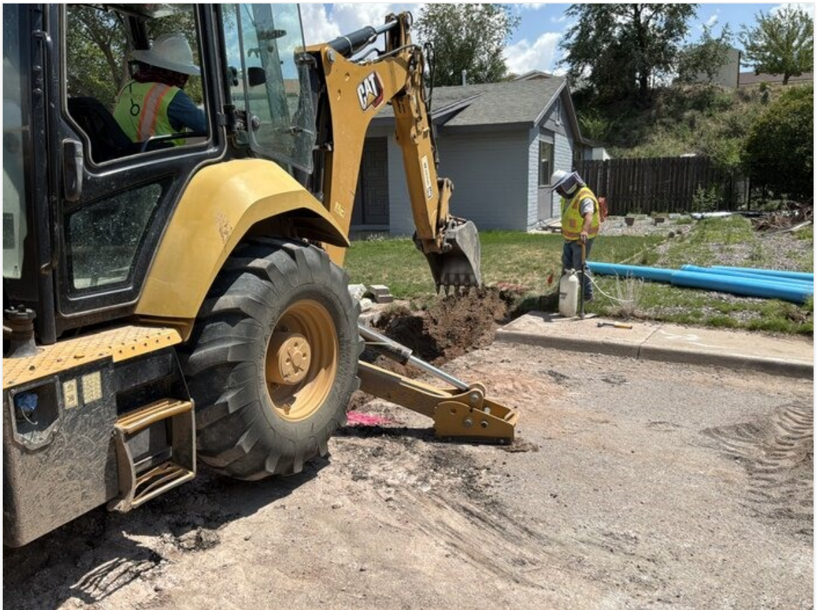
Excavation for hydrant #43 on Chalcocite St.
