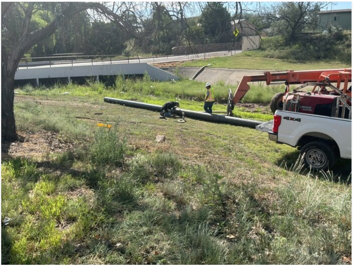
Welding of the 12" steel casing for arroyo crossing.
