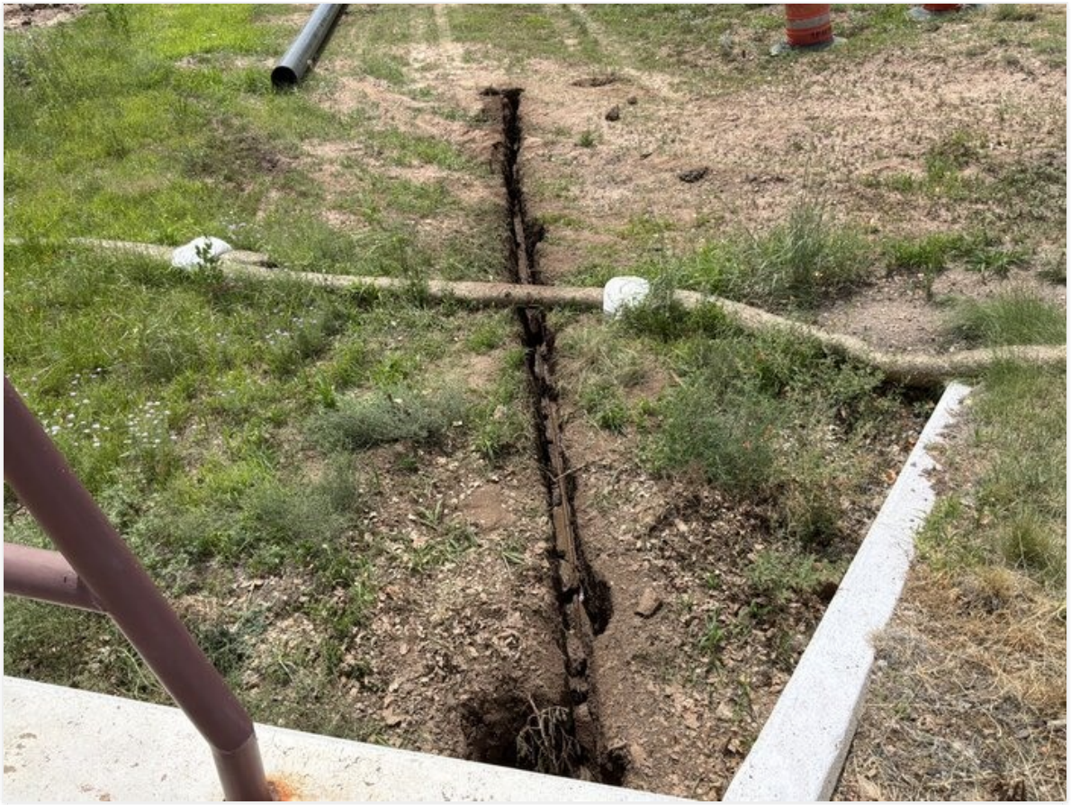
Located power line in arroyo.
