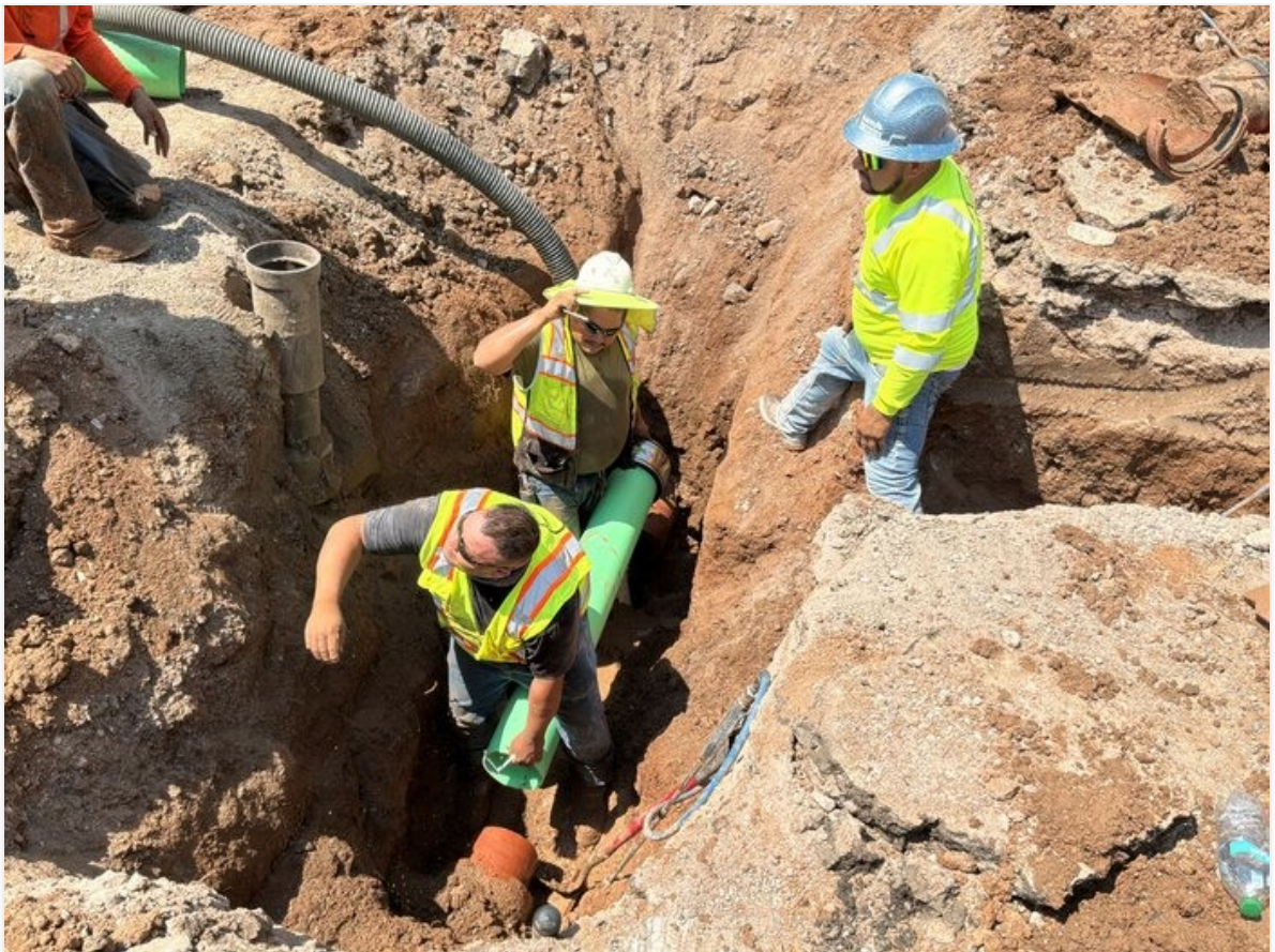
Repair for sewer at approx sta 29+17 Cuprite St.
