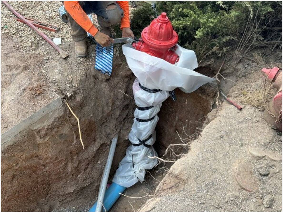
Installed hydrant #32. A riser will be needed to raise to grade.
