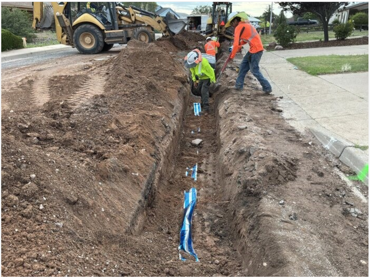
Caution tape being placed as per plan detail.
