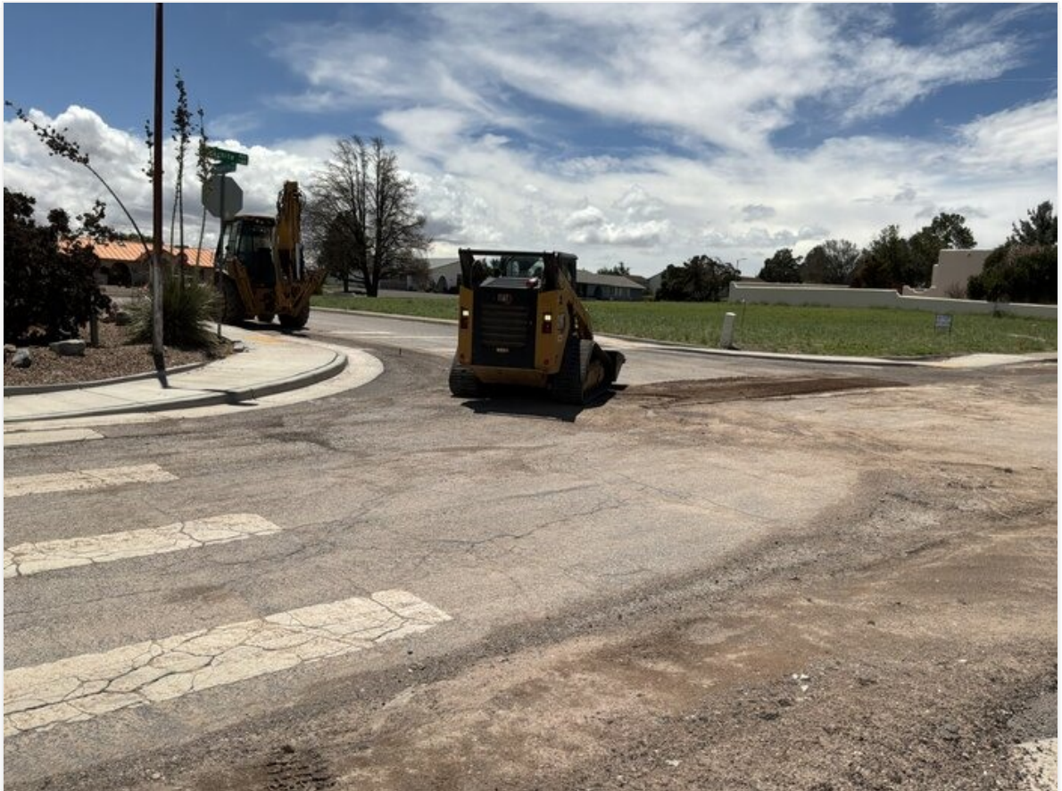
Maintaining intersections due to rain.
