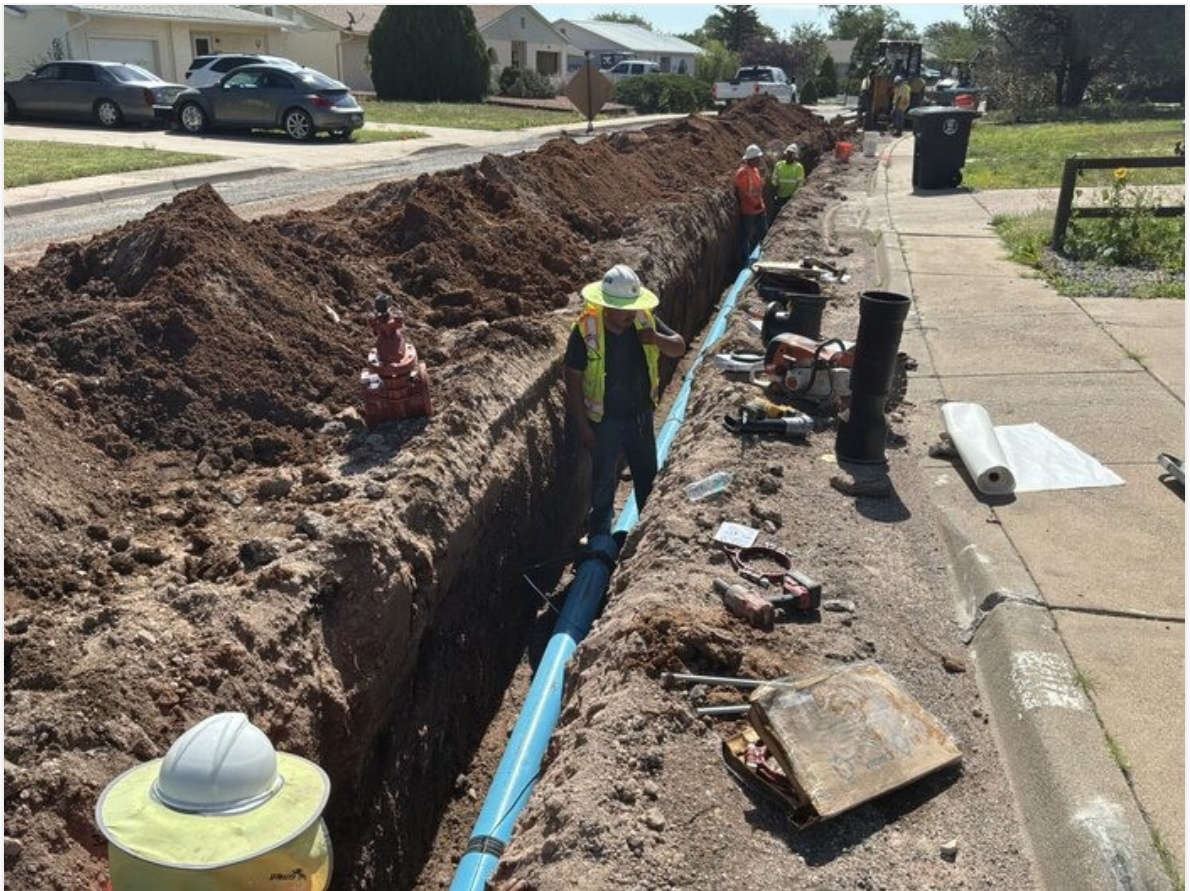
6" C-900 pipe laying operations on Chalcocite St.
