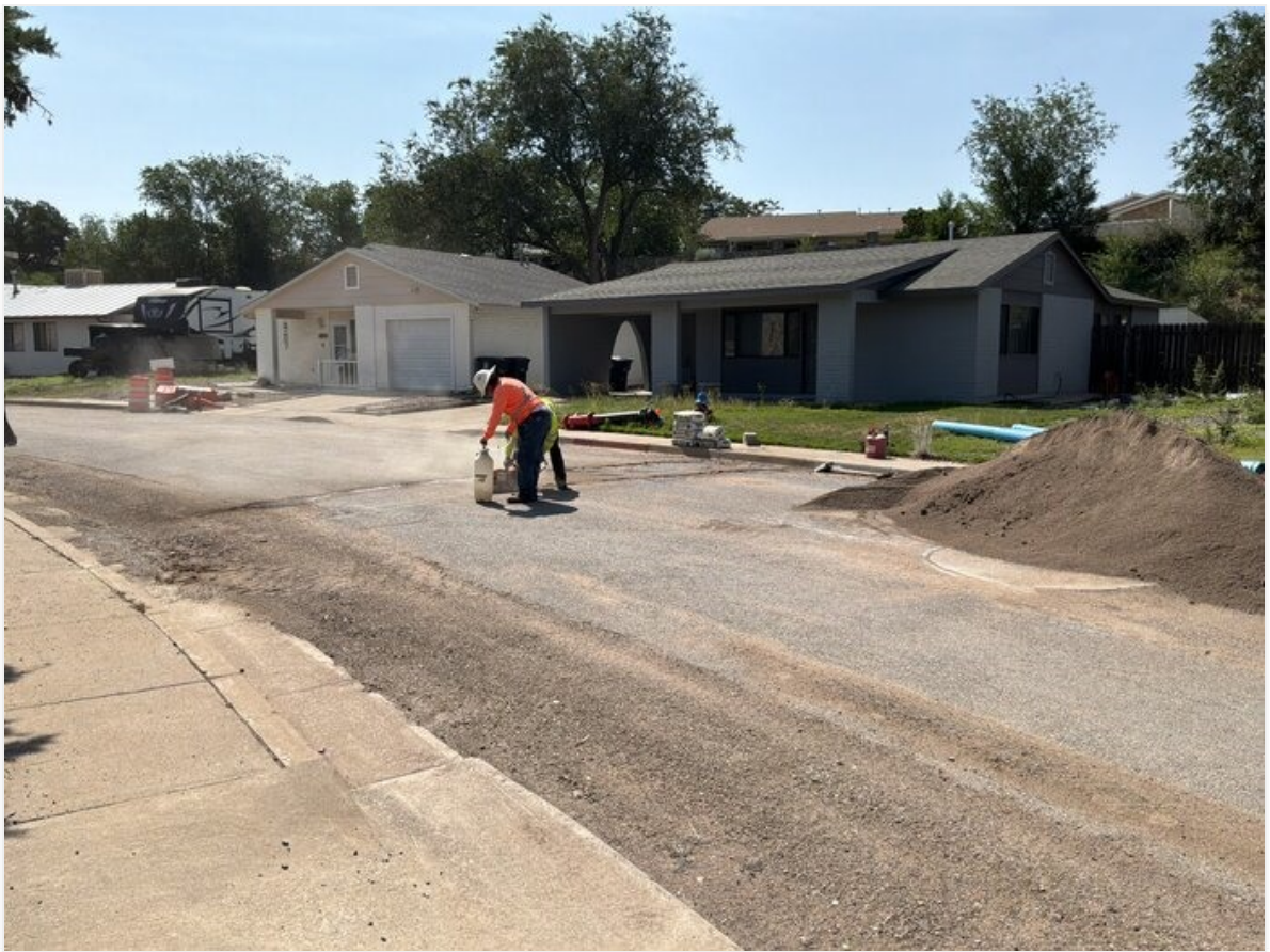
Saw cutting roadway for fire line on Chalcocite St. hydrant #43
