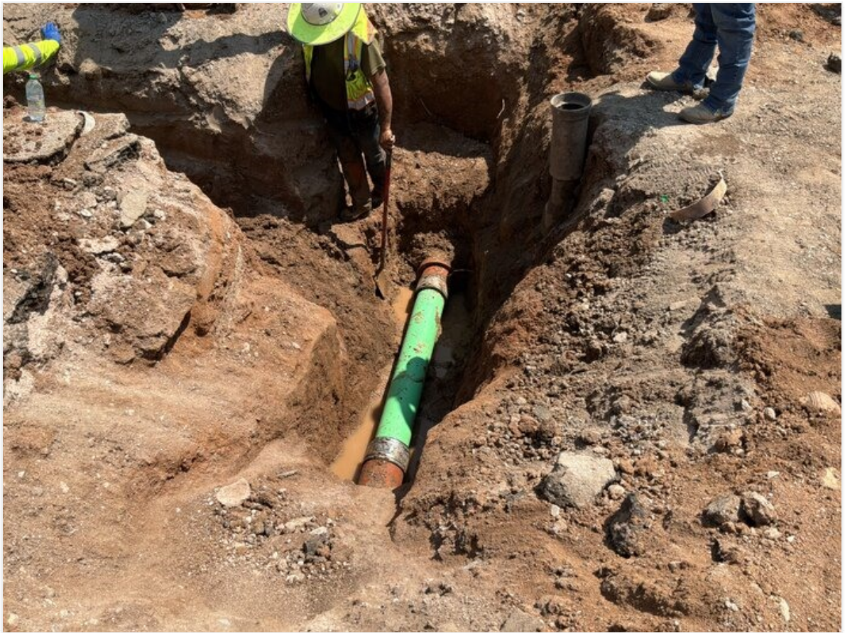
Repaired sewer line at approx. sta 29+17
