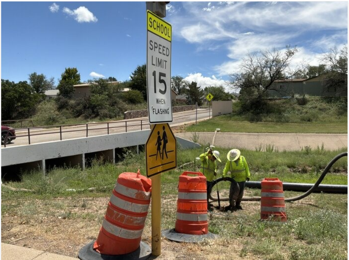
Potholing for power line in arroyo.
