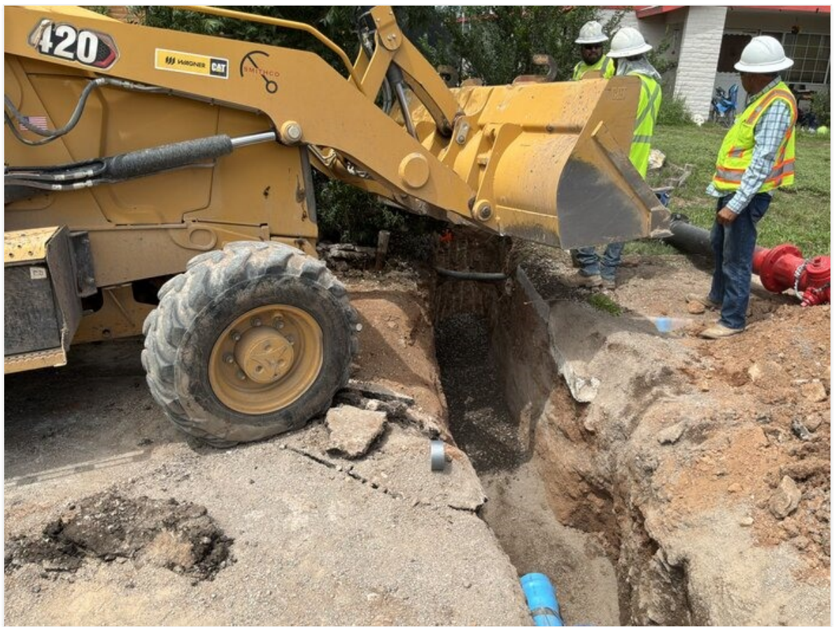
Placing gravel for hydrant weep hole.
