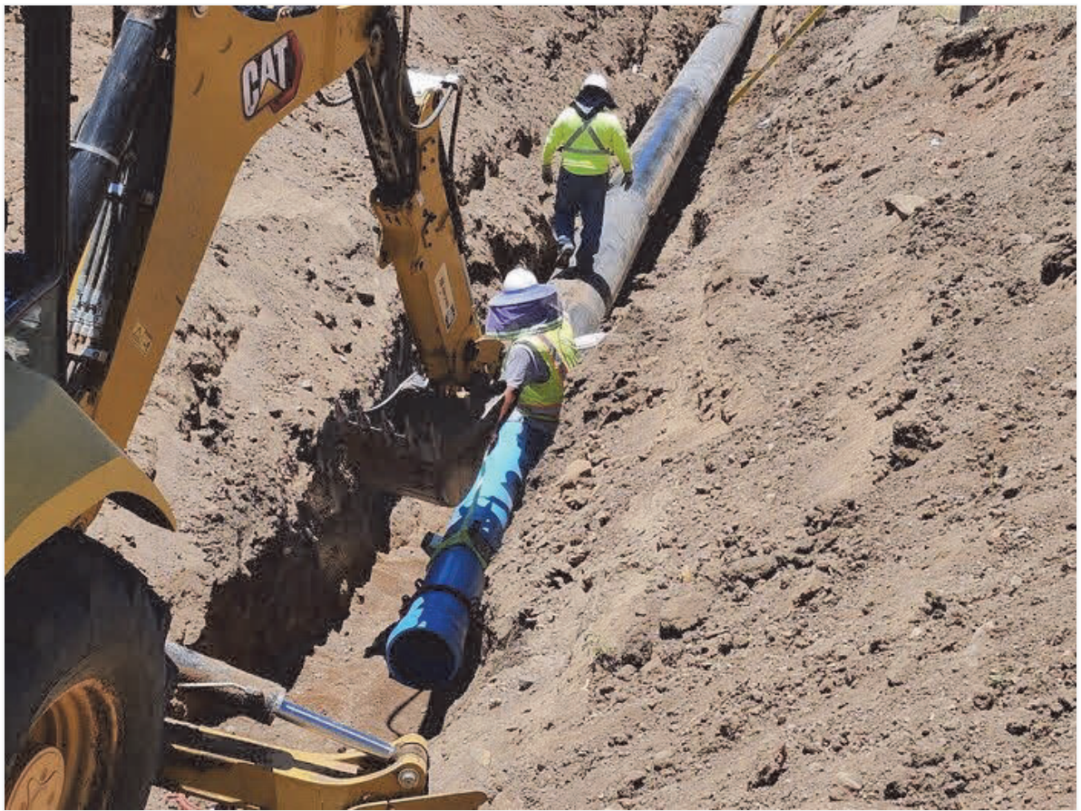
Pushing 12" C-900 into steel casing with pipe spacers.
