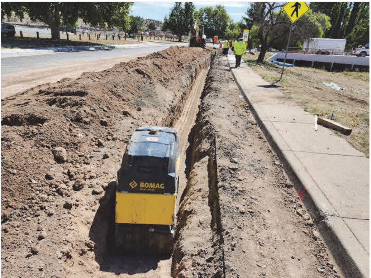
Trench roller backfill on 12" C-900 on Copper Dr.
