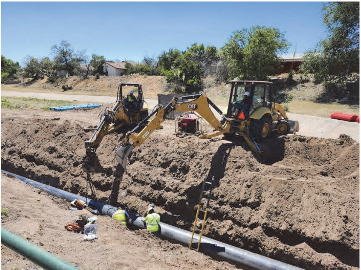
Placing the 24" steel casing in Copper Dr arroyo.
