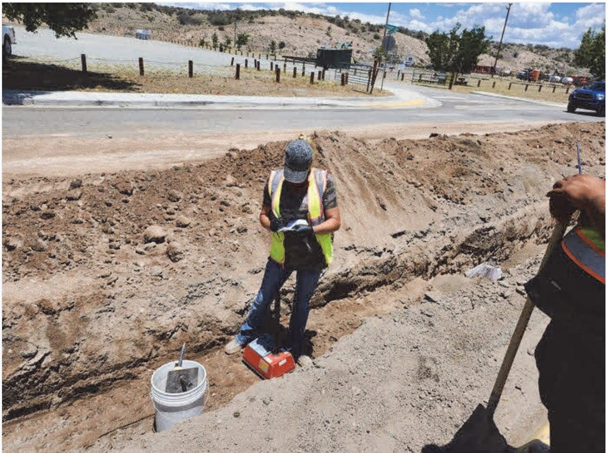
Summit testing tech, taking density on 12" C-900.
