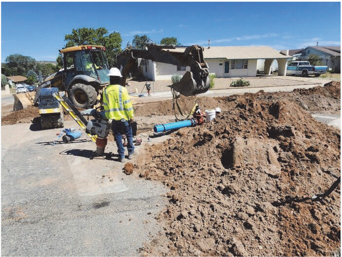
Crew #2 installing GV on Chalcocite St.
