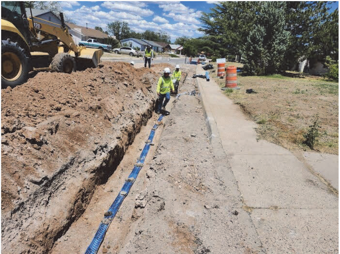
Caution tape placed as per plan over the 6" C-900 on Chalcocite St.
