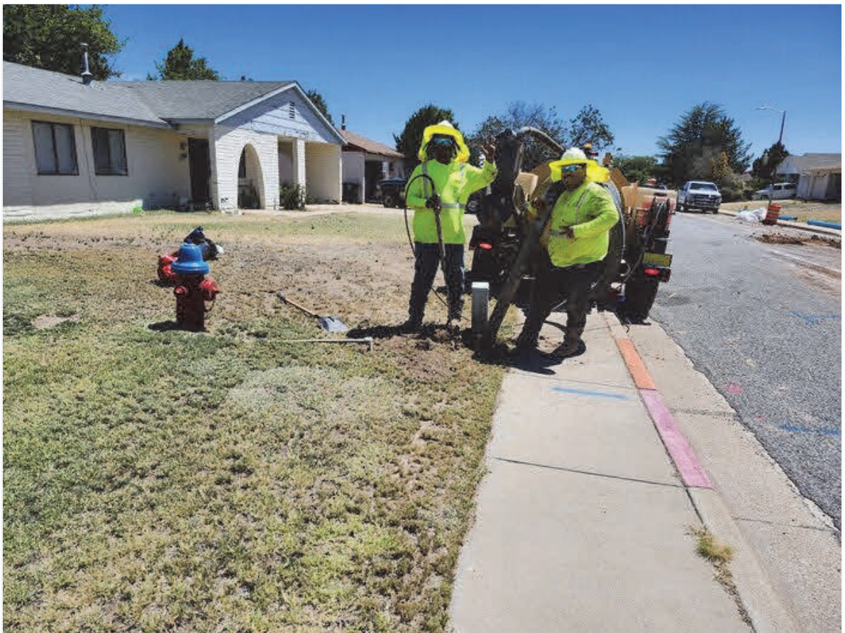
Potholing for hydrant placement on Chalcocite St.
