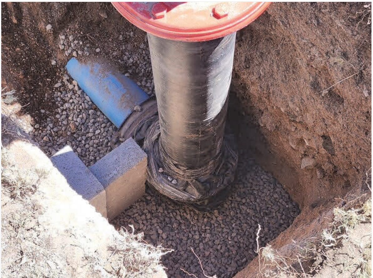
18" of gravel placed under hydrant foot.
