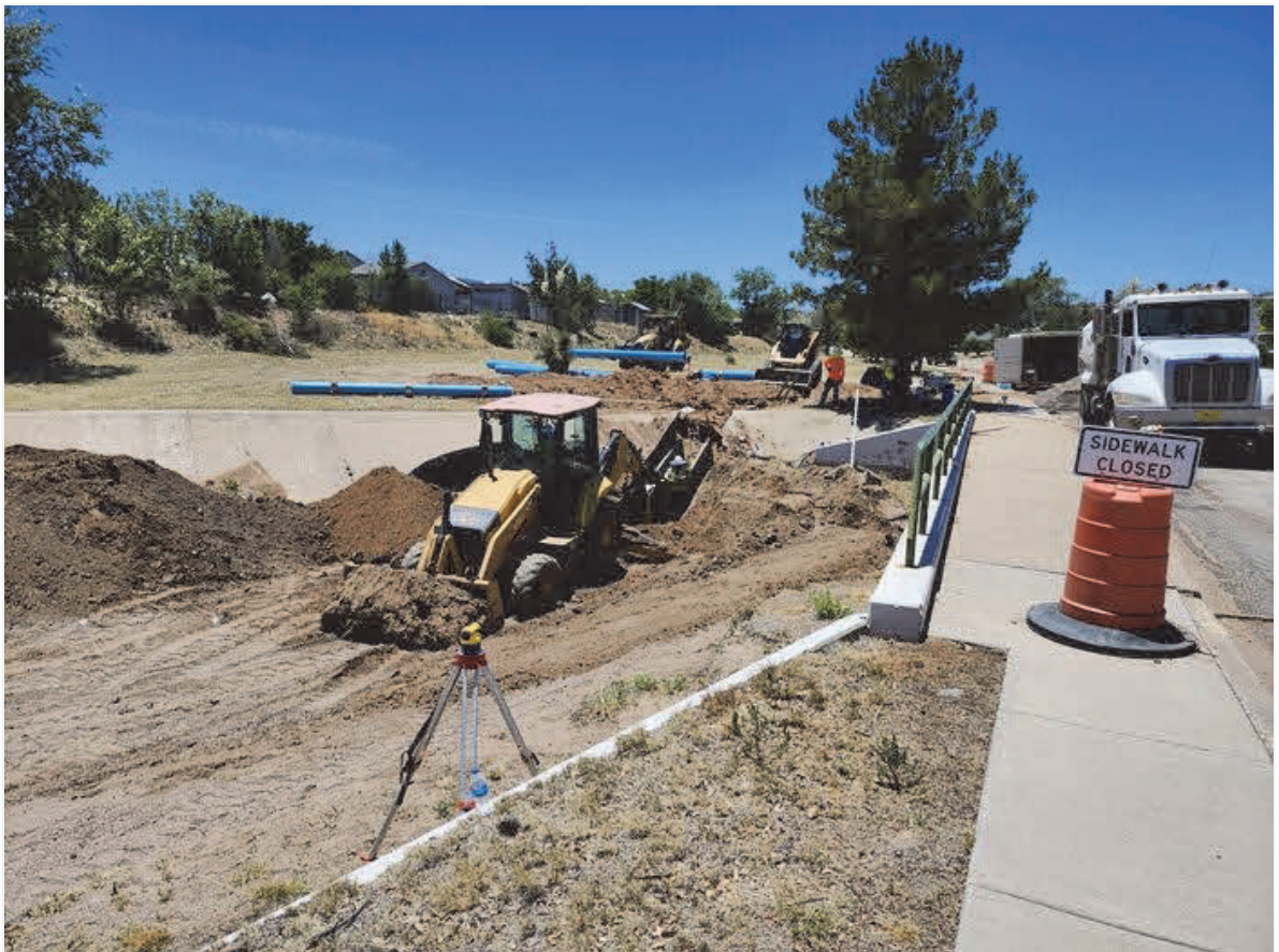
Excavation for 12" C-900 at arroyo crossing.
