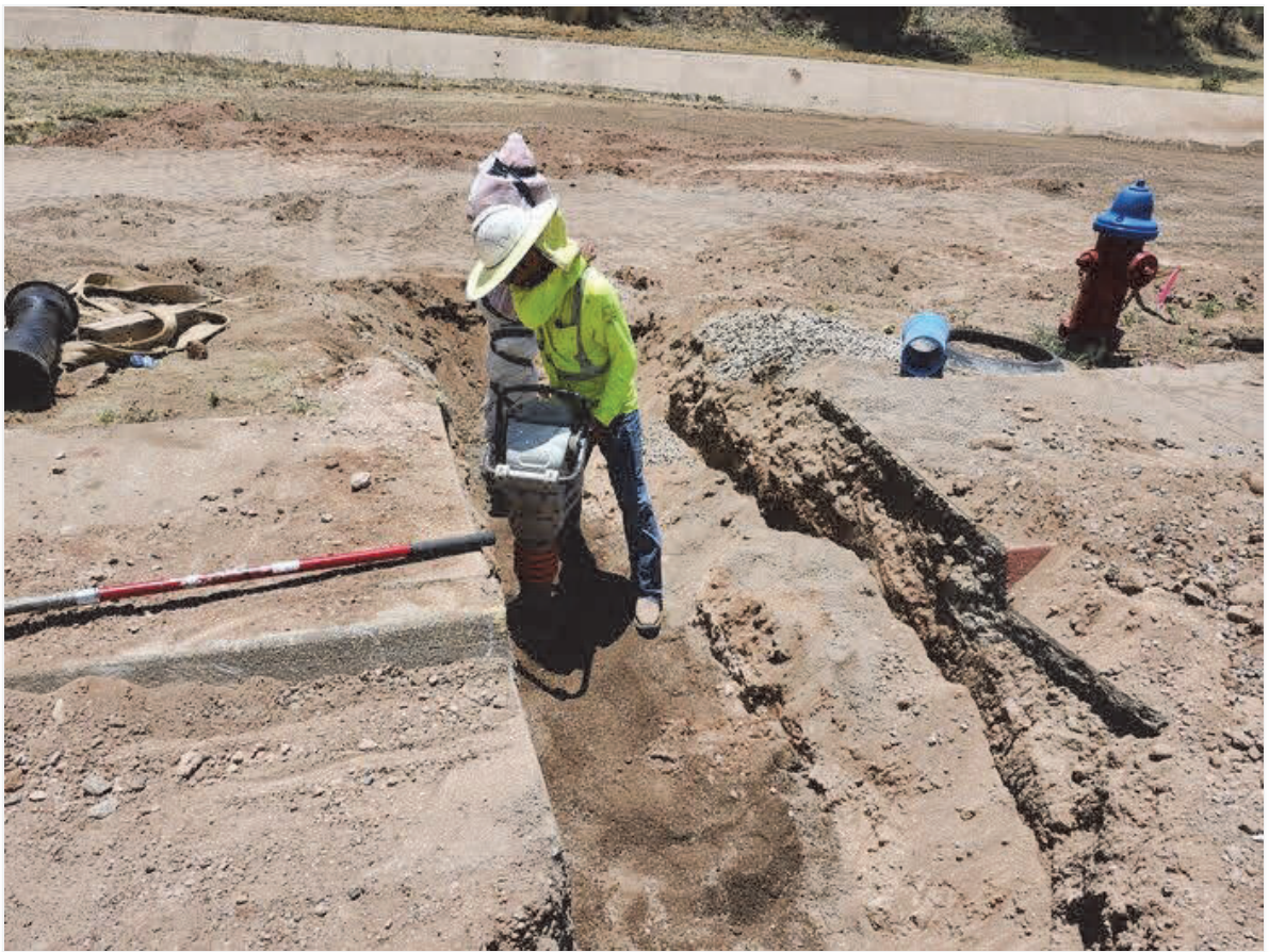
Compaction for 6" fire line on Copper Dr.
