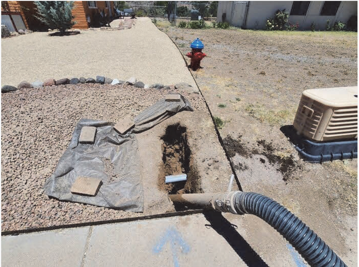
Potholing for hydrant placement on Chalcocite St.
