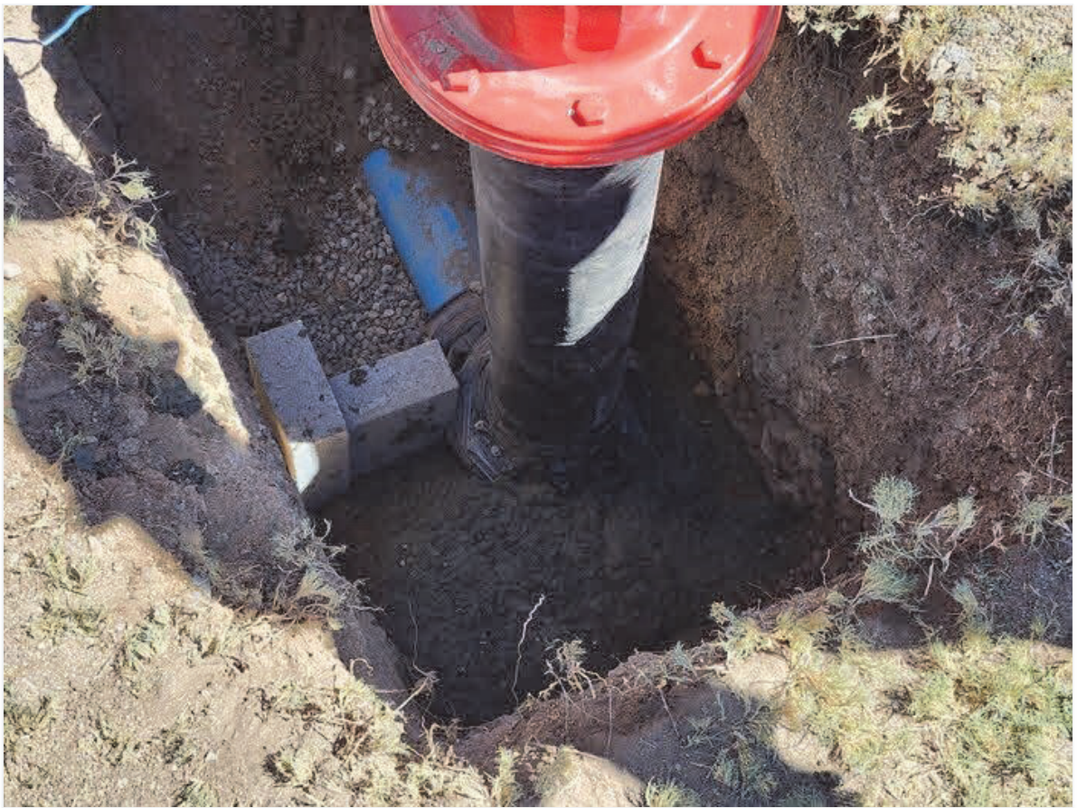
2'x2' 3000psi concrete thrust block placed behind hydrant #40 on Chalcocite St.
