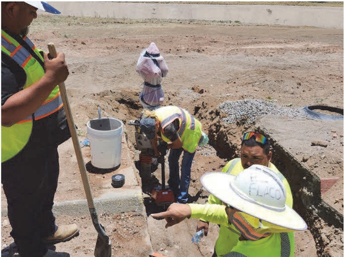
6" C-900 fire line hydrant #7 backfill density.
