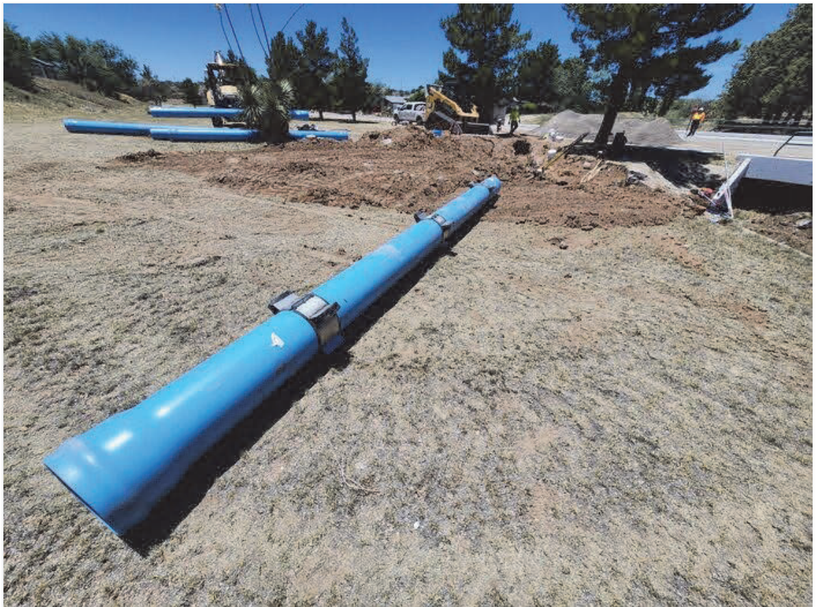
Spacers for 24" steel casing on Copper Dr. arroyo.
