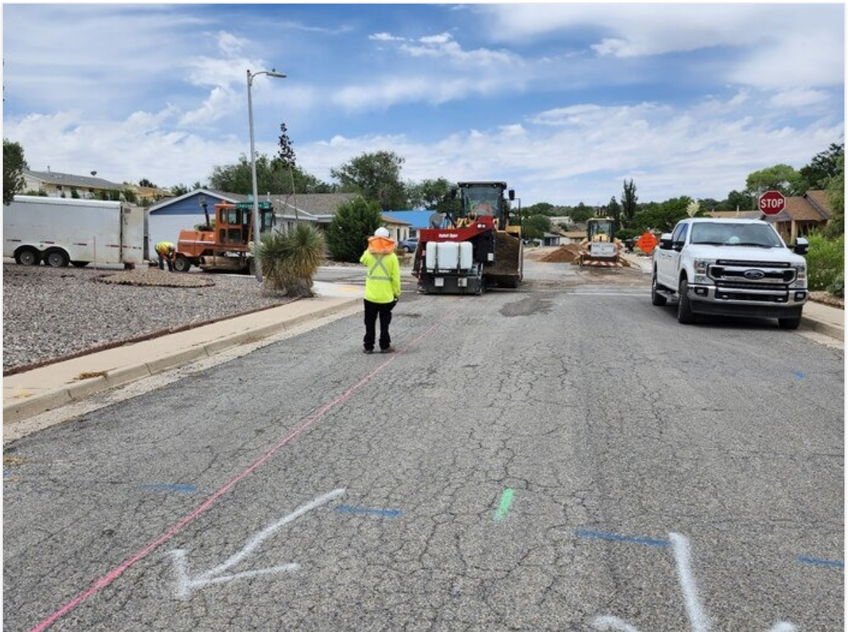
Milling Chalcocite 6" C-900 pipe alignment.
