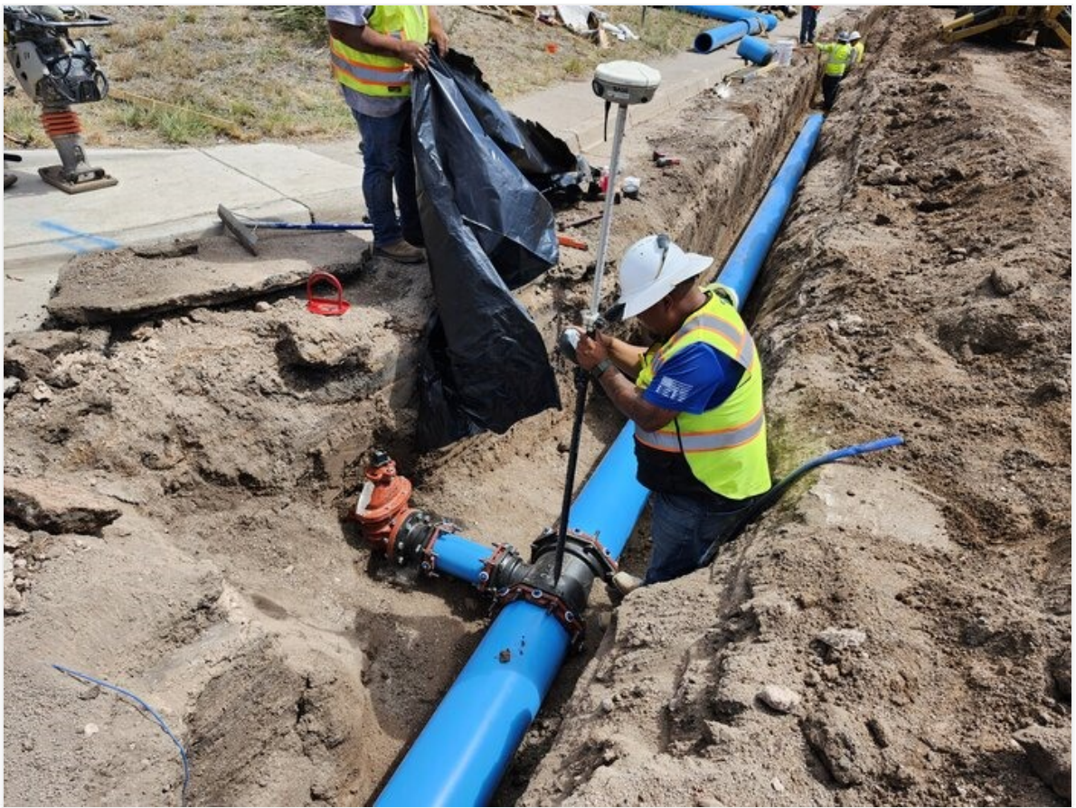
As-Built survey shots being taken on 12" DI fittings on Copper Dr.
