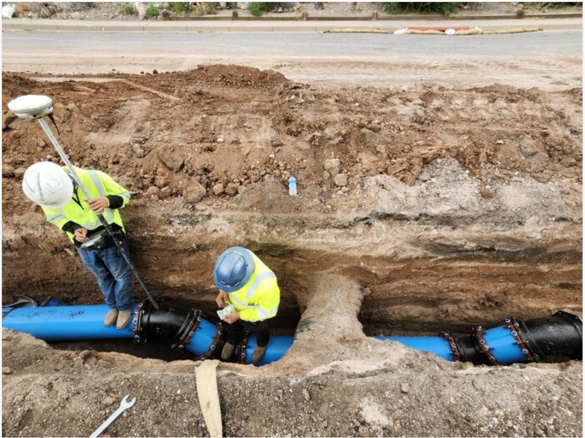
As-built survey on DI 45 bends on Copper Dr.
