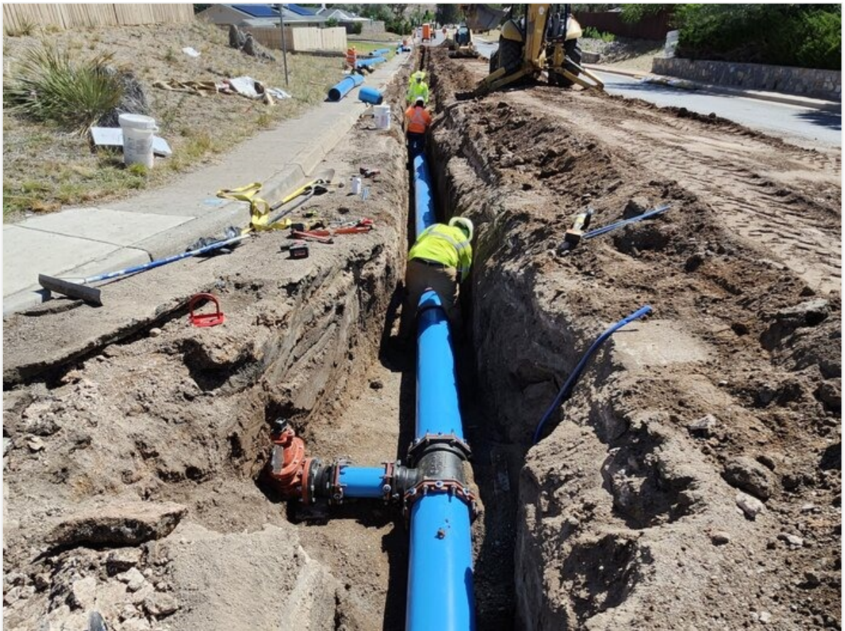
DI fittings being installed on Copper Dr. for the 12" C-900
