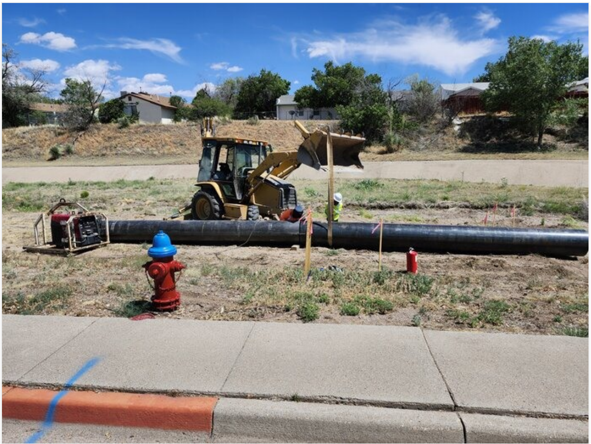
Welding of 24" steel casing for 12" C-900 on Copper Dr.
