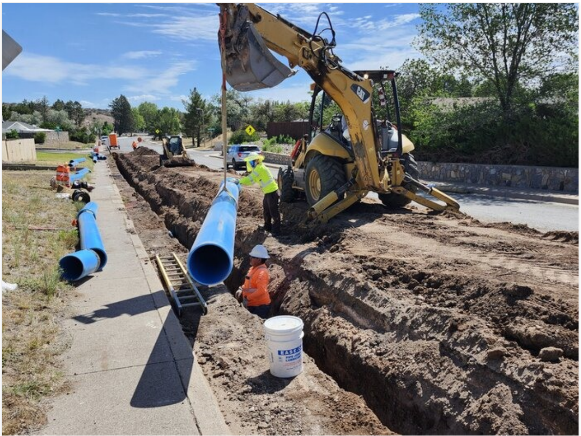
12" C-900 being placed on Copper Dr.
