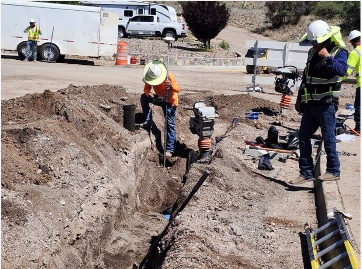
As-Built survey being taken on 6" fitting on Chalcocite St.
