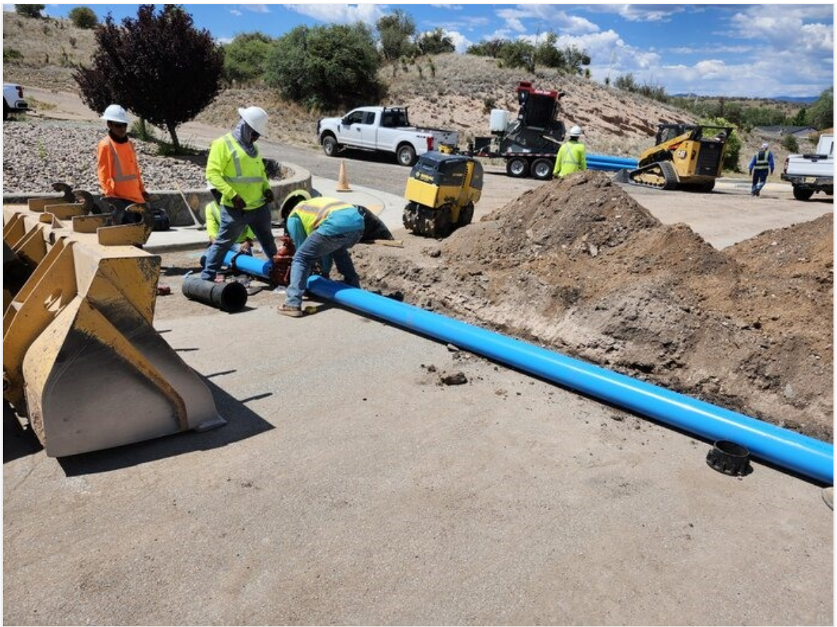
Crew #2 attaching fittings outside trench for connection to 12x6 tee on Copper Dr.
