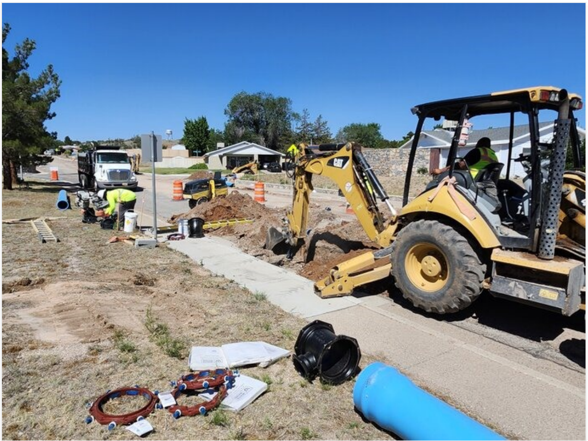
Crew #1 south side of Copper Dr excavation.
