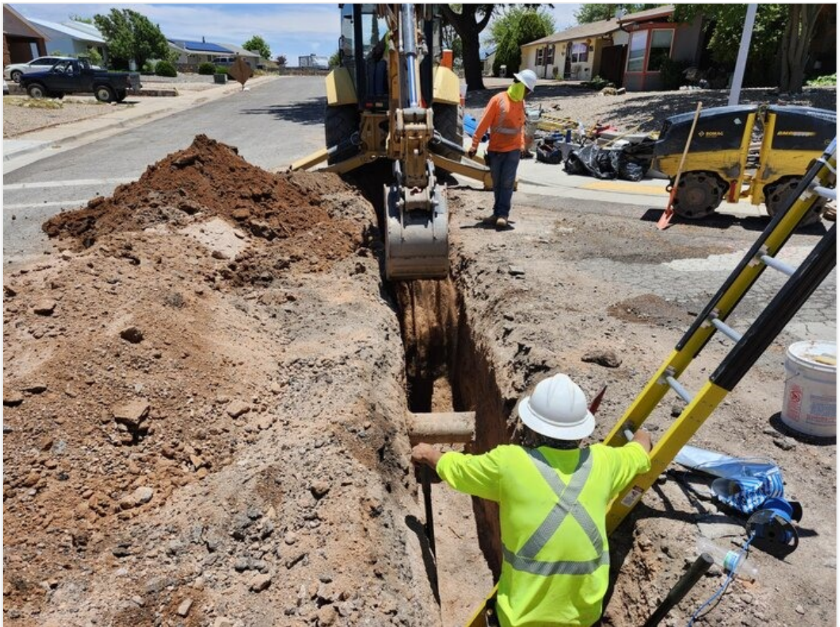
Exposing existing water line on Cuprite St. Crew #2 will use DI 45s to go under.
