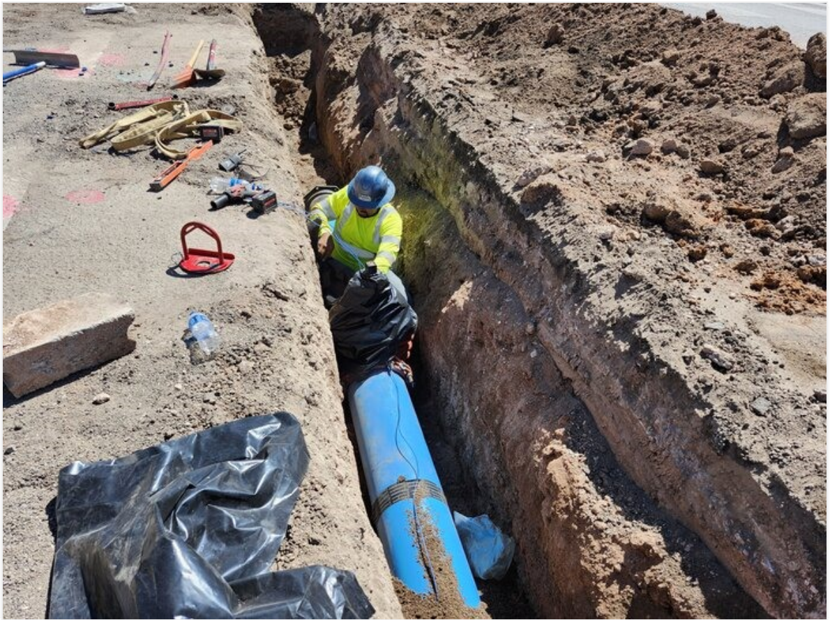
Wrapping anticorrosion plastic around 12" fittings on Copper Dr.
