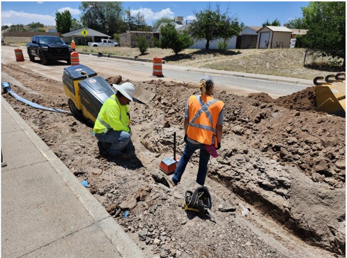
Summit testing backfill over 6" C-900 on Chalcocite St.
