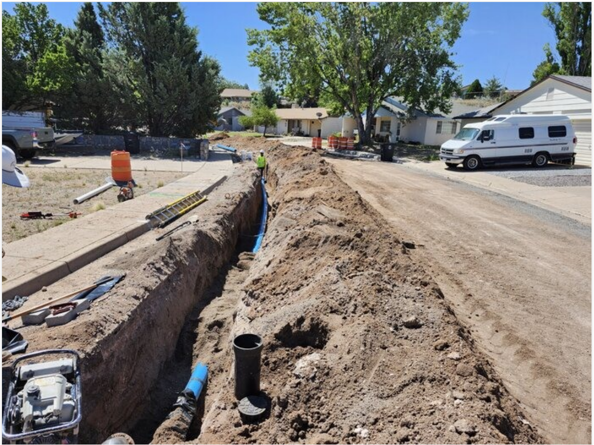
6" C-900 placement on Chalcocite St.
