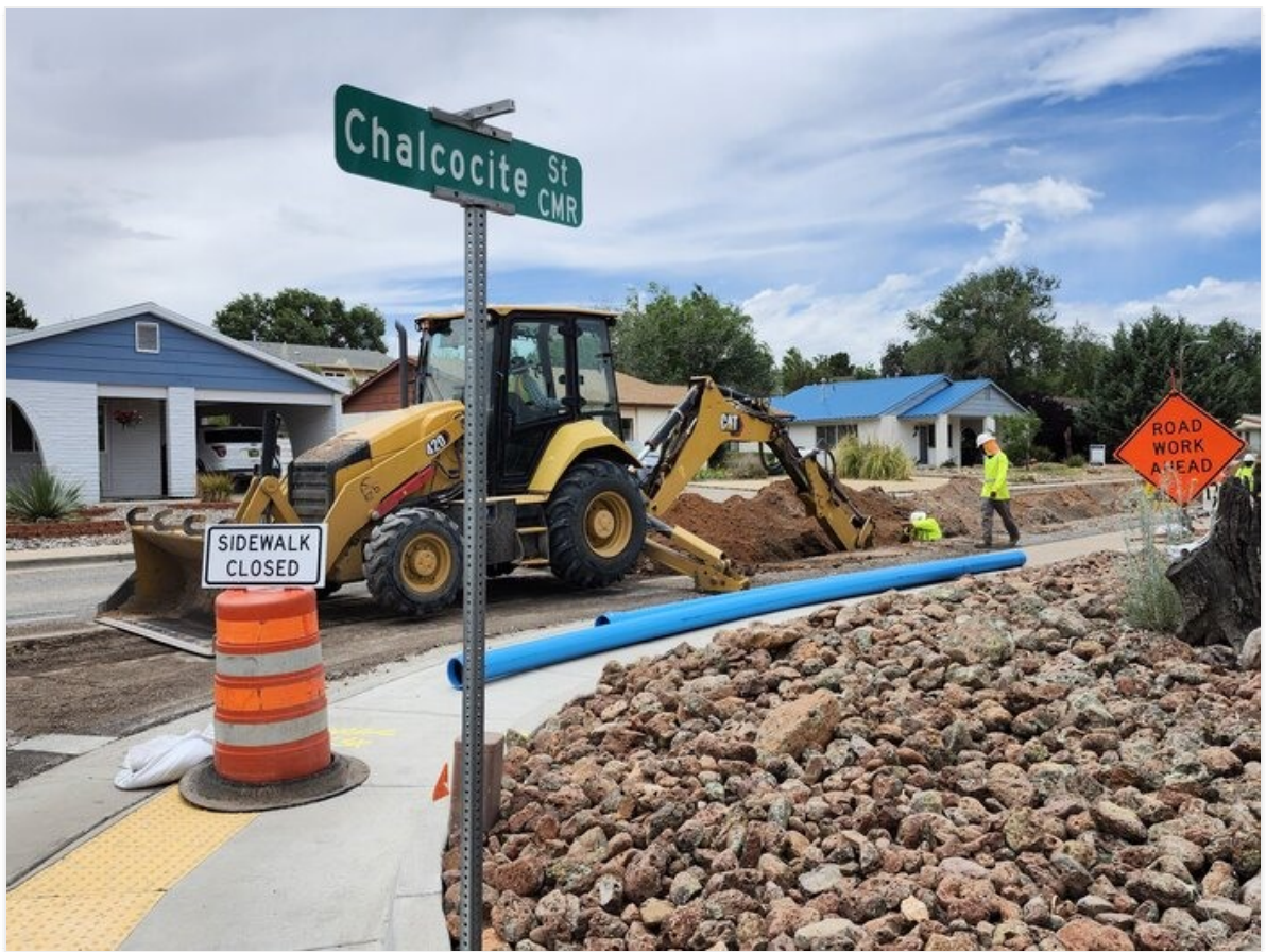
6" C-900 pipe operations.
