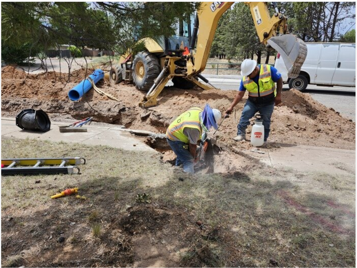
Saw cutting sidewalk on Copper Dr at sta. 42+85.
